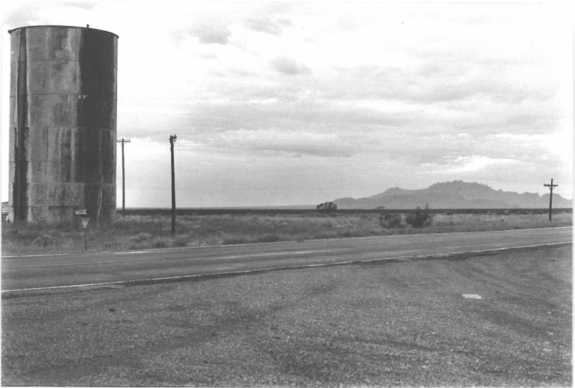
Figure 6. The Florida dump (looking south).
