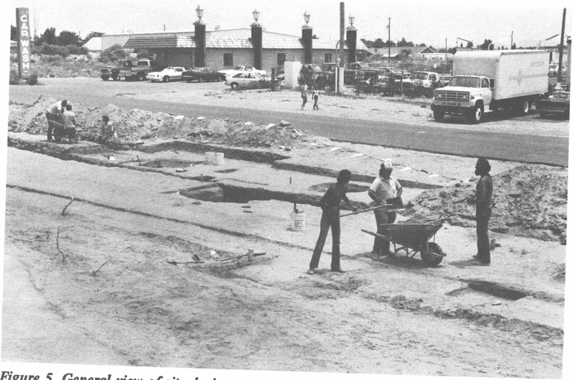
Figure 5. General view of site during excavation.
