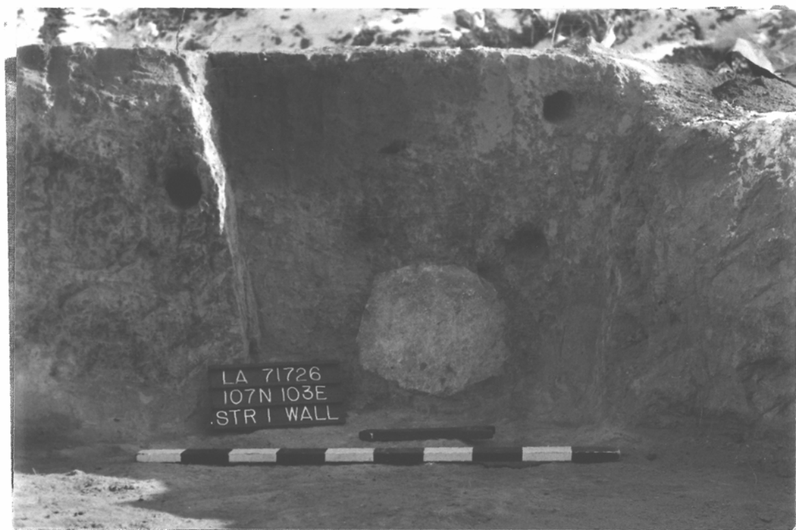
Figure 8. Ventilator, with damper slab in place.
