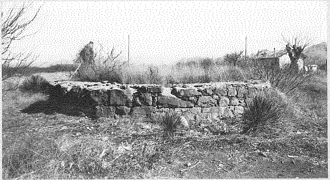
Figure 7. Rock base for water tank, LA 67962.
