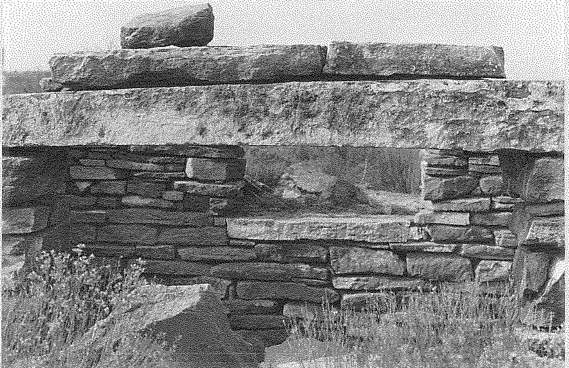
Figure 8. Window of dugout with stone lintel and sill; facing west.
