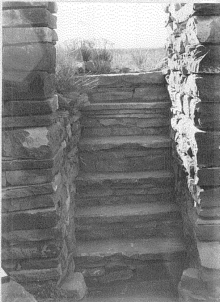
Figure 9. Stone steps leading into dugout; facing south. Note stone sills at base of stairs possibly for wood floor.
