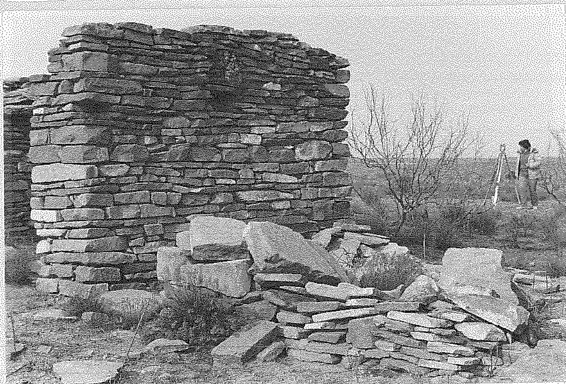
Figure 14. Section B of rock outbuilding showing collapsed walls; facing northwest.
