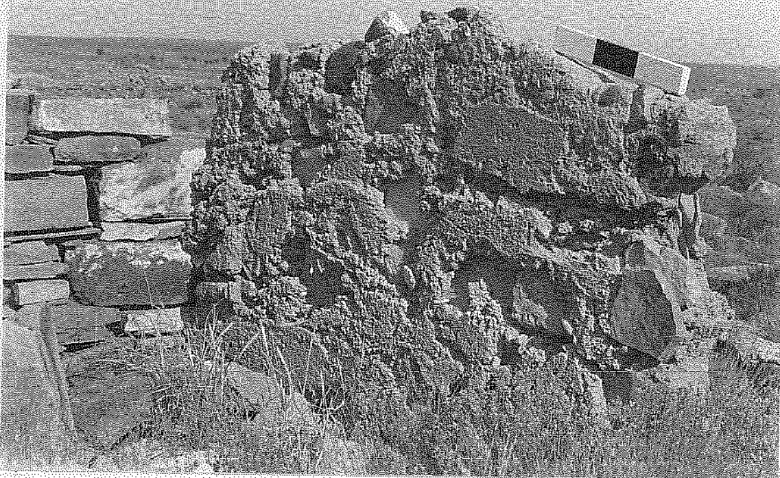
Figure 11. Sandstone and concrete wall of addition to dugout; facing northeast.
