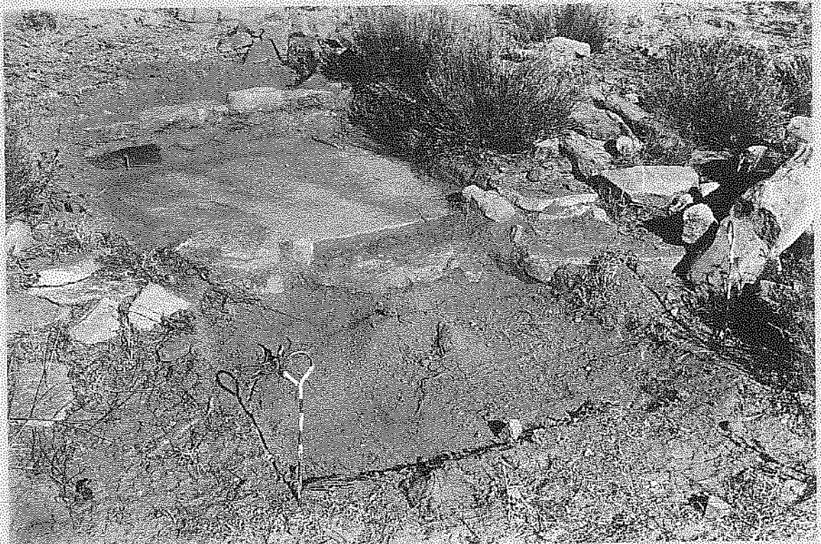
Figure 15. Concrete slab foundation; facing north.
