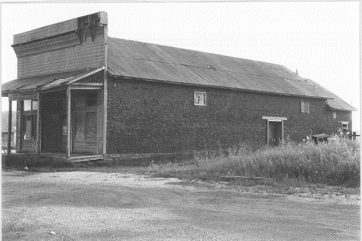
Figure 13. The former Weil Store, built in 1906, located on the southwest corner of the intersection of NM 120 and 422, Ocate, New Mexico. This store was purchased and run by the Strong family after WW II. In 1960, Donaciano Mondragon bought and operated it. It has been closed since 1974. (Photo by Linda J. Goodman, August 1991)
