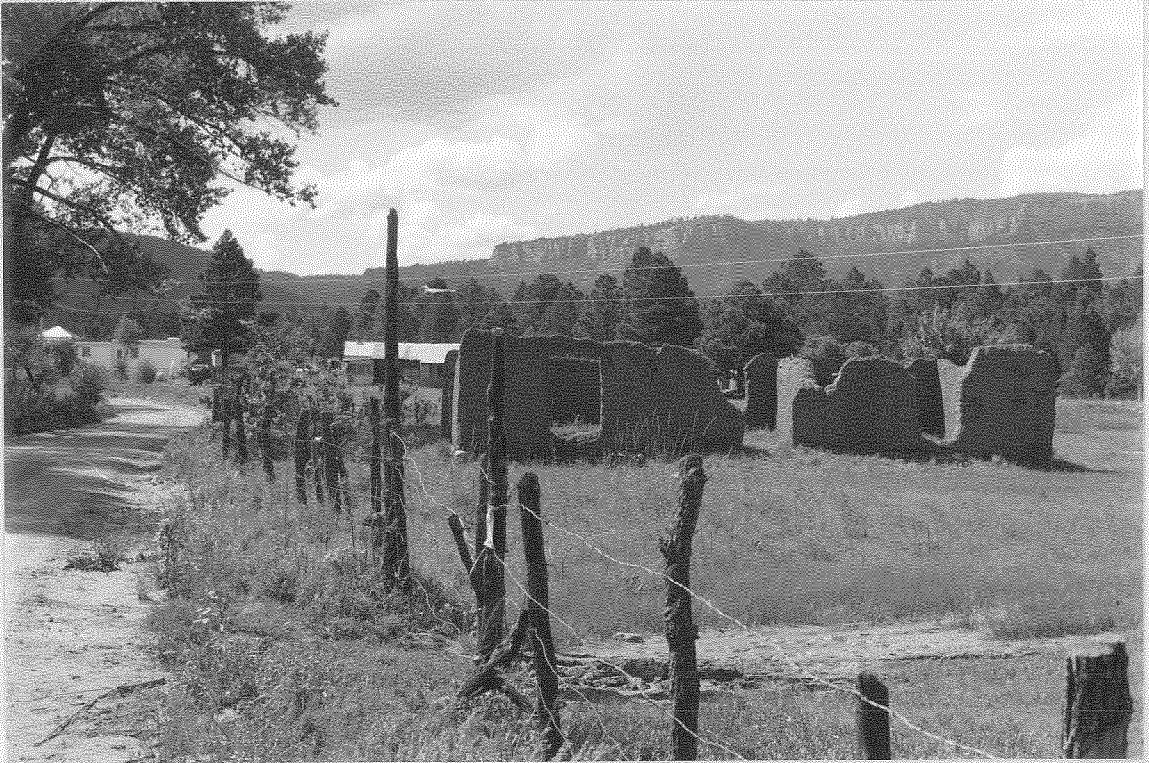
Figure 12. Ruin of Juan Le Febre's house in the village of Le Febre, northwest of Ocate. (Photo by Linda J. Goodman, August 1991)
