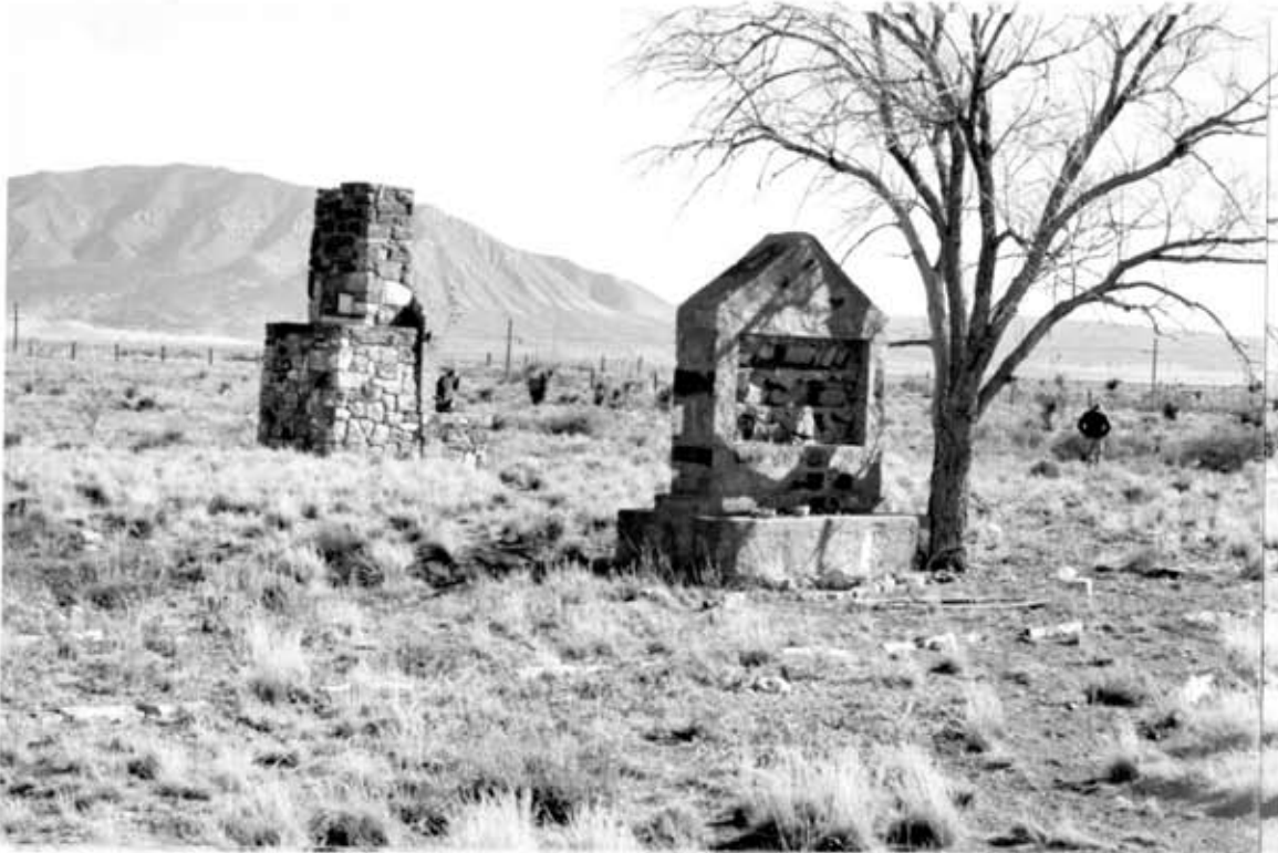
Figure 3. Recreation hall fireplace and masonry bulletin board at the Carrizozo CCC camp, looking northeast.
