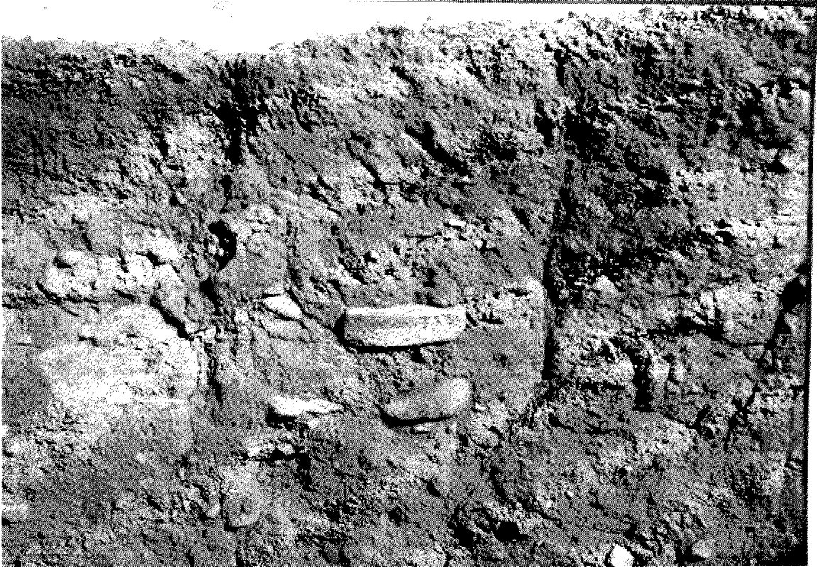
Figure 39. Detail of blocked doorway between Room 10 and Room 8.
