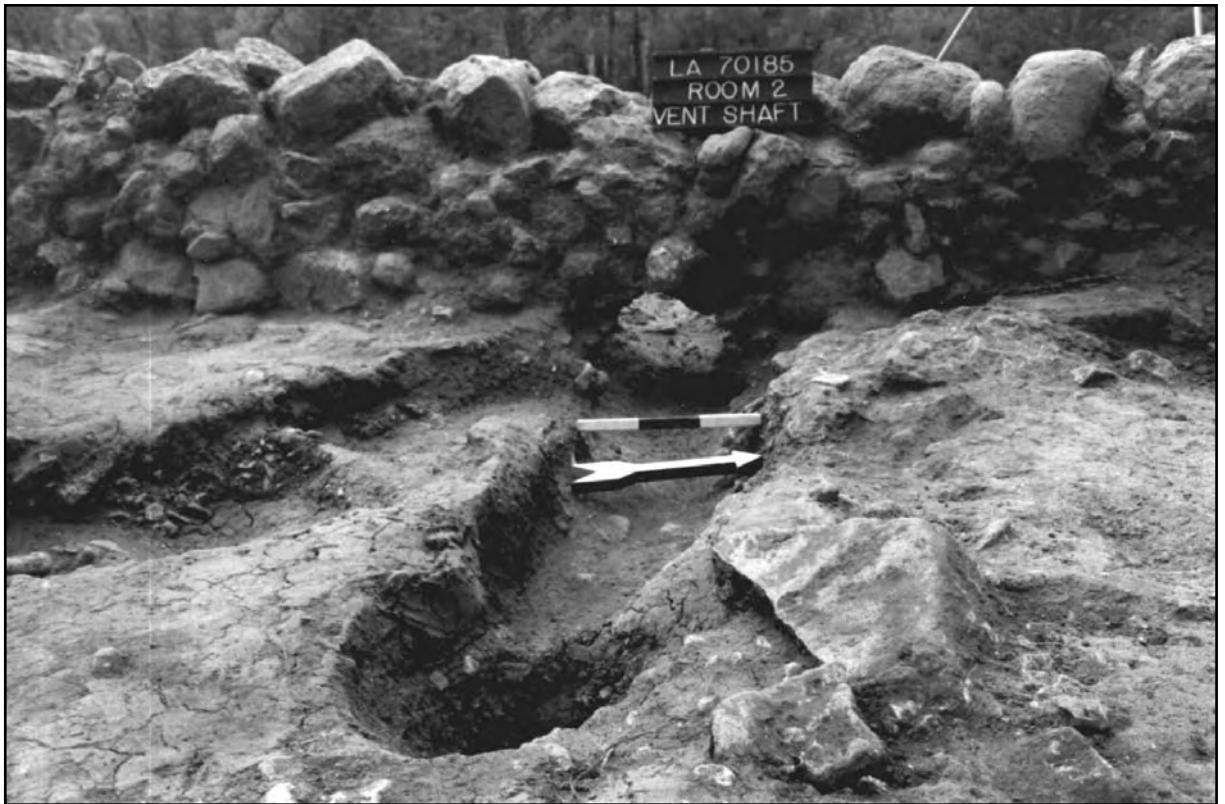
Figure 2.220. Vent shaft through the west wall. Sipapu east of the shaft. Pits 1 and 2 to the left.
