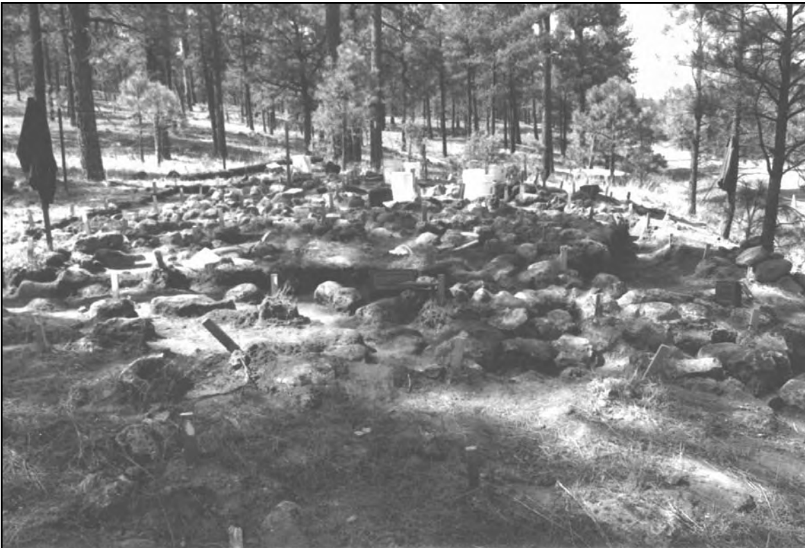
Figure 2.206. Surface stripping, facing south.
