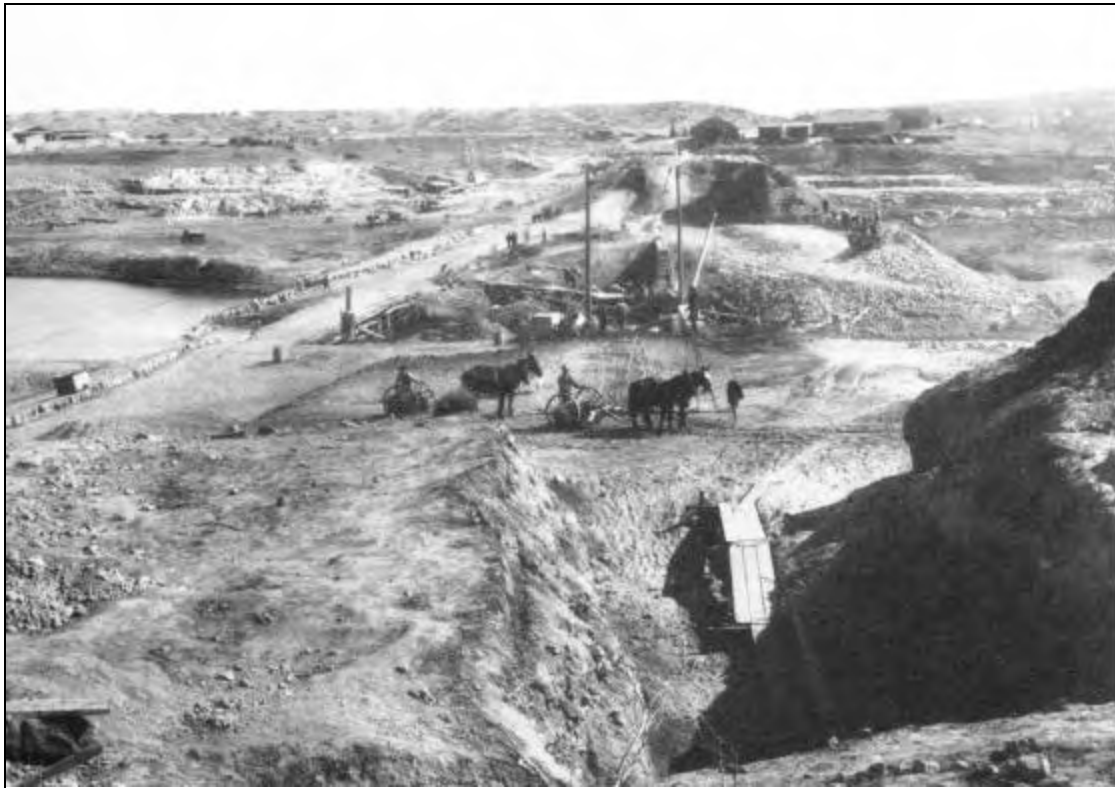
Figure 71. Construction of new rock-filled Avalon Dam, 1907. (From Watering the Land, courtesy National Park Service, Bureau of Reclamation, Denver)
