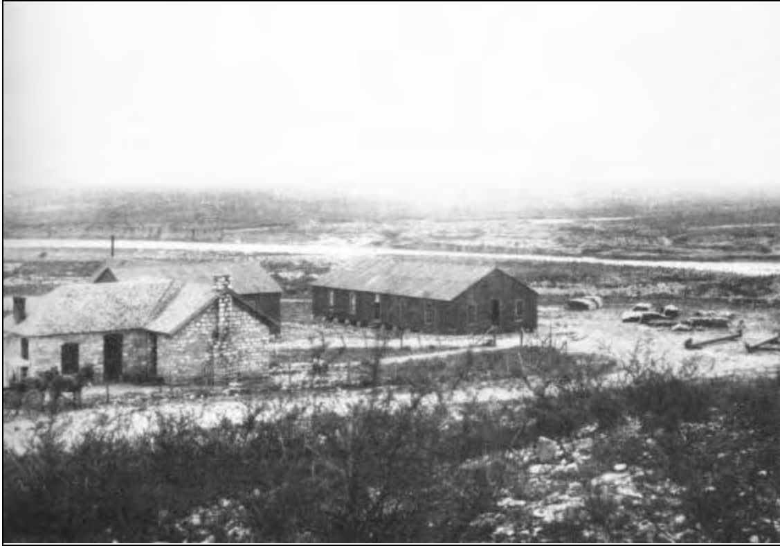
Figure 70. Reclamation repair crews' buildings and yard, Avalon Dam, 1906. (From Watering the Land, courtesy National Park Service, Bureau of Reclamation, Denver)
