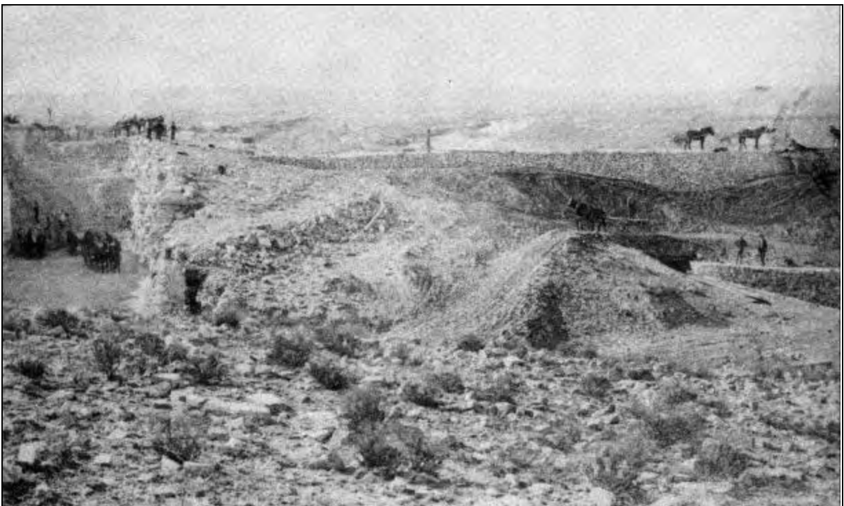
Figure 54. Avalon Dam under construction, 1889. (From Watering the Land, courtesy National Park Service, Bureau of Reclamation, Denver)
