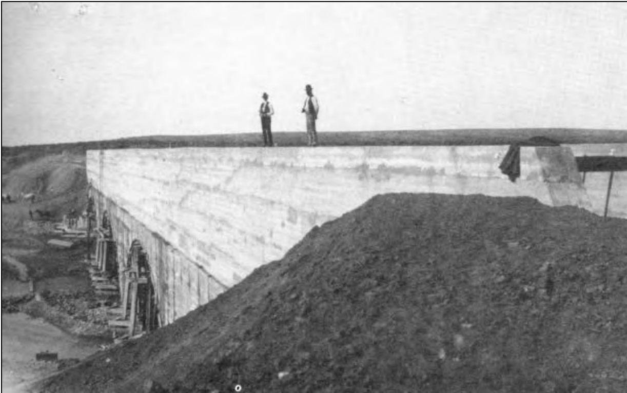
Figure 69. Concrete flume over Pecos River that replaced the wooden flume lost to flood waters. (From Watering the Land, courtesy National Park Service, Bureau of Reclamation, Denver)
