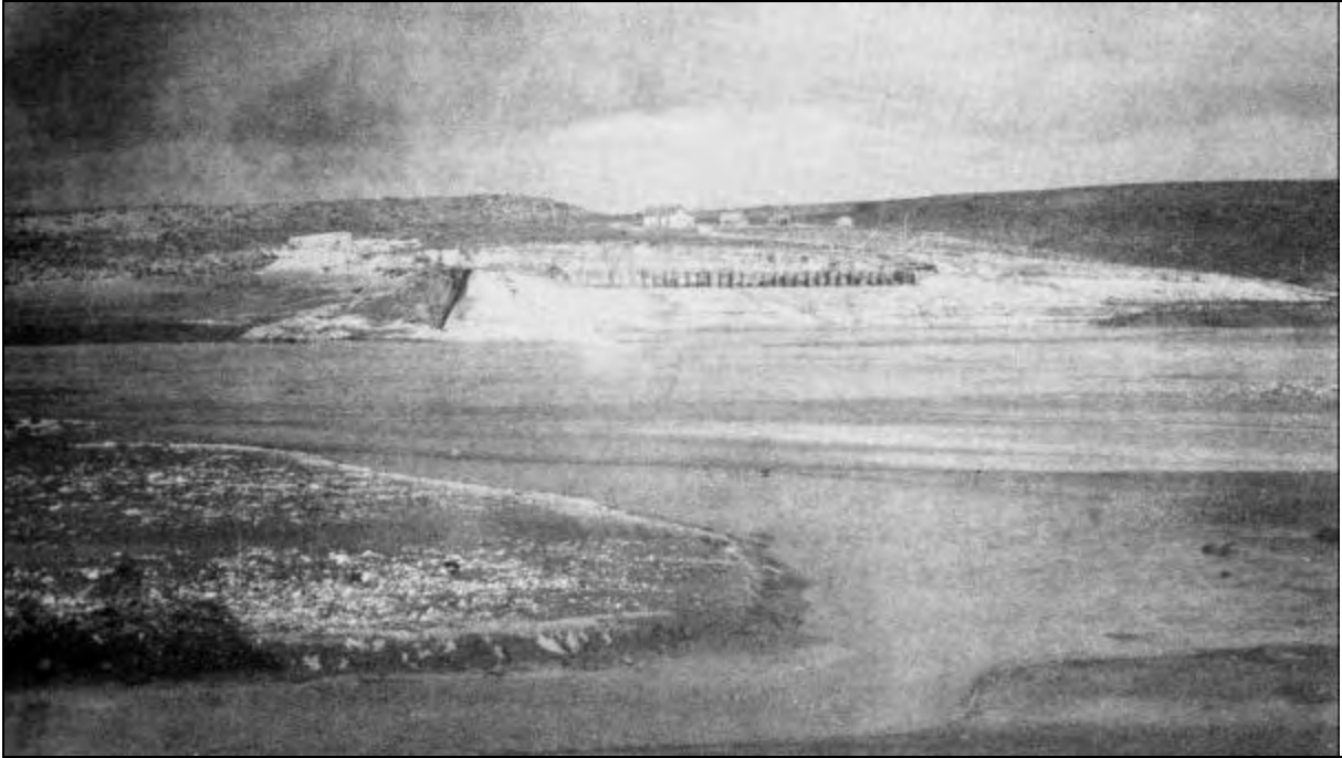
Figure 68. 1893 flood damage to Avalon Dam. (From Watering the Land, courtesy National Park Service, Bureau of Reclamation, Denver)
