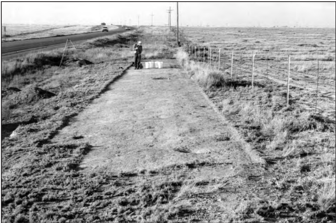
Figure 4. Surface stripping, LA 116467 (Site 7), looking south.
