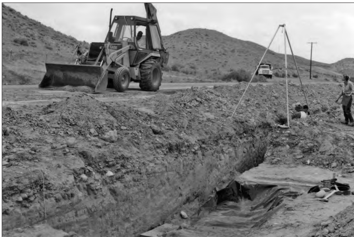
Figure 11.6. LA 60751, Backhoe Trench, north-south, between NM 170 and existing right-of-way fence.
