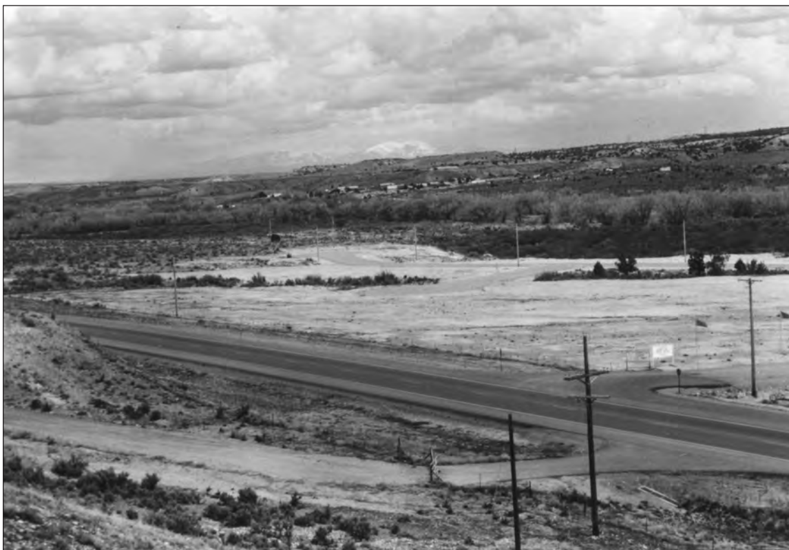
Figure 7.3. LA 60752, site area, post-excavation development overview, view northeast.
