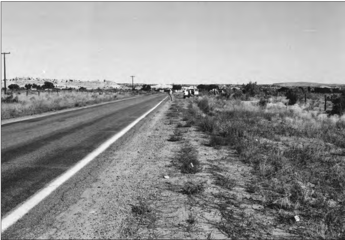
Figure 9.2. LA 60753, site overview, view north, pre-excavation.
