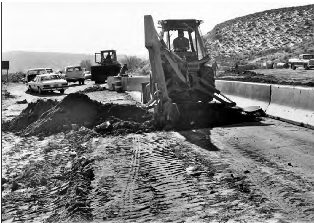
Figure 12.49. LA 37595, overview, Pit Structures 2, 3, and 4; northbound NM 170 pavement removal in progress.
