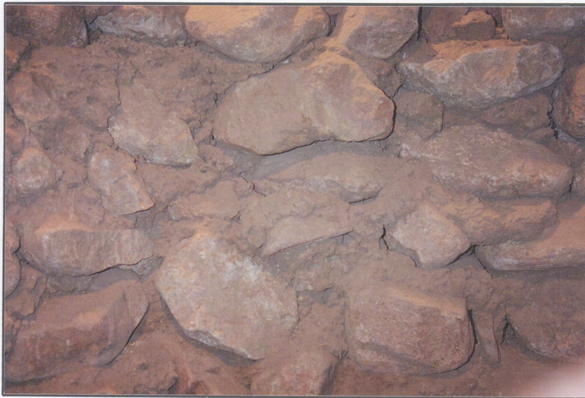
Figure 3. Stones and adobe mortar.
