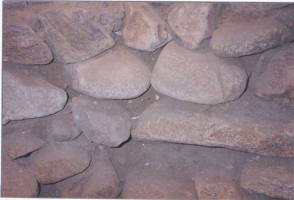
Figure 4. Stones below former water line, without mortar.
