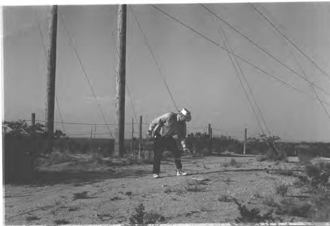
Figure 3. View of LA 113981, looking southwest.
