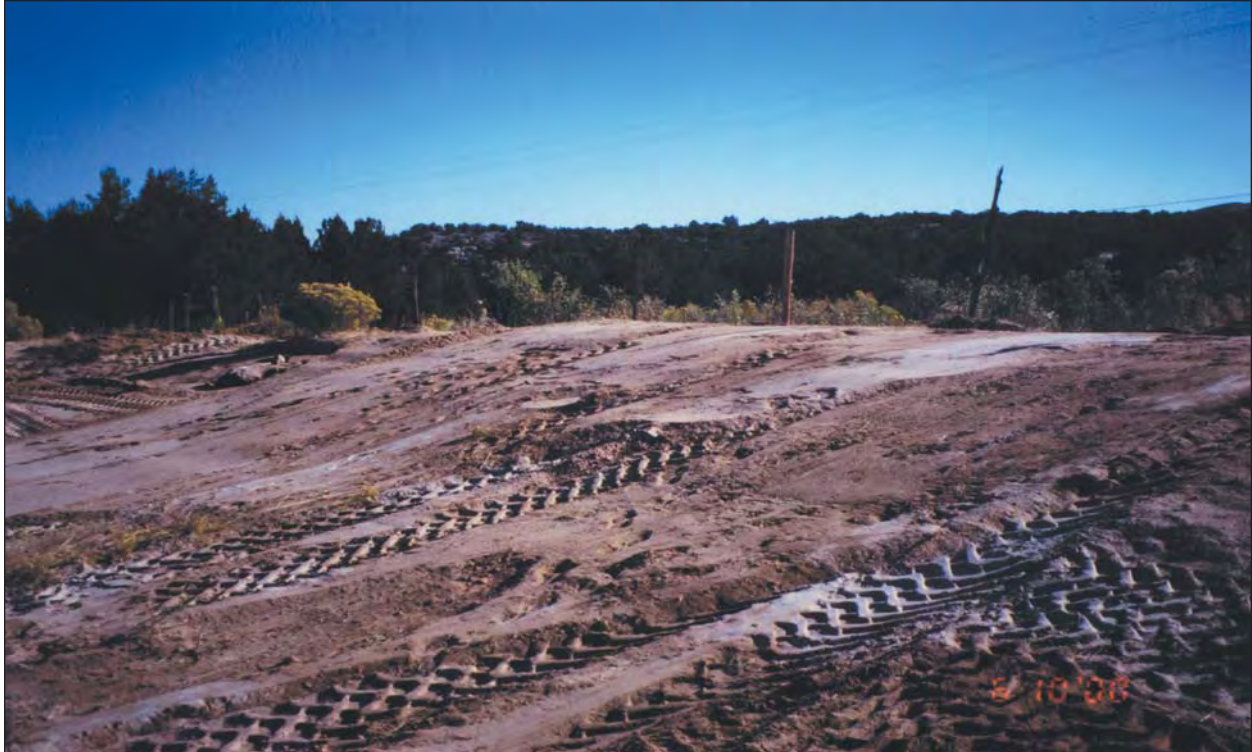
Figure 6. Roomblock in the process of being backfilled
