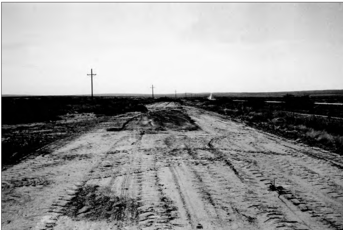
Figure 18. Mechanical stripping at LA 117248, looking south.
