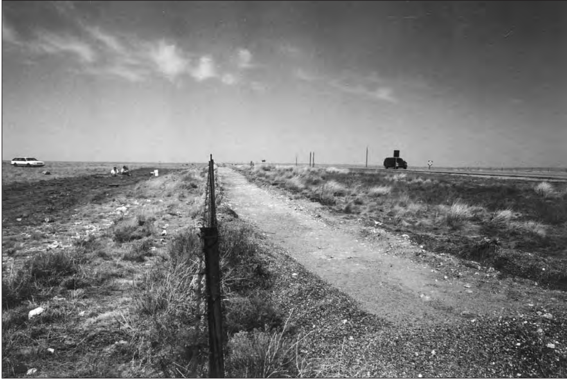
Figure 3. Mechanical scraping within the existing right-of-way at LA 117257, facing north.
