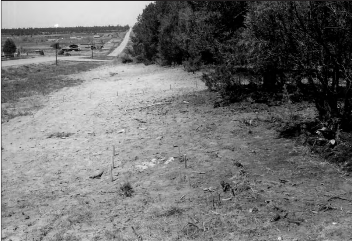
Figure 4. Bladed highway shoulder.
