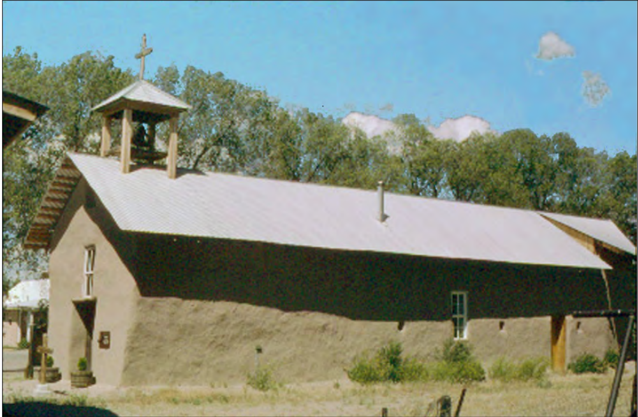
Figure 25.16. The Church of Santa Cruz, Ojo Caliente, originally built in 1793, refurbished in 1994, and photographed in 1998. Note the loop (gun) holes in the church wall just below the shadow. Photo by Linda J. Goodman.
