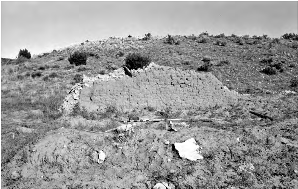
Figure 14.6. Standing portion of the east wall of Structure 1, LA 105710.
