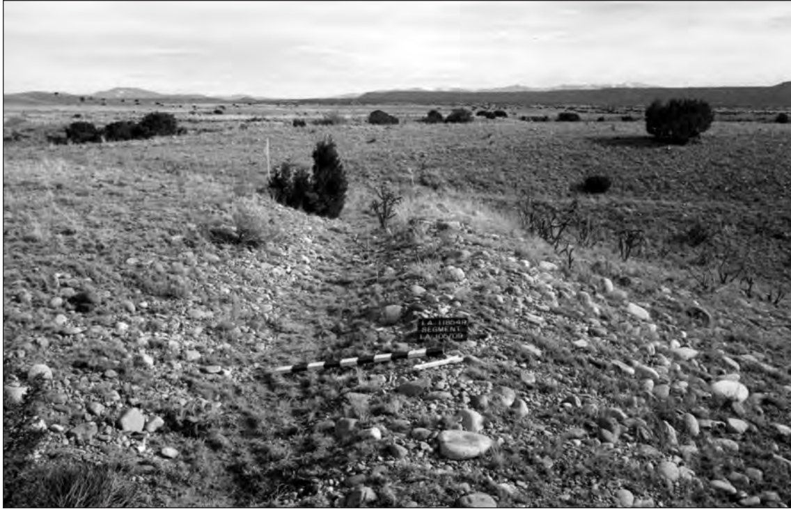
Figure 17.9. South end of segment of LA 118549 adjacent to LA 105709, showing how it followed the contours up to the top of the terrace. Note the distinct berm on the downslope side and the swalelike cross section.
