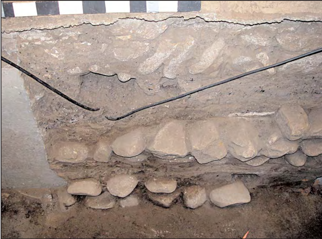
Figure 5. Feature 19, early Spanish Colonial foundations (lower) and Feature 19, middle Spanish Colonial foundation (middle), and 1867 foundation (upper).
