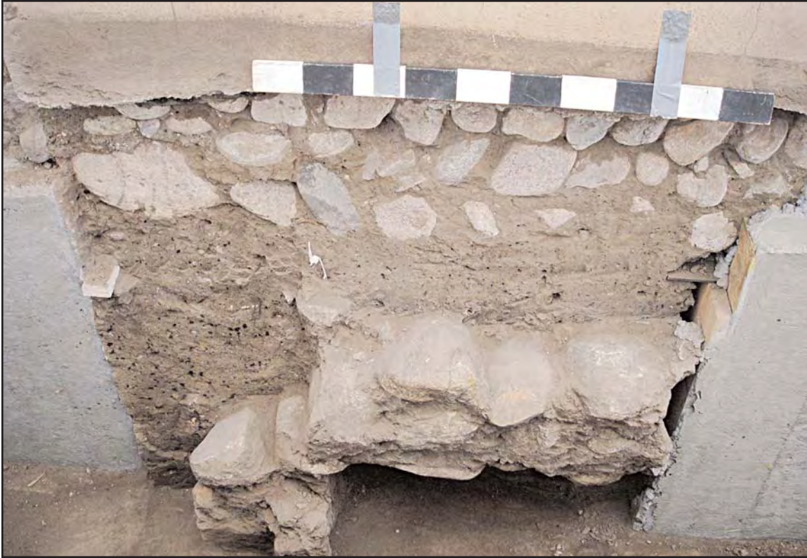
Figure 9. Feature 7, middle Spanish Colonial foundation and 1867 foundation.
