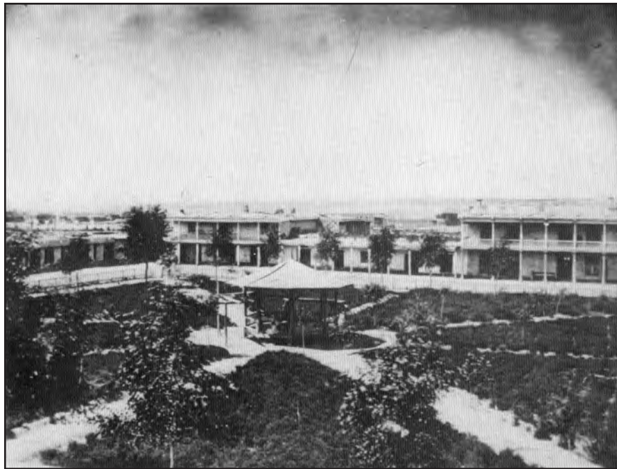
Figure 5. The gazebo being built in ca. 1866. Courtesy Museum of New Mexico, Neg. No. 11256.
