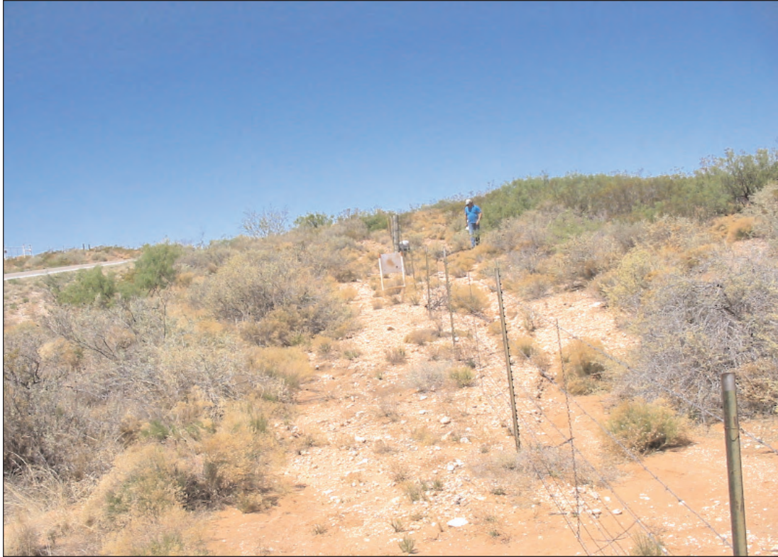
Figure 5. Eroded feature area next to right-of-way fence, LA113042.
