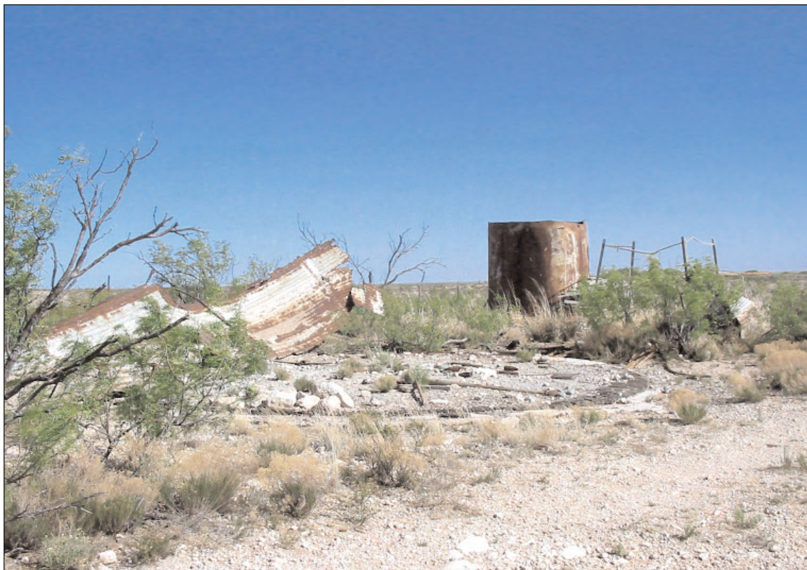
Figure 15. Water tank features outside project limits south of NM 128, LA 129220.
