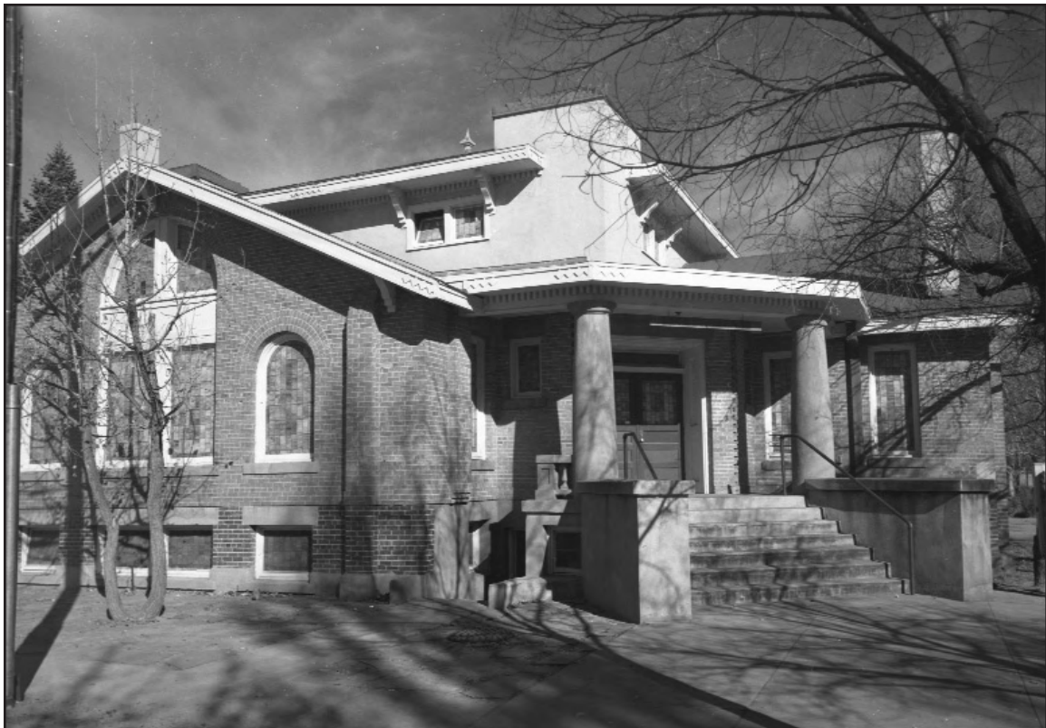
Figure 15. The First Baptist Church, ca. 1949. Museum of New Mexico Neg. No. 73834.
