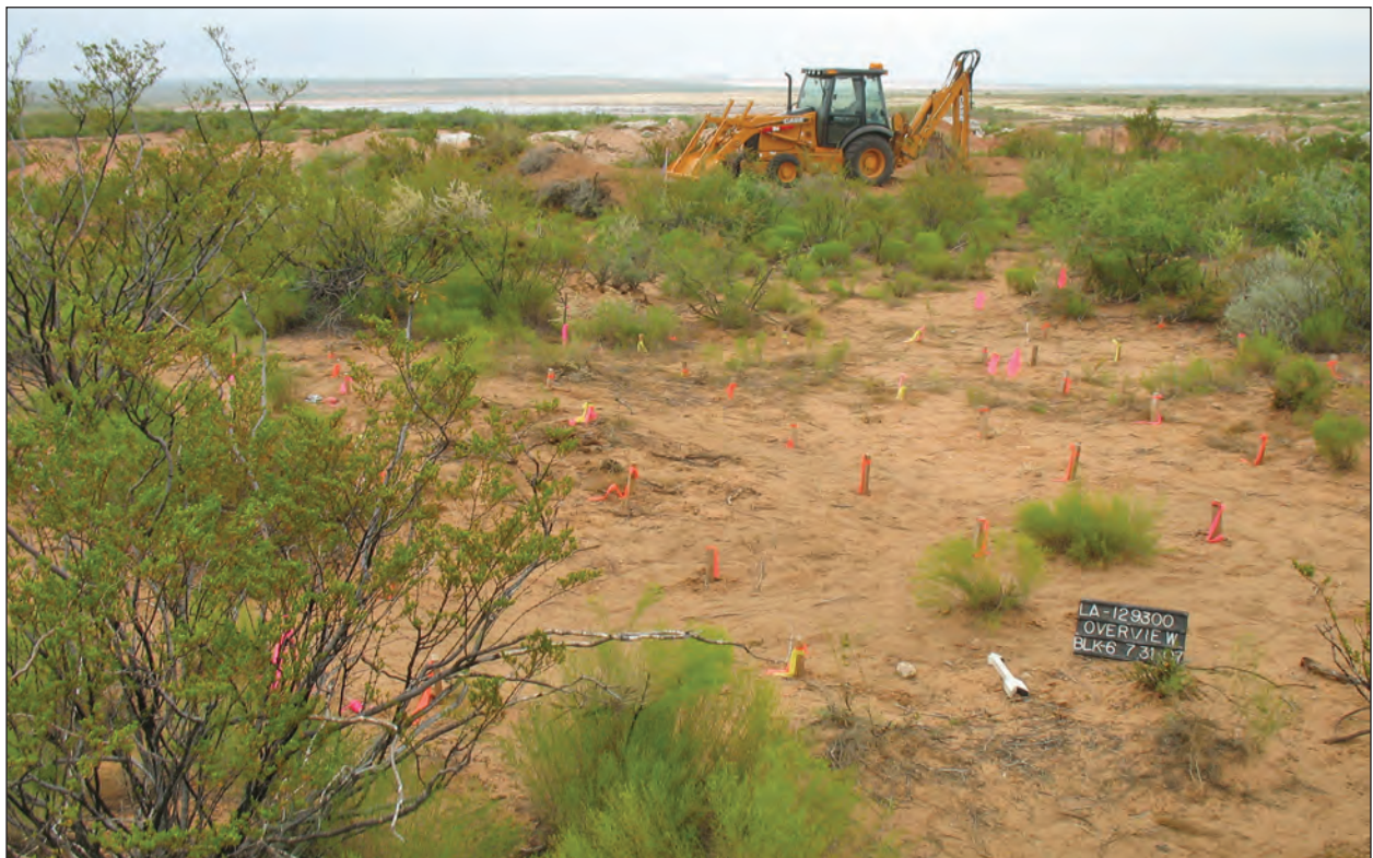
Figure 13.10. LA 129300, Block 6, at ready for excavation.
