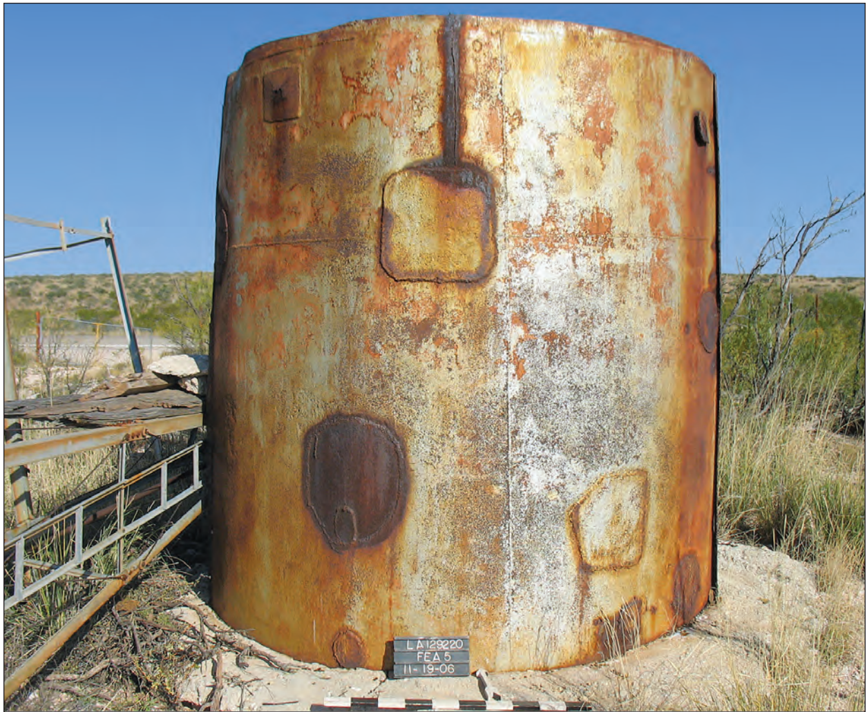
Figure 14.6. LA 129220, Feature 5, a standing, solid metal tank – note the welded patches.
