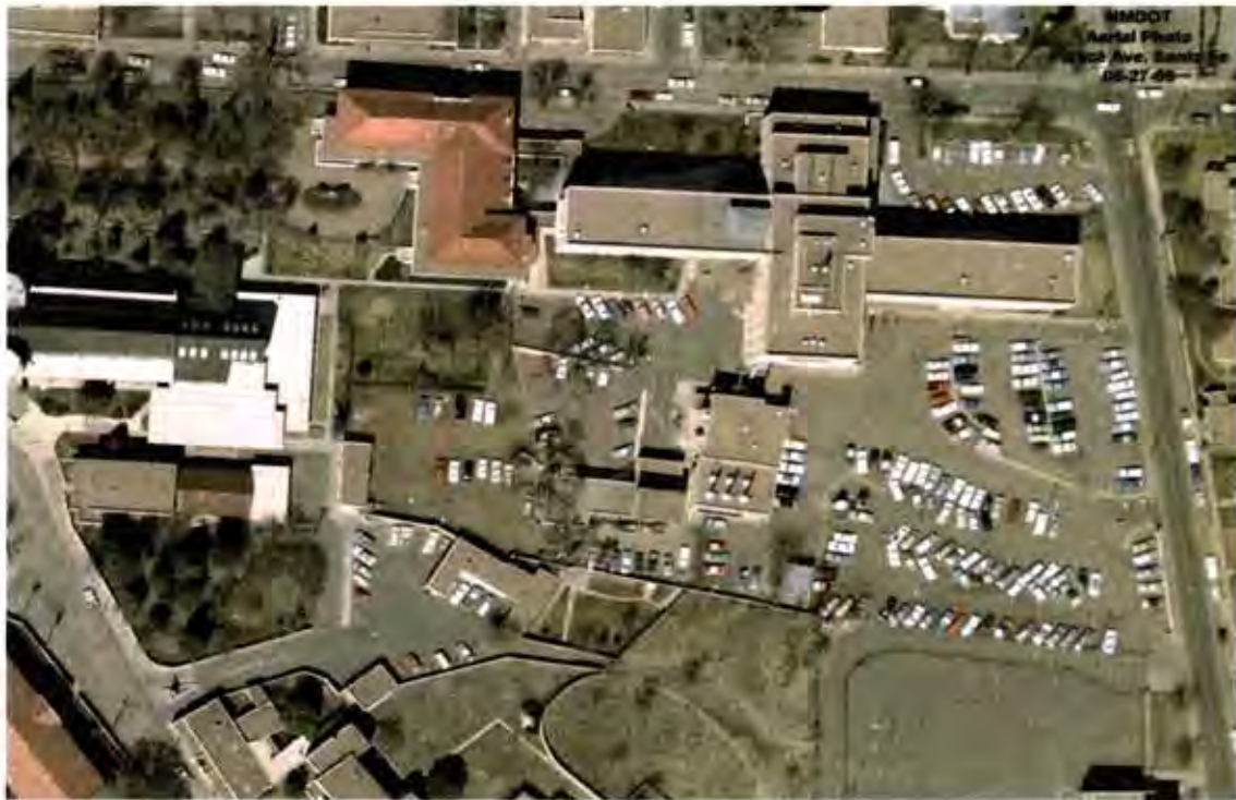
Fig. 1. Aerial view of the project area. New Mexico DOT photo taken June 27, 1969.
