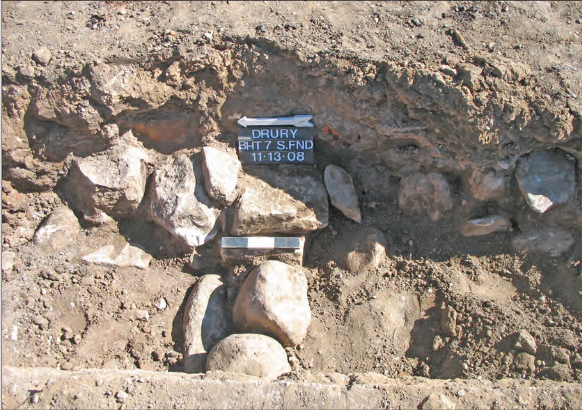
Figure 15. South end of BHT 7, showing the cobble and limestone block foundation.
