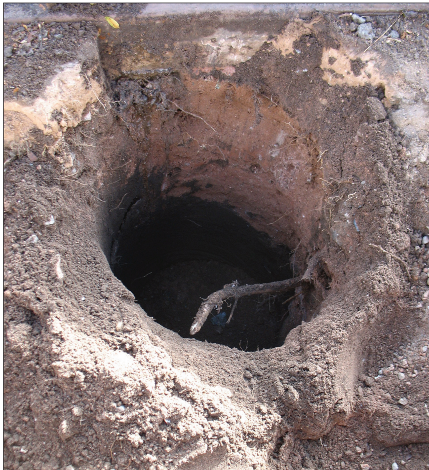
Figure 5. Excavated light-post hole.
