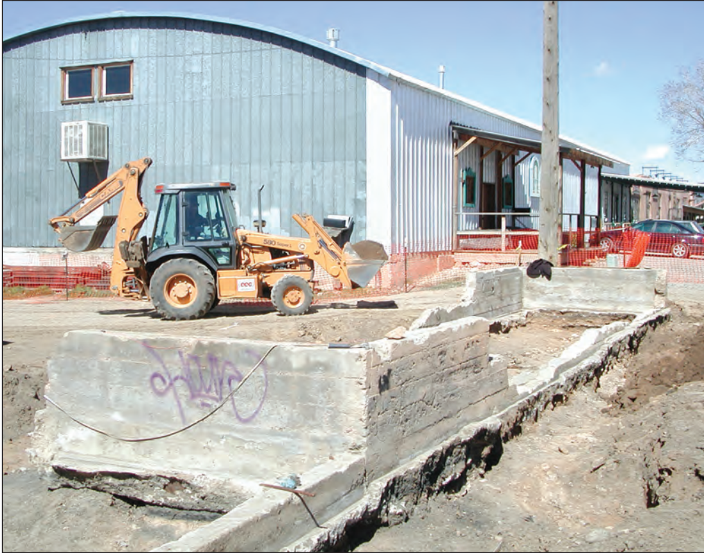
Figure 4.6. LA 146405, Structure 1.1, foundation, view to the north.
