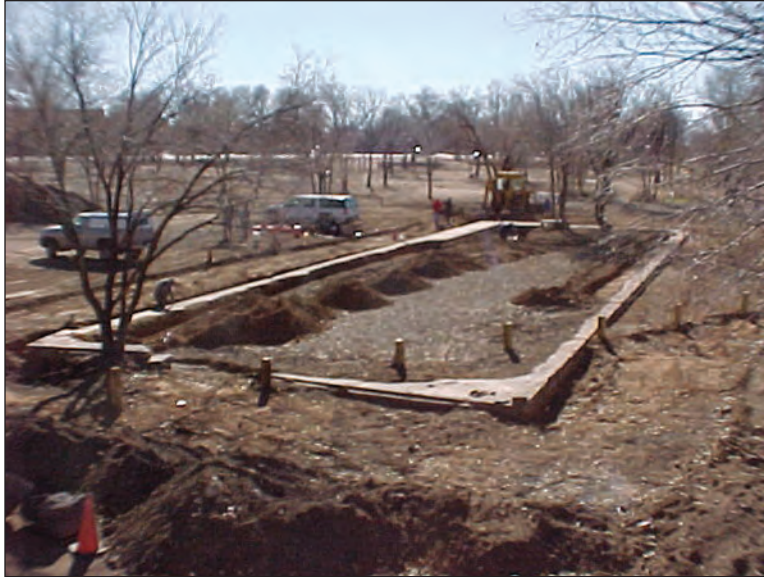
Figure 6.12. LA 146411, overview of Structure 1, view to the south.
