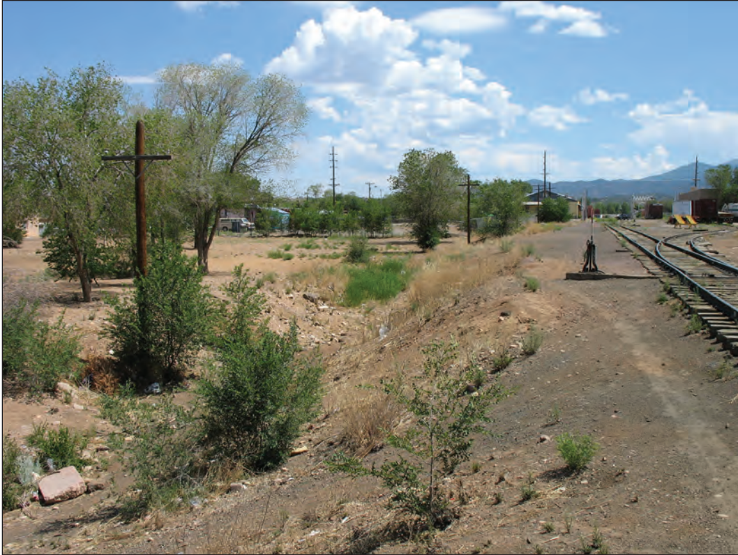
Figure 6.37. LA 153442, view of intact poles with insulators along the railroad tracks, facing northeast toward the Paseo de Peralta crossing.
