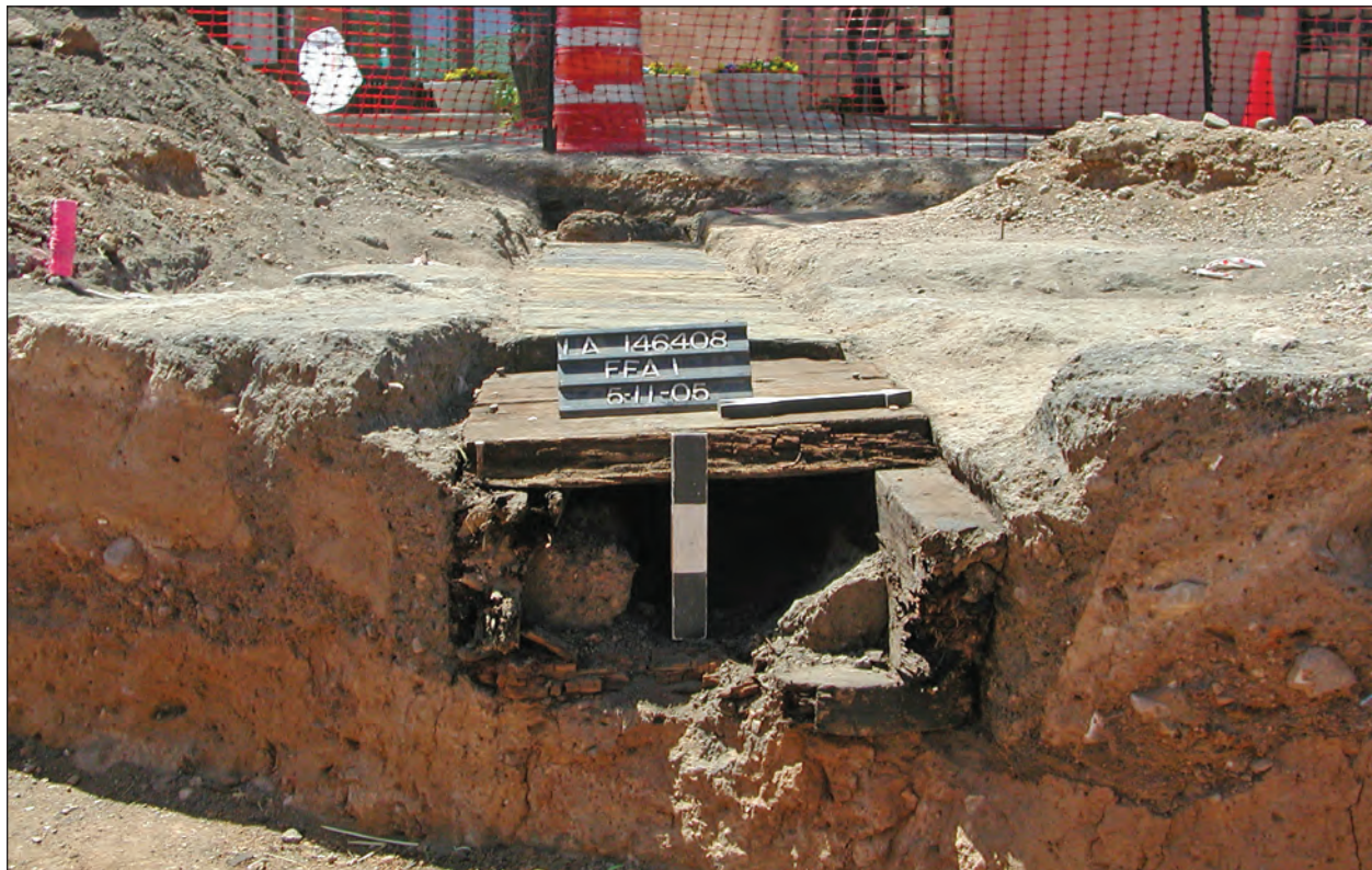
Figure 2.7. LA 146408, BHT 51, west wall, Features 1 and 28, cross sections after excavation of overburden, showing construction details.
