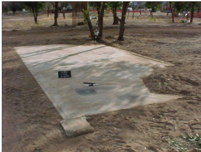
Figure 6.31. LA 149919, Feature 1015, view of the concrete slab in the southeastern corner.
