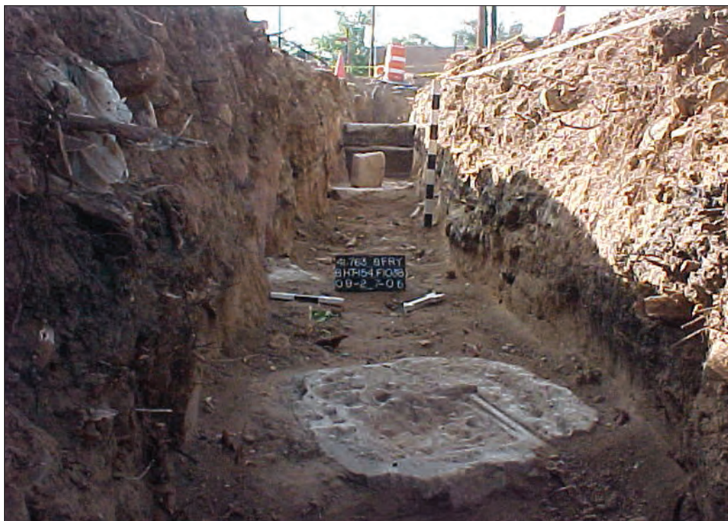
Figure 6.24. LA 149916, Feature 1038, from the north. The array of concrete piers occupies the foreground and the concrete wall foundation is visible in the background.
