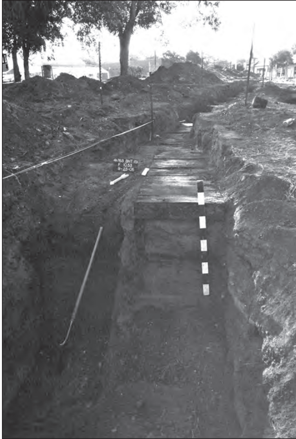
Figure 4.18. LA 149911, view of Feature 1033, a wooden culvert crossing under the railroad tracks.
