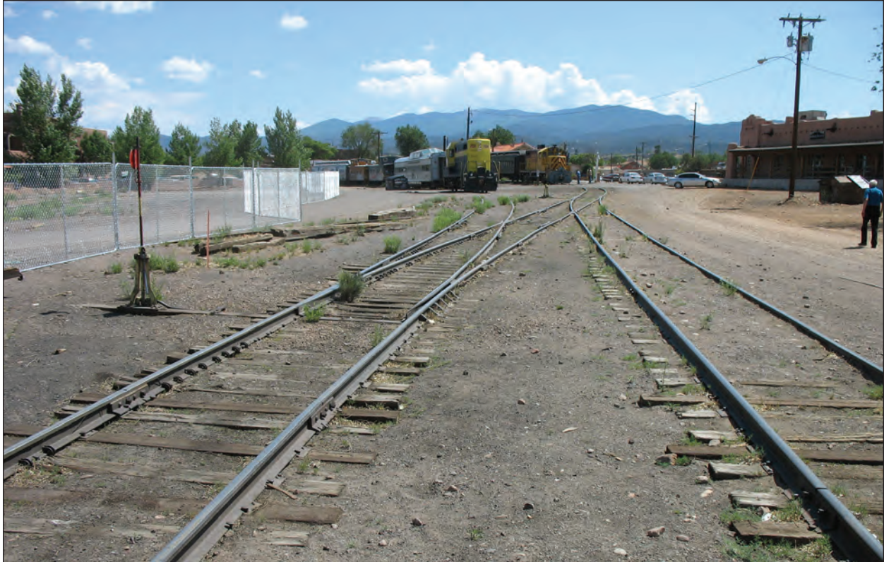
Figure 3.109. View of railroad tracks (LA 153441) in the Santa Fe Railyard, facing northeast toward the Manhattan Avenue crossing. The 1909 AT&SF depot is in the background, behind the locomotives; note the manual switch stand in the left mid-ground.
