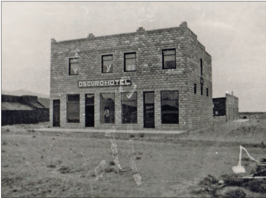
Figure 4.3. Oscuro Hotel, ca. 1915. The second floor had eight rooms; the ground floor had two smaller guest rooms, a dining room, and a kitchen (courtesy Helen Shields).
