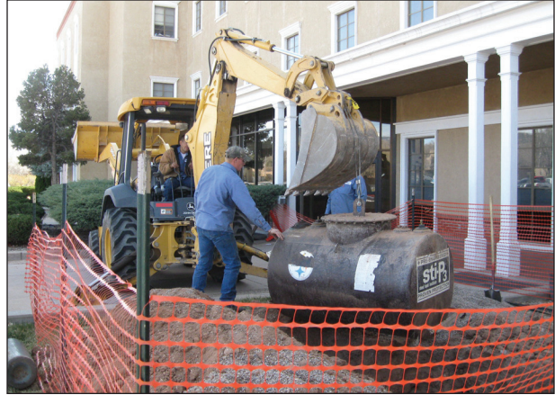
Figure A2.14. Tank removal, facing south.
