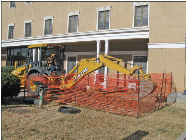
Figure A2.11. Backhoe, facing west.
