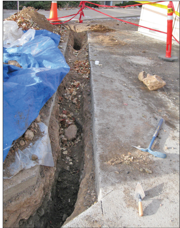
Figure A2.2. Trench, facing west.
