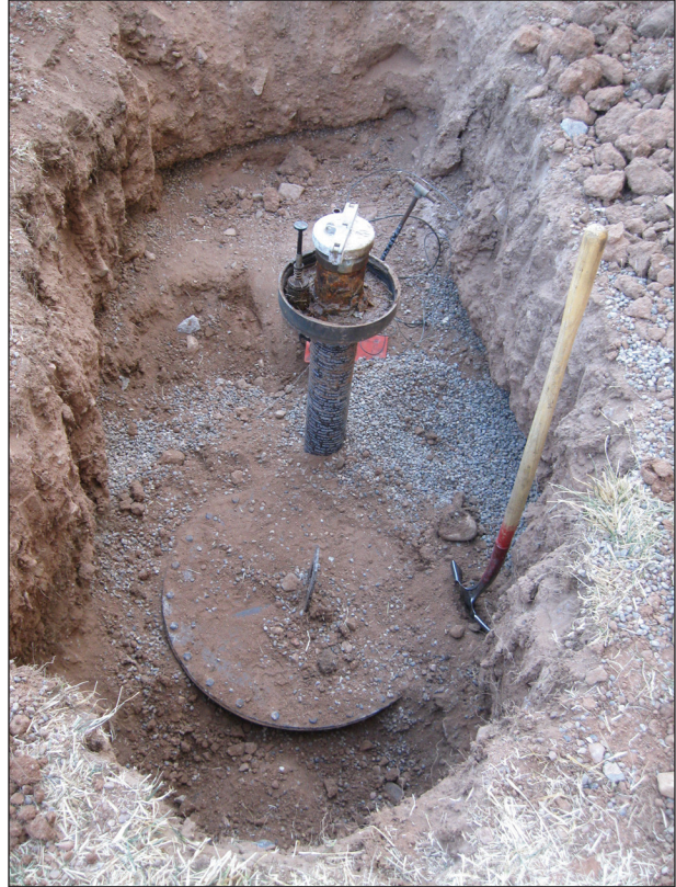
Figure A2.10. Fuel gauge attached to diesel tank, facing south.
