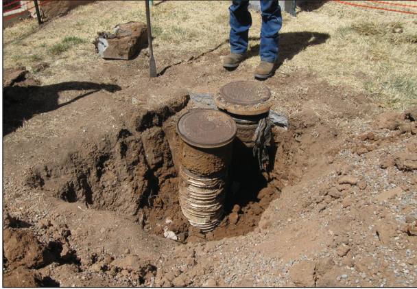
Figure A2.9. Metal manhole covers above steel diesel tank, facing northwest.
