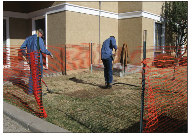
Figure A2.8. Excavation area, facing northwest.
