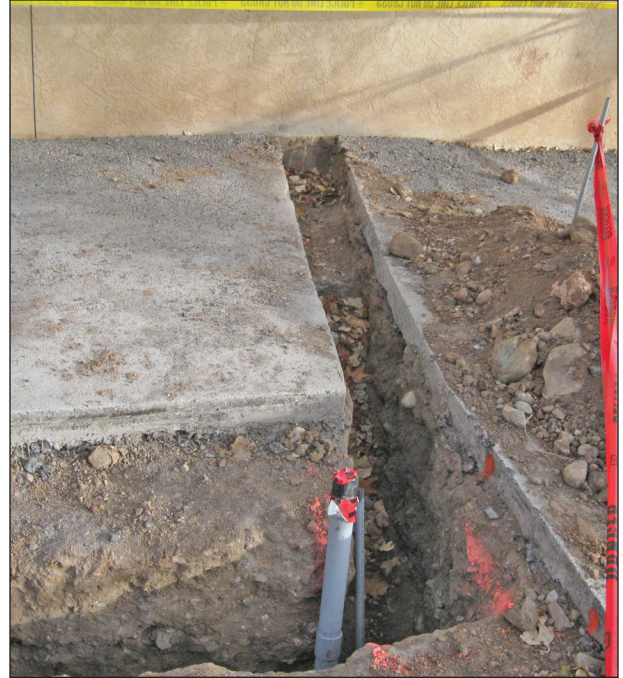
Figure A2.6. Short north-south trench to PERA Maintenance Shop, facing north.
