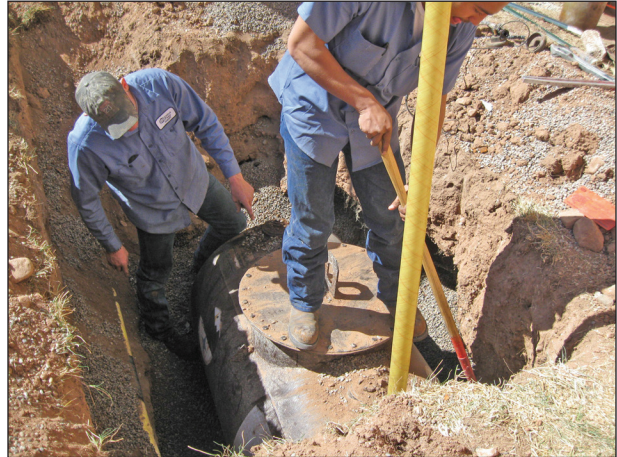
Figure A2.12. Tank in pit, facing south.
