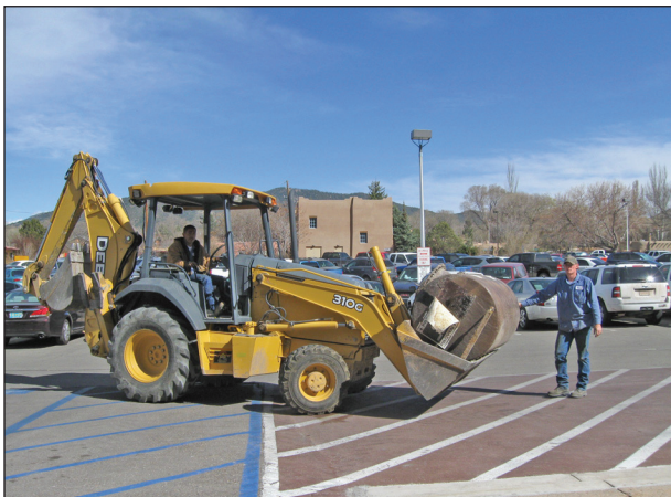
Figure A2.15. Tank removed from pit, facing south.
