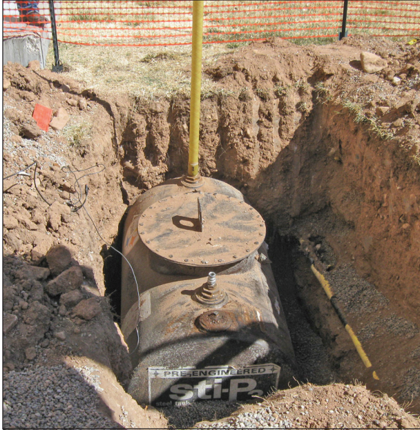
Figure A2.13. Tank partially removed from pit, facing north.
