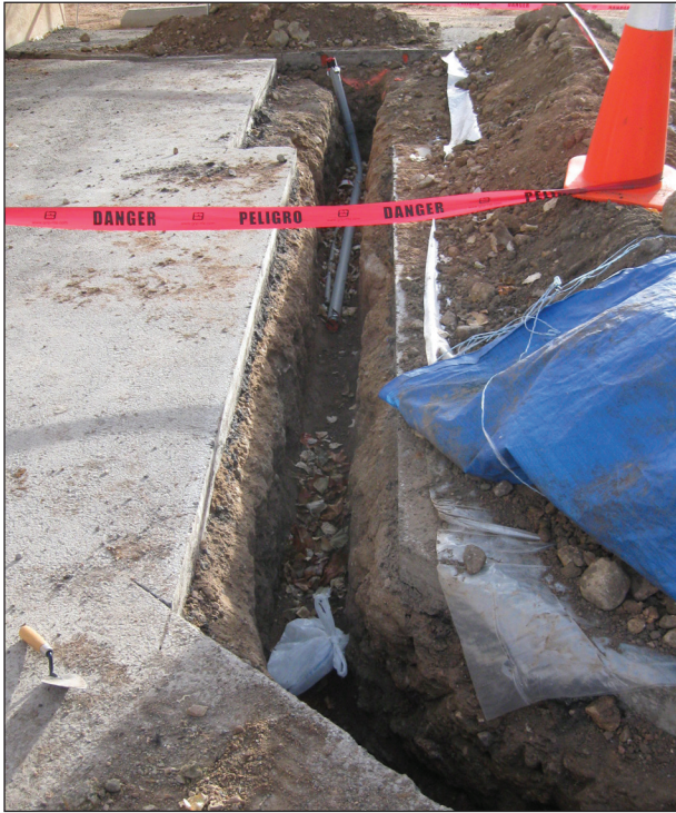
Figure A2.1. Trench with bag of human remains, facing east.
