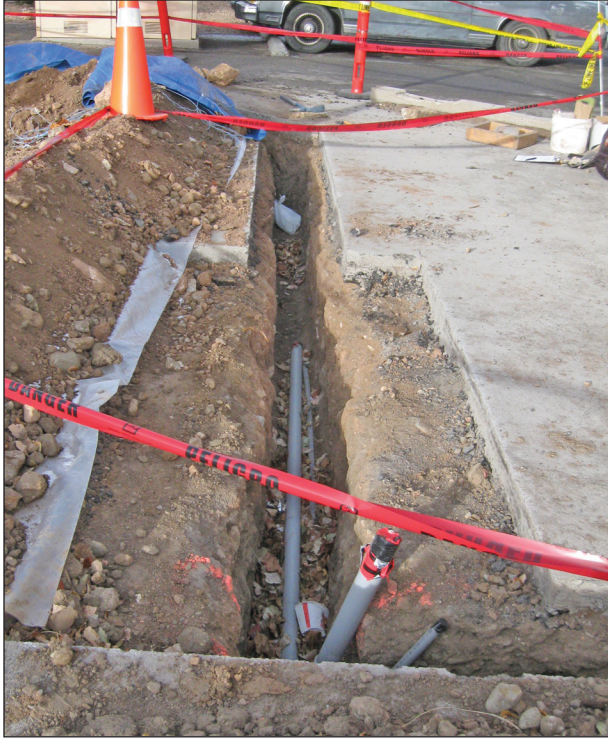
Figure A2.5. Entire trench, facing west.
