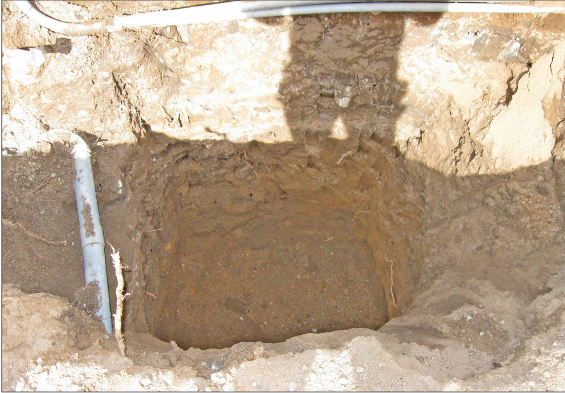
Figure 7. TU 1 after excavation.
