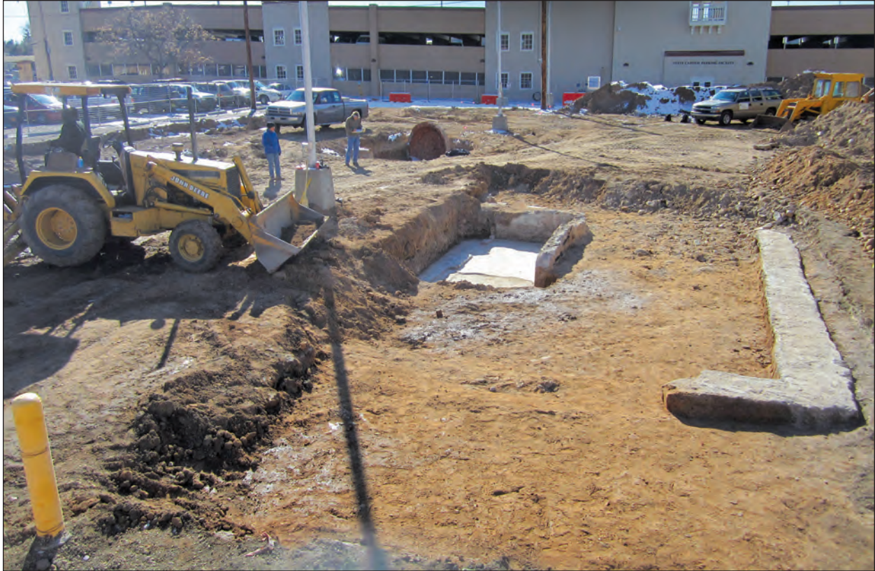
Figure 14.6. Structure 12, foundations and basement.
