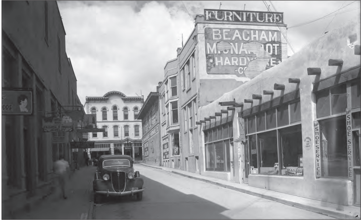
Figure 13.1. Beacham-Minardot Hardware, ca. 1925-45 (courtesy Palace of the Governors Photo Archives, NMHM/DCA, neg. no. 011124).
