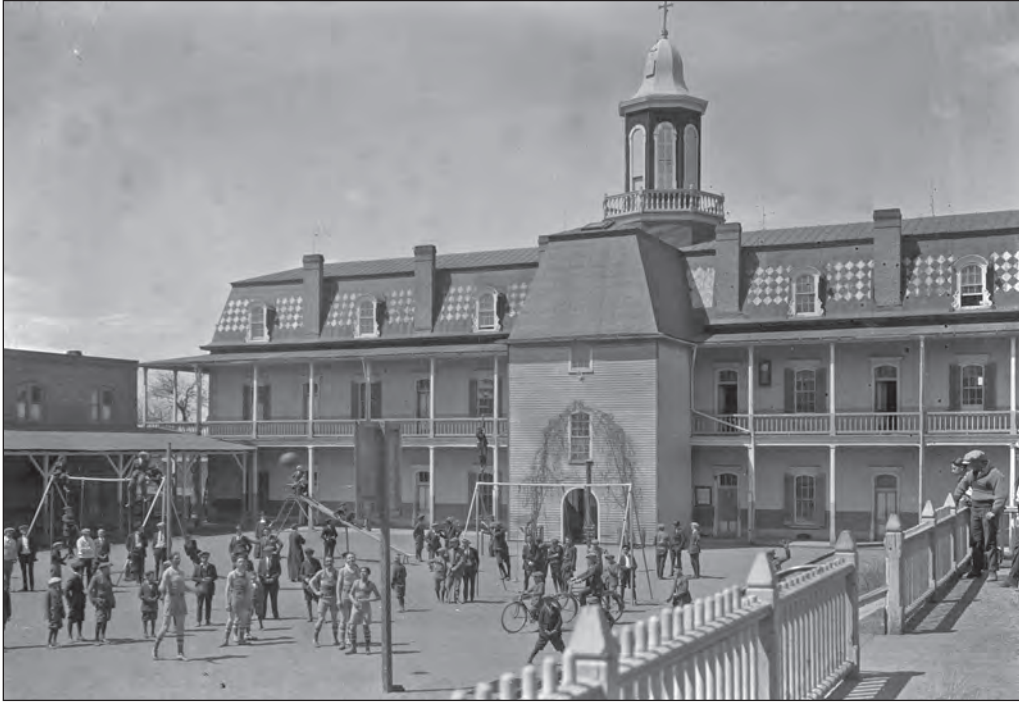
Figure 4.4. St. Michael's Playground with dormitory, now the Lamy Building, in the background, ca. 1924 (courtesy Palace of the Governors Photo Archives, NMHM/DCA, neg. no. 051336).
