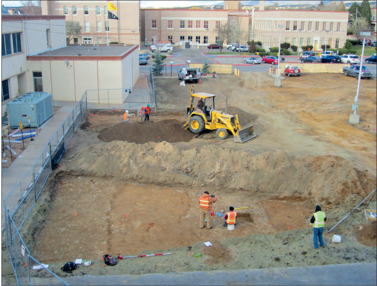
Figure 7.3. The excavation of Scraping Units 10 and 11.
