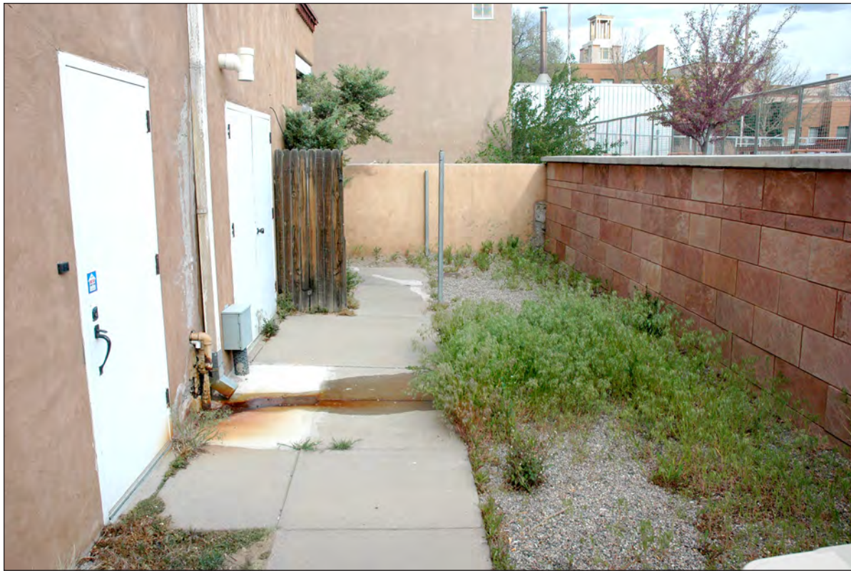
Figure 19. View west toward Area 3. The utility replacement will be conducted at the far end of the walled area.
