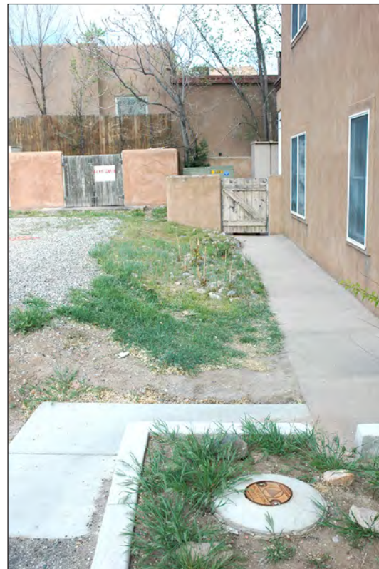
Figure 17. View west of Area 1, the northeast corner of the District Attorney building.
