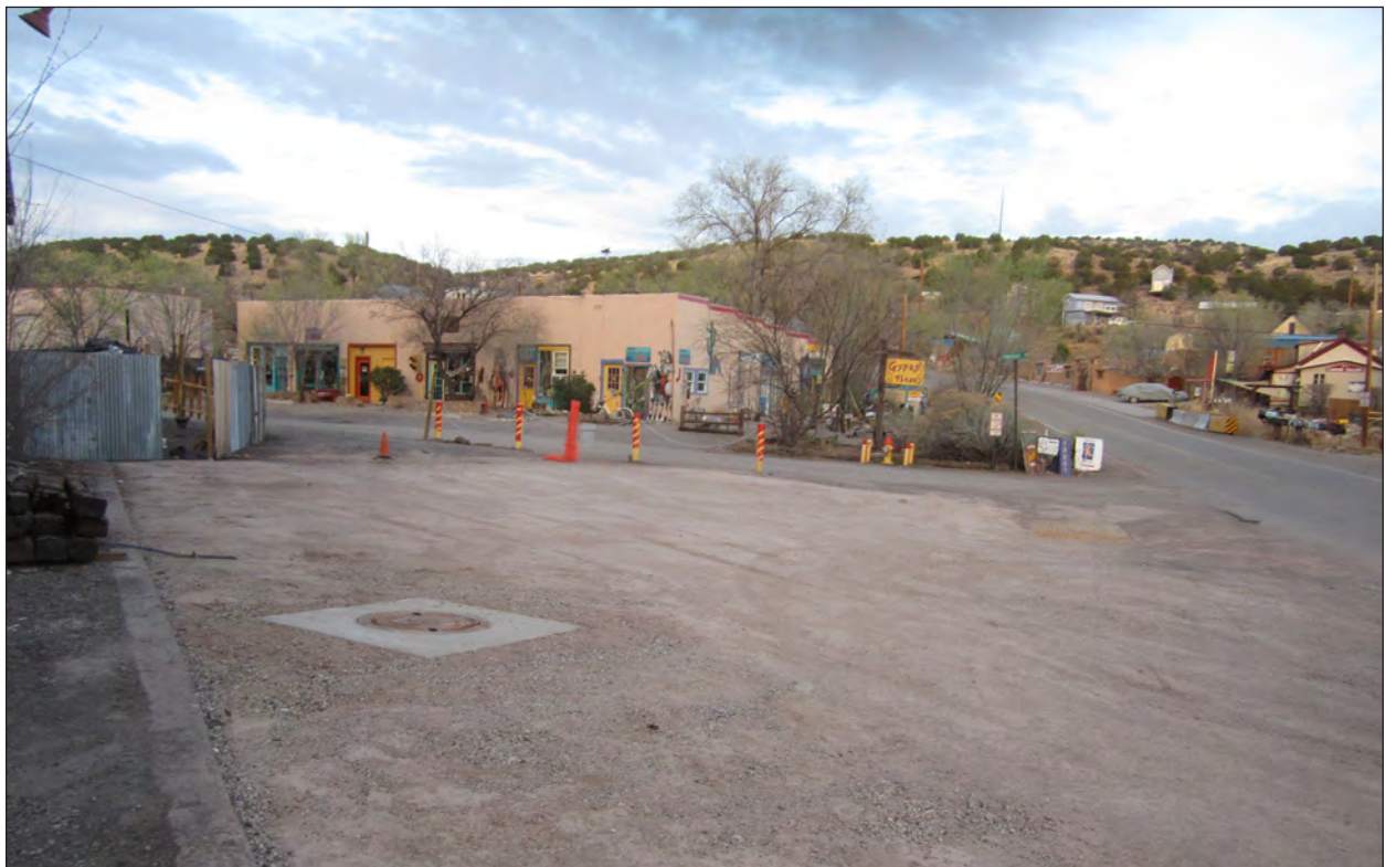
Figure 6.74. The completed Mine Shaft Tavern parking lot, view south.
