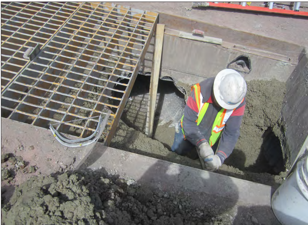
Figure 6.32. Crew builds a concrete swale inside lower drop inlet, view west.
