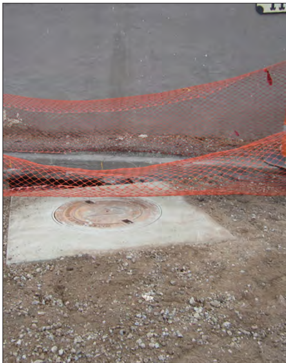
Figure 6.34. Completed manhole, west of the tavern porch, view east.
