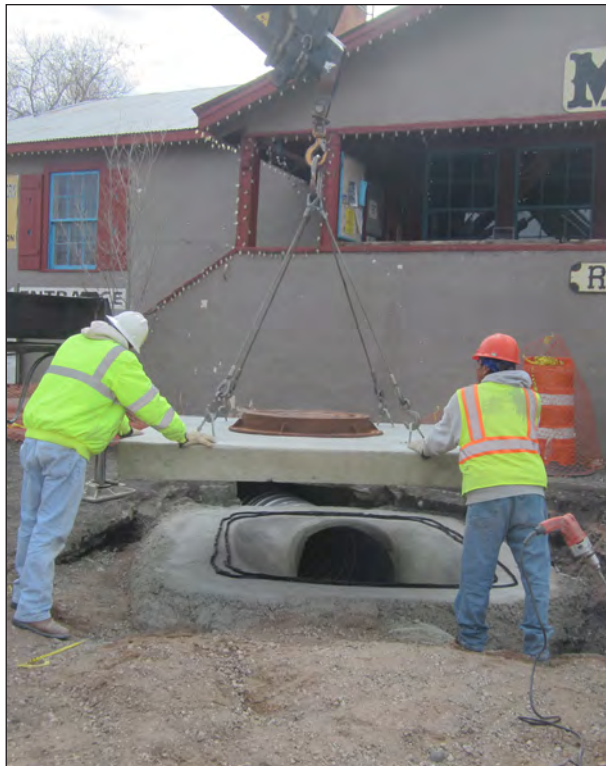
Figure 6.29. Pre-made lid is set on manhole base, view east.
