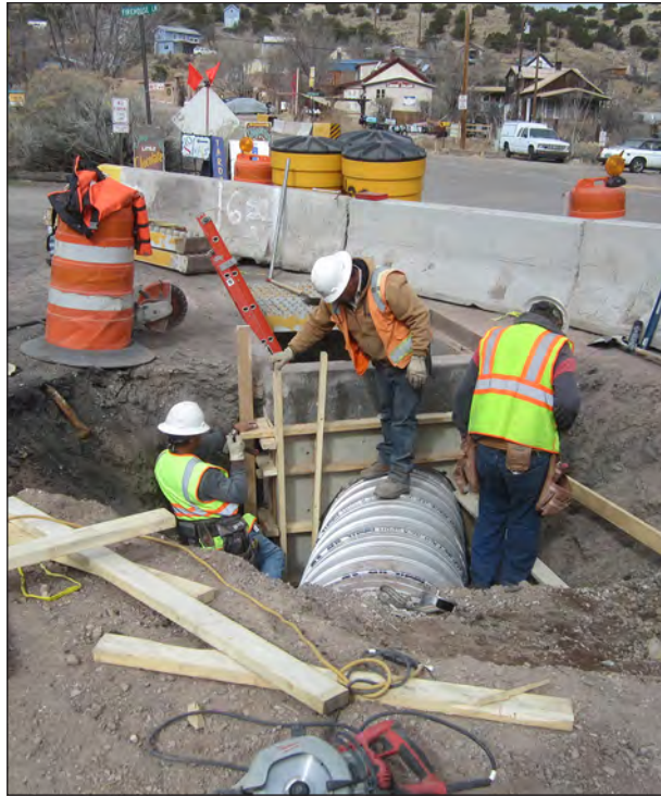
Figure 6.31. Crew prepares concrete forms at lower inlet, view southwest.
