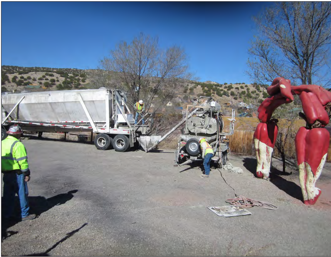
Figure 6.60. Con Deck crew sets up grouting operation, view west.
