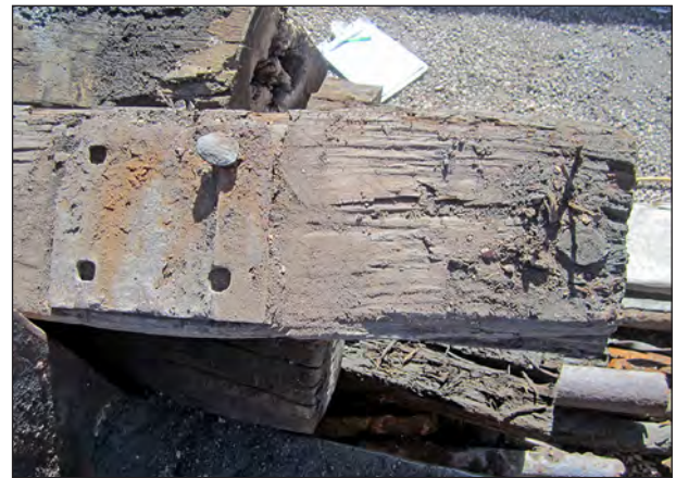
Figure 6.53. Metal tie plate attached to railroad tie with spikes, view east.
