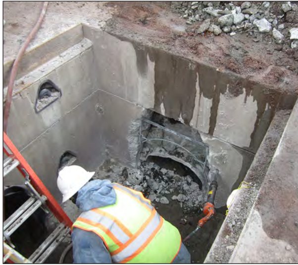
Figure 6.9. Clearing interior of lower box inlet, view west.
