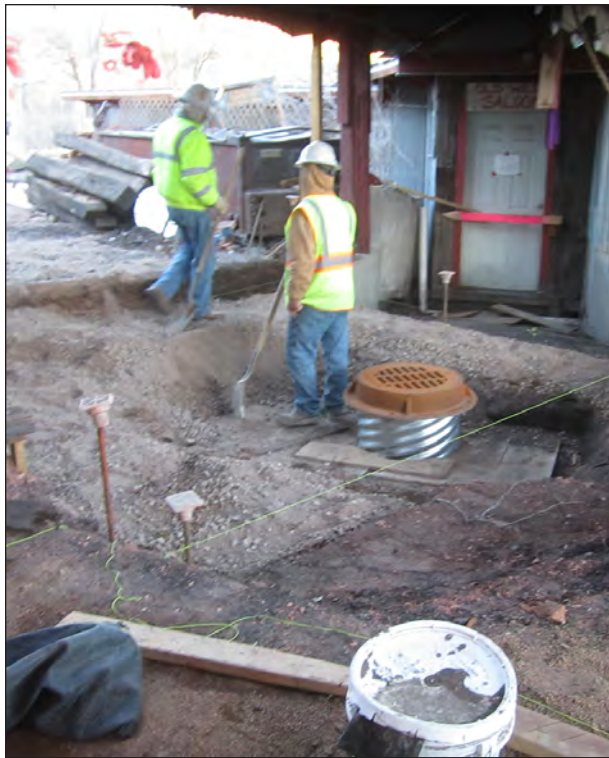
Figure 6.75. AUI crew fills manhole pit with base course, view west.
