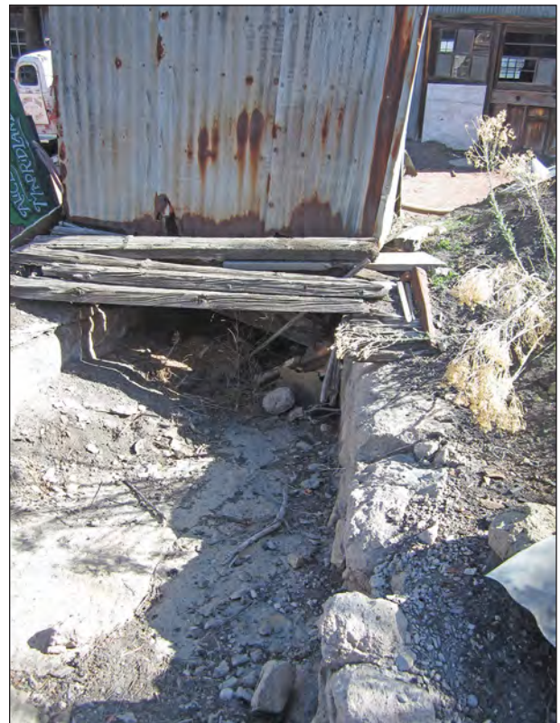
Figure 6.64. LA 126142, Feature 26, concrete culvert under old pump house, view north.
