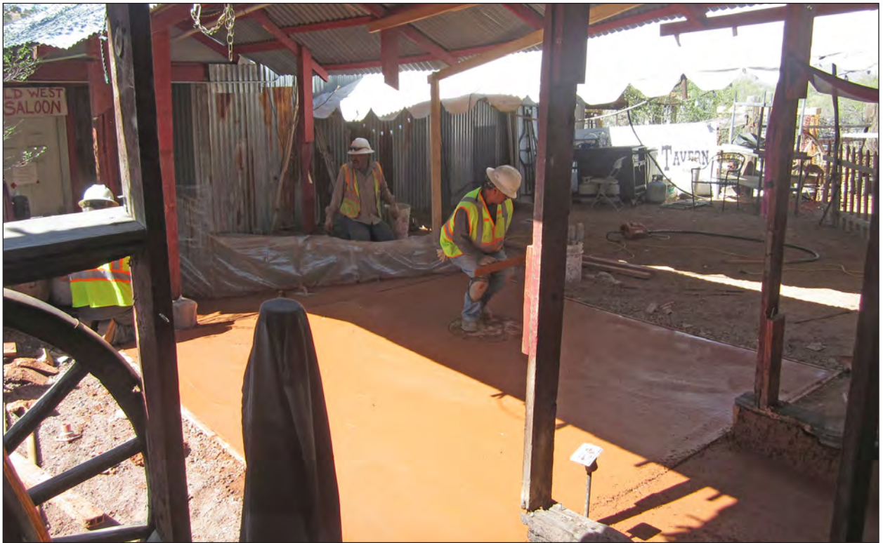
Figure 6.77. AUI crew pours concrete pad at the theatre walkway, view west.
