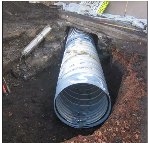
Figure 6.19. Additional section of the recently installed slip liner, view northeast.
