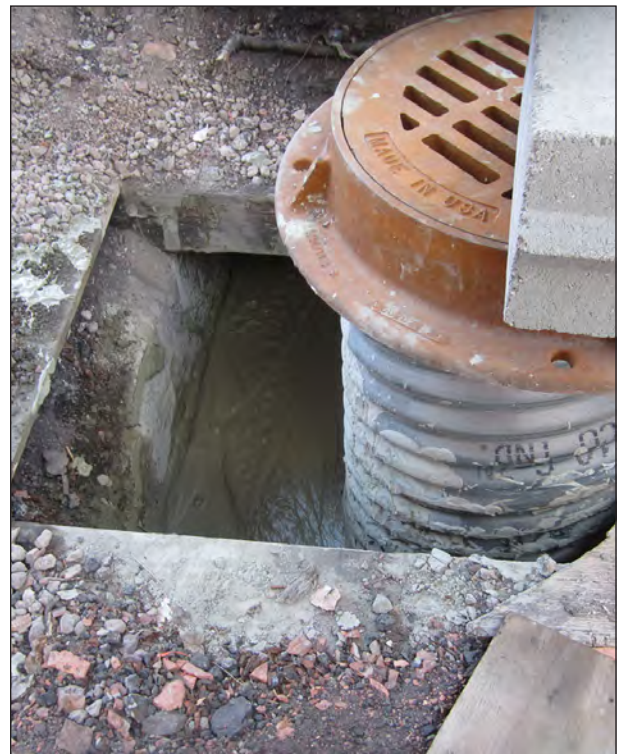
Figure 6.70. Grouting in progress at the theatre walkway manhole, view west.
