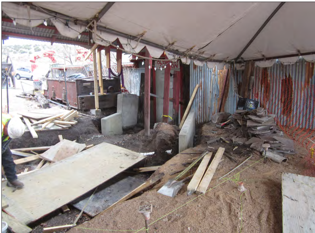
Figure 6.49. Forms removed from walls near the theatre walkway, view southeast.
