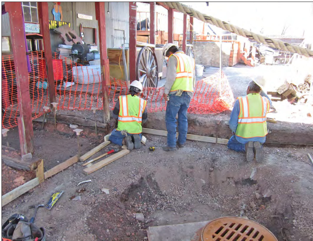
Figure 6.76. AUI crew sets concrete forms at the theatre walkway, view south.
