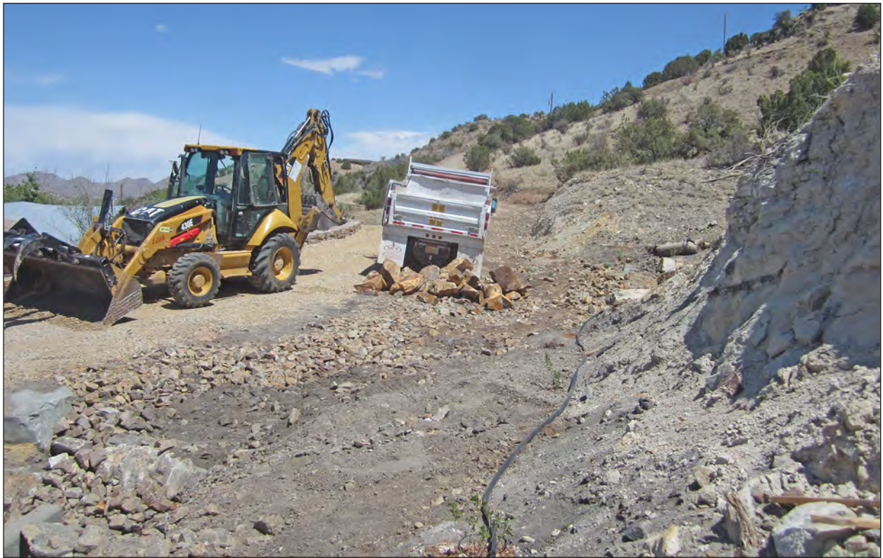
Figure 6.81. Truck with landscaping boulders for upper drop inlet, view north.
