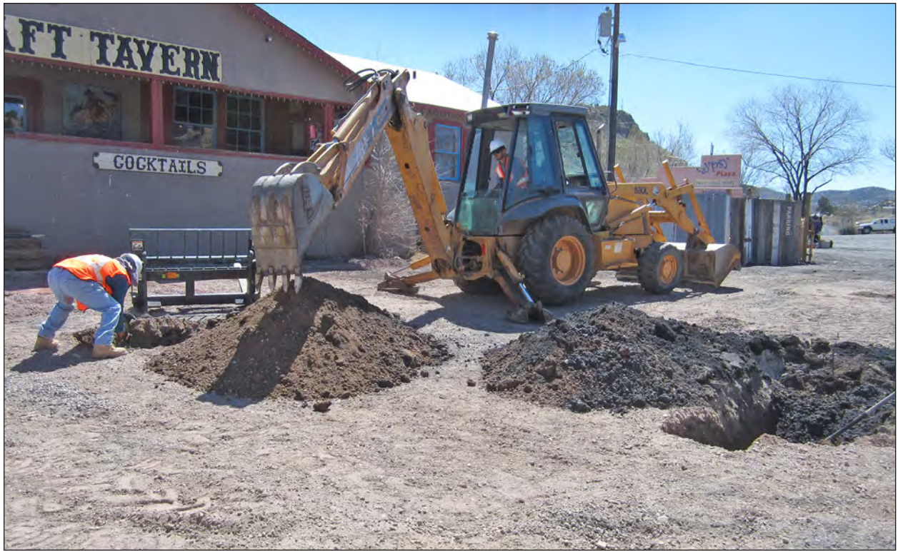
Figure 6.71. JC Septic crew members trench for septic lines, view east.
