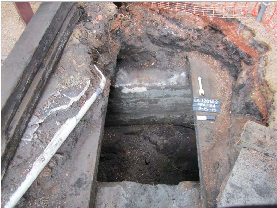
Figure 8.91. Feature 12, box culvert filled with gob and sediment, view north.
