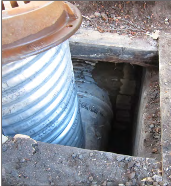
Figure 6.56. Initial grout pour at the theatre walkway manhole, view east.
