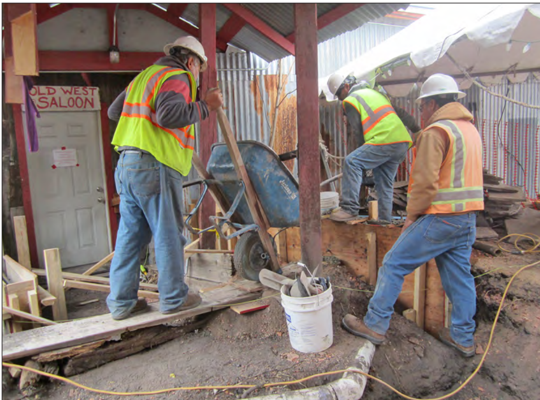
Figure 6.47. Crew pours concrete into north wall forms, view northwest.
