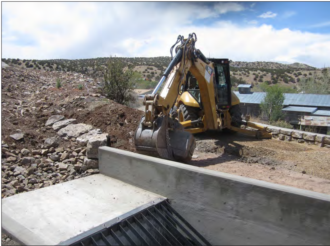
Figure 6.83. Steve Carson aligns boulders south of upper drop inlet, view southwest.
