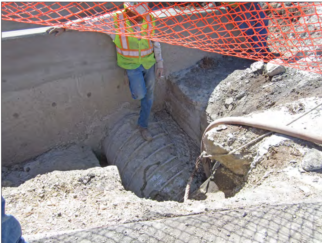
Figure 6.68. Con Deck crew member pumps grout into upper inlet, view east.
