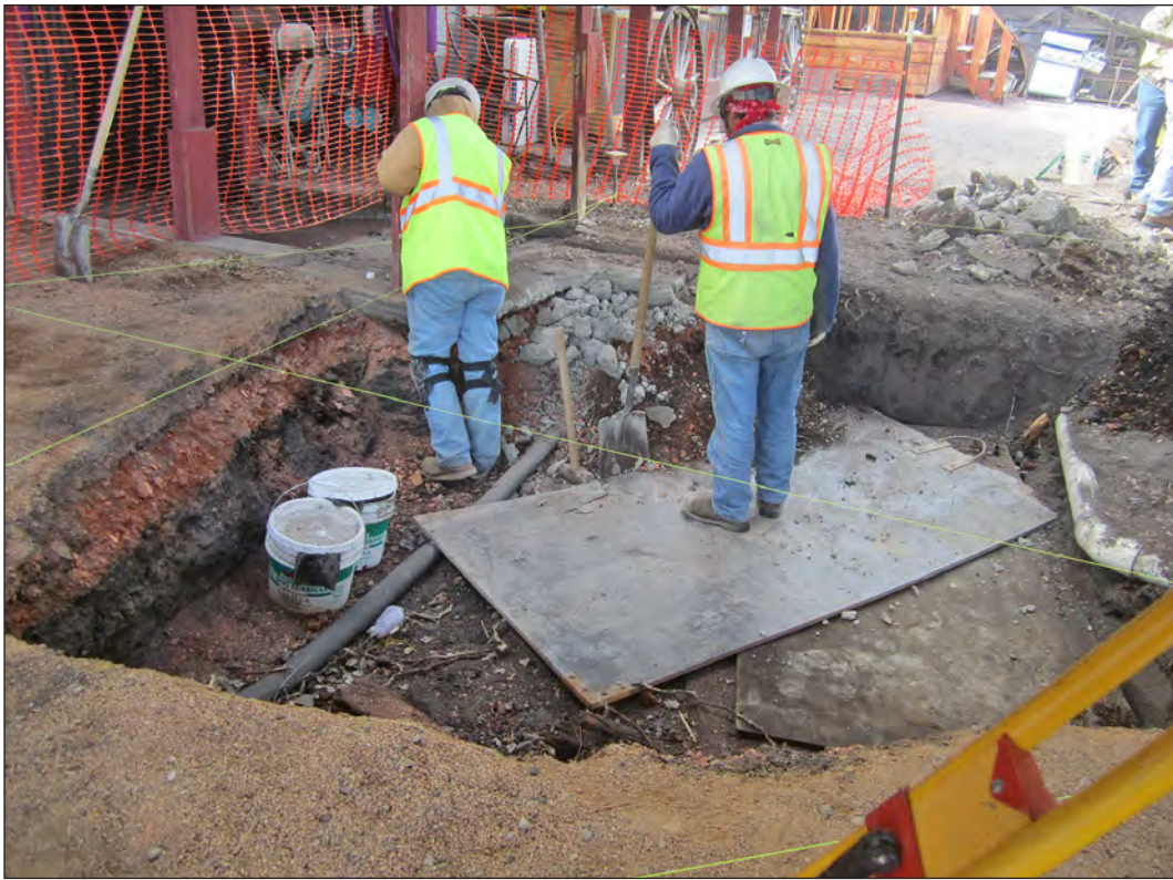
Figure 6.44. Crew removes the cement pad at the theatre walkway, view south.
