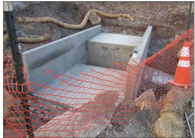
Figure 6.42. Completed upper drop inlet, view southeast.
