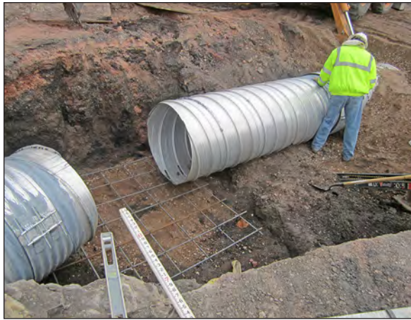
Figure 6.26. Rebar grid is installed at base of manhole, view west.
