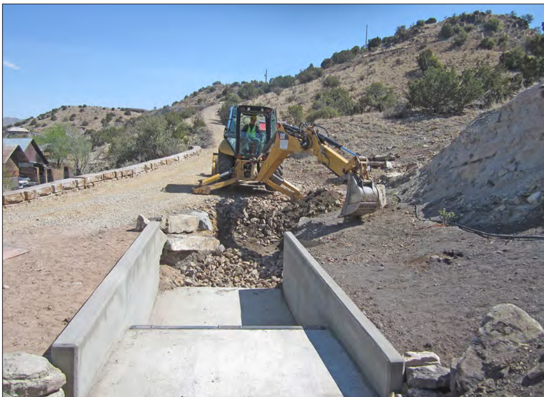
Figure 6.82. Steve Carson aligns boulders north of upper drop inlet, view north.
