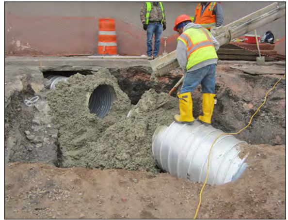
Figure 6.27. Concrete is poured for manhole, view east.
