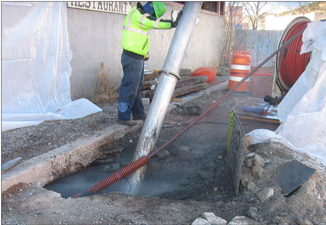
Figure 6.4. Jet-vacuuming the western end of Feature 12 box culvert, view east.
