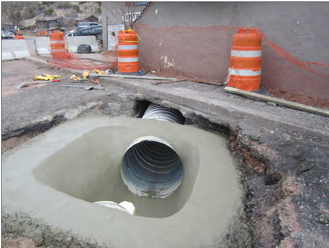
Figure 6.28. Hand-formed concrete manhole base, view northeast.
