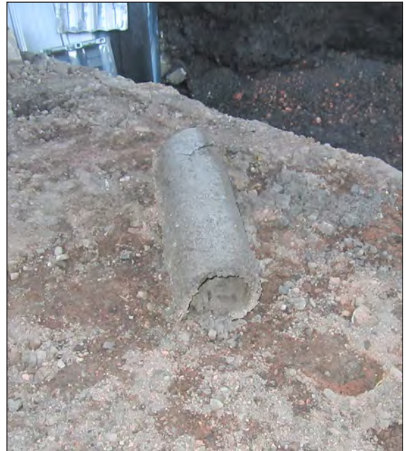
Figure 6.23. Section of Orangeburg pipe, view northeast.
