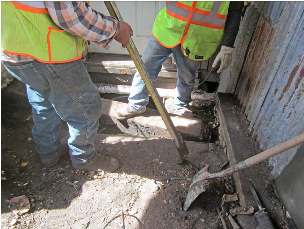
Figure 6.51. AUI crew removes railroad ties from the saloon doorway, view west.
