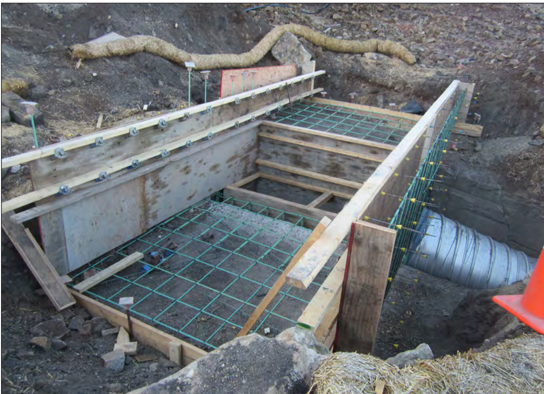
Figure 6.39. Completed wall and apron forms upper inlet, view southeast.
