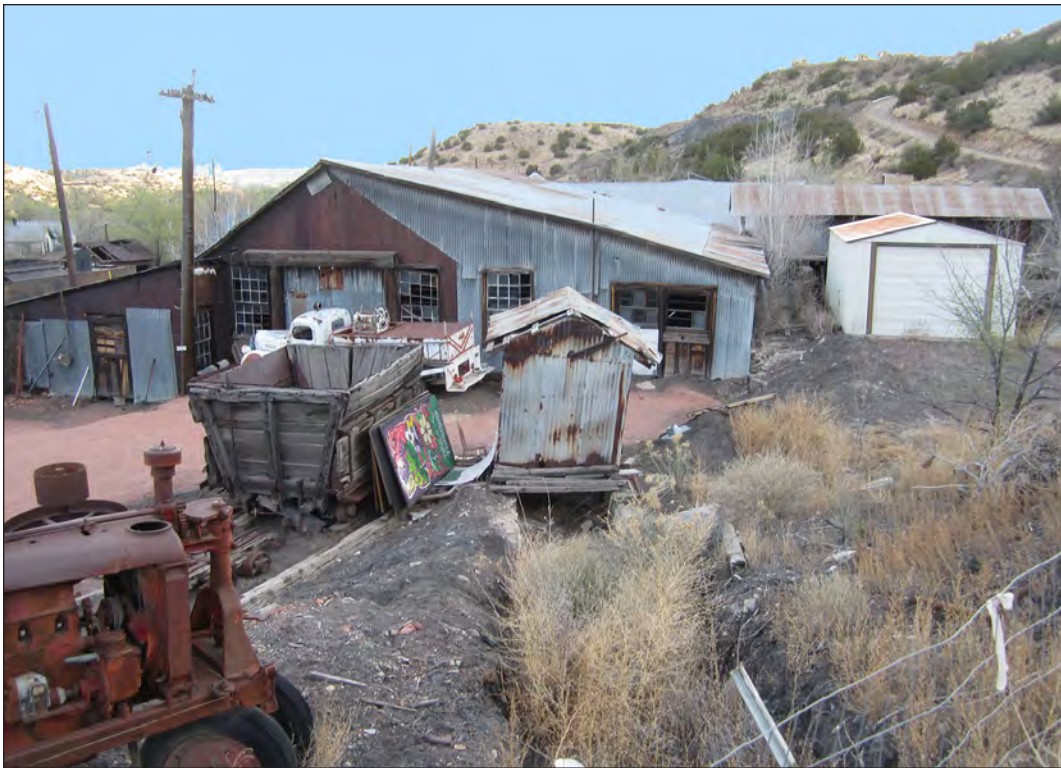
Figure 6.65. Pump house with concrete culvert, view north.
