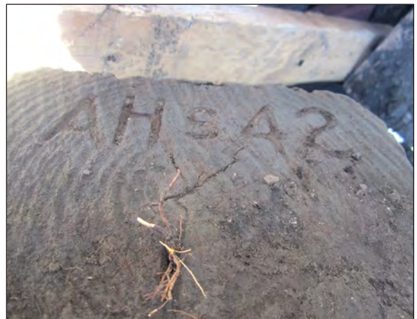
Figure 6.59. Stamped end of railroad tie.
