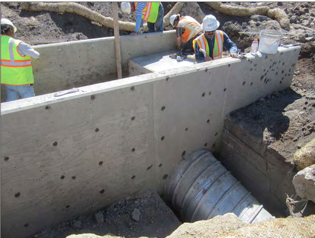
Figure 6.41. Concrete walls with slip liner at upper inlet, view southeast.
