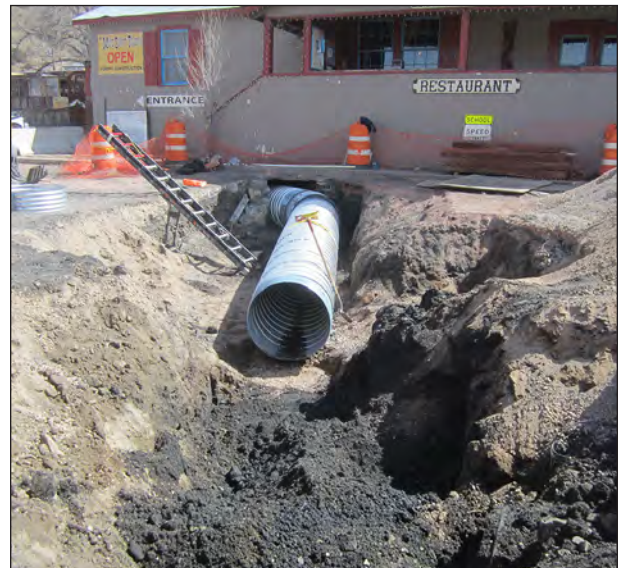
Figure 6.20. Elbow installed on slip liner, view east.
