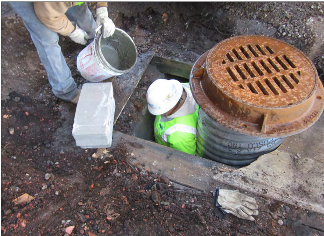
Figure 6.55. AUI crew installs side walls in Feature 12 slip liner, view west.
