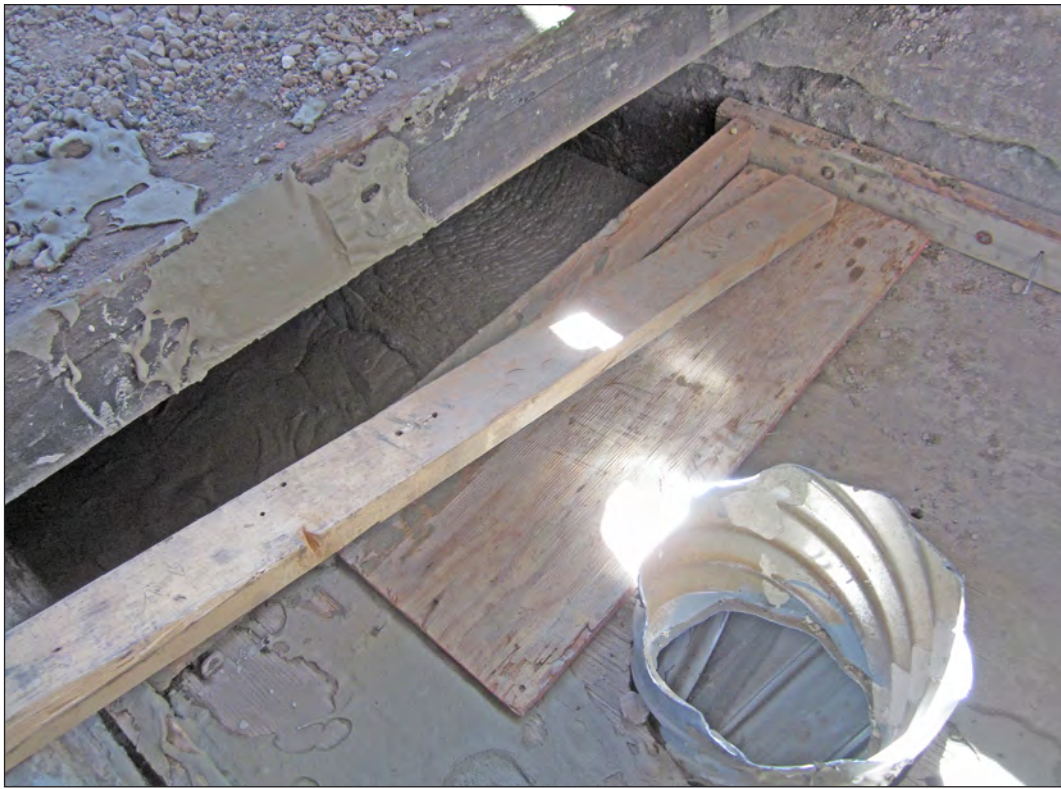
Figure 6.69. Inlet, with grout, at the saloon's doorway, view southwest.
