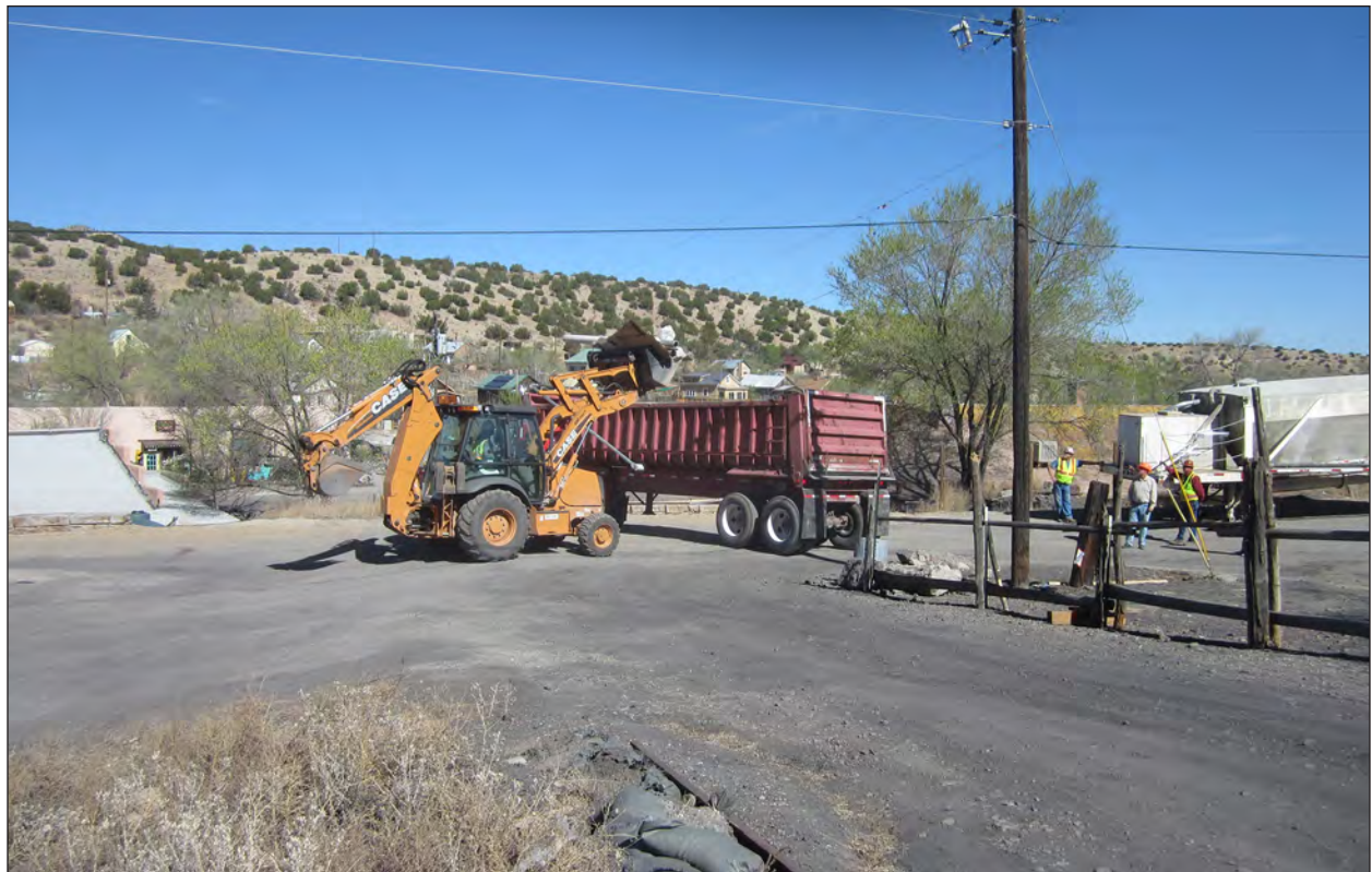
Figure 6.80. Trash is removed from the site, view northwest.
