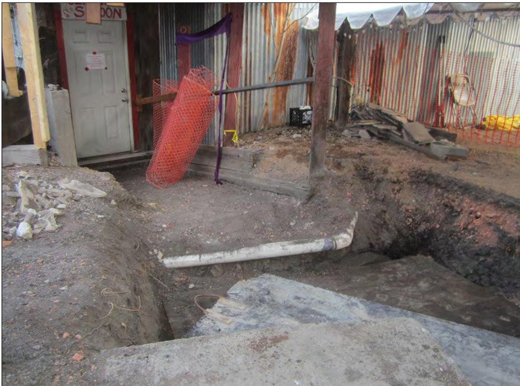
Figure 6.43. Theatre walkway prior to reconstruction, view north.
