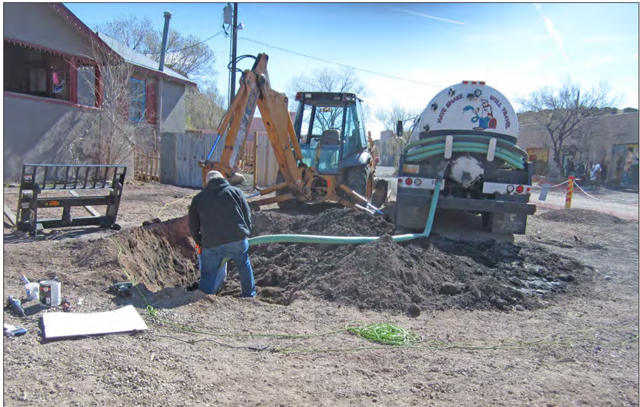
Figure 6.72. A JC Septic crew member pumps sewage from trench, view southeast.
