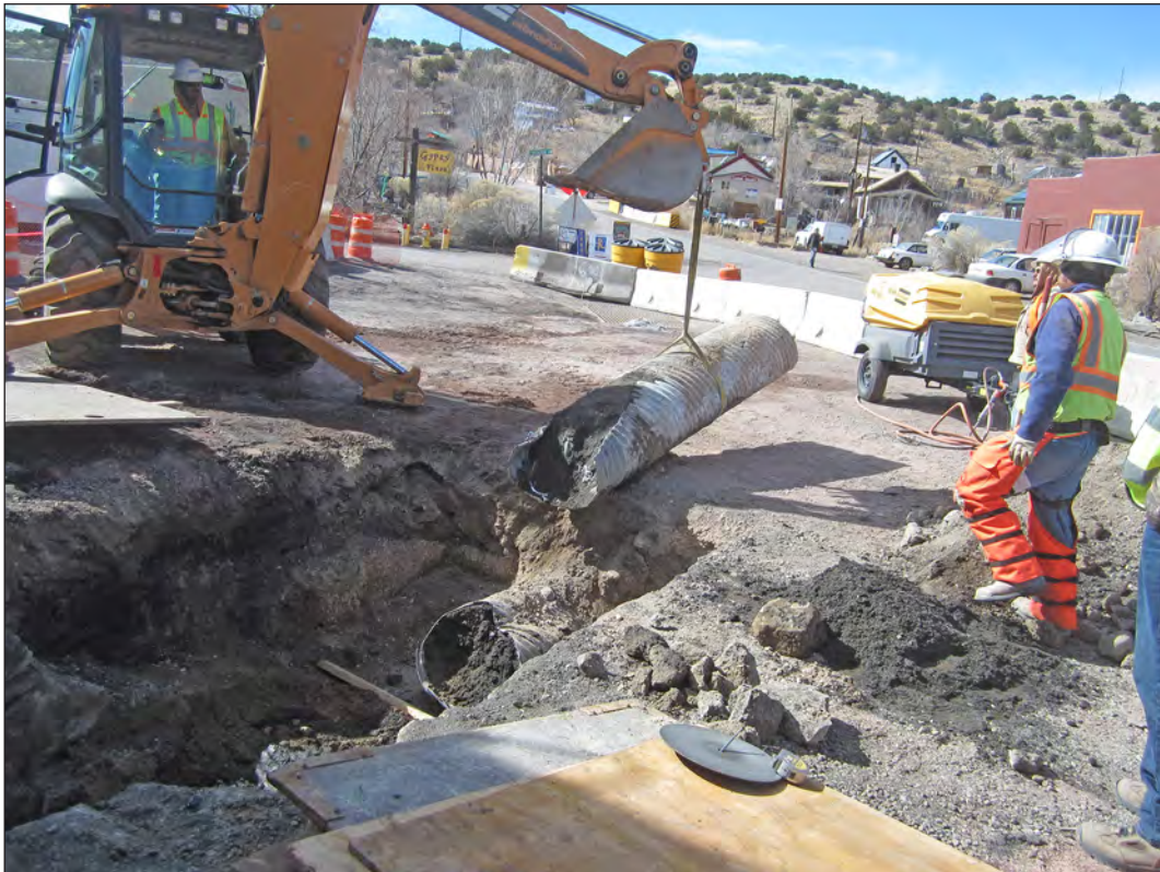
Figure 6.11. Removal of old culvert filled with gob and sediment, view southwest.
