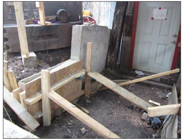
Figure 6.48. Poured south wall in the theatre walkway, view west.
