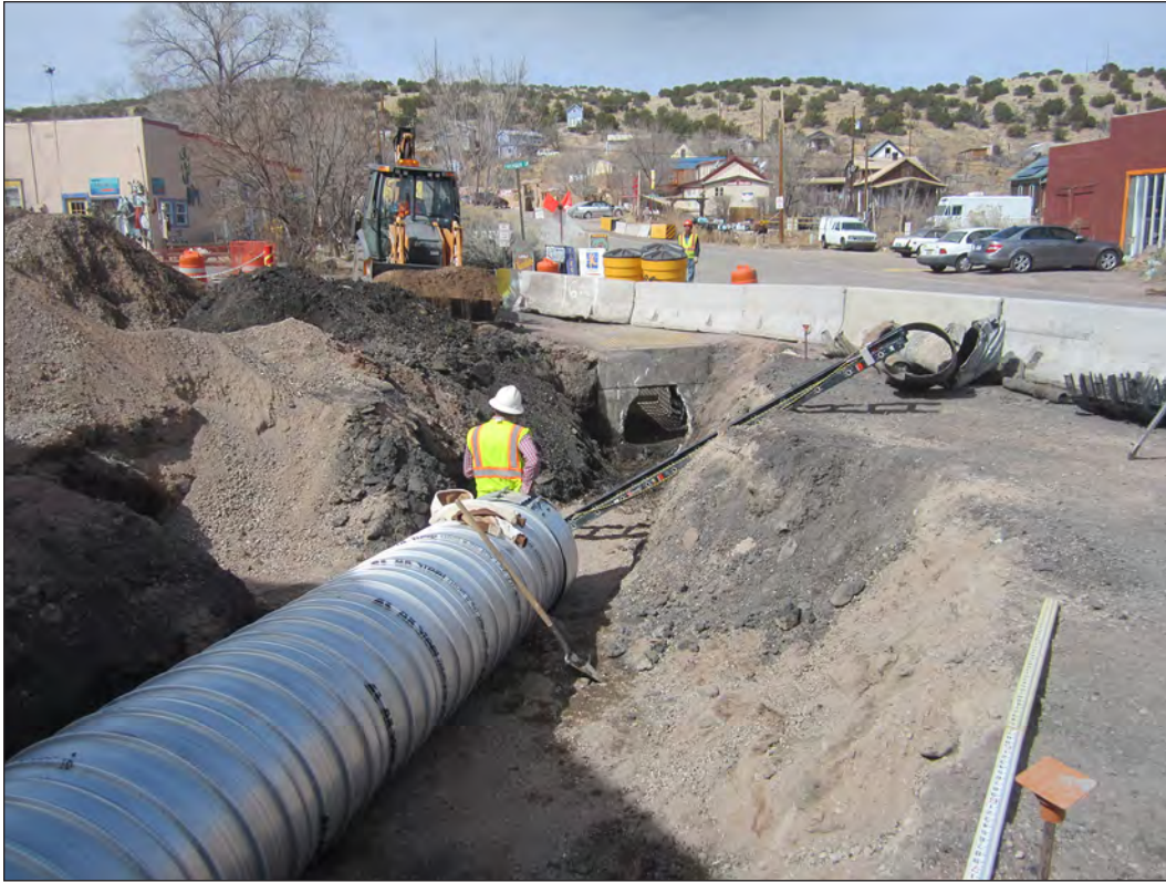
Figure 6.21. Widening the trench for slip liner, view southwest.
