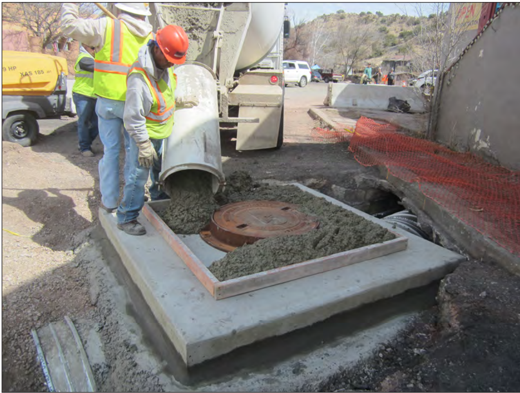
Figure 6.33. Concrete is poured into the manhole cover base, view north.
