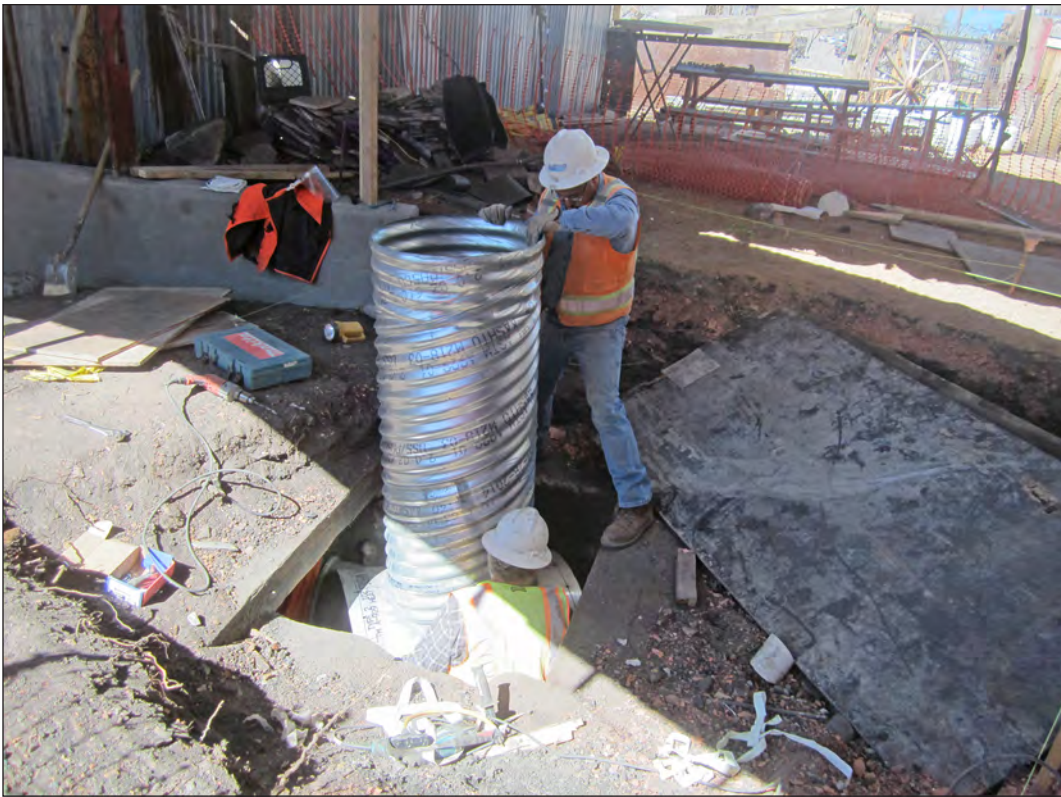
Figure 6.54. AUI crew attaches upright culvert to horizontal slip liner, view north.
