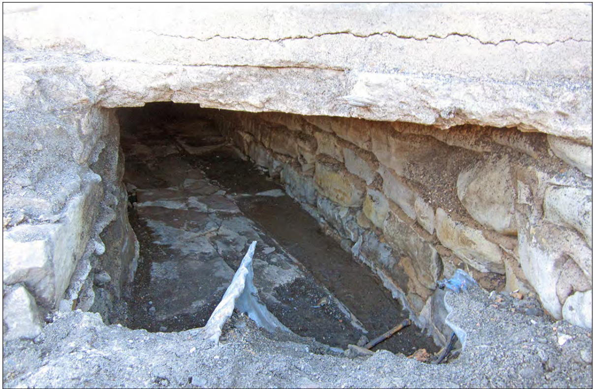
Figure 6.13. Feature 12, western end of cobble walls, view east.
