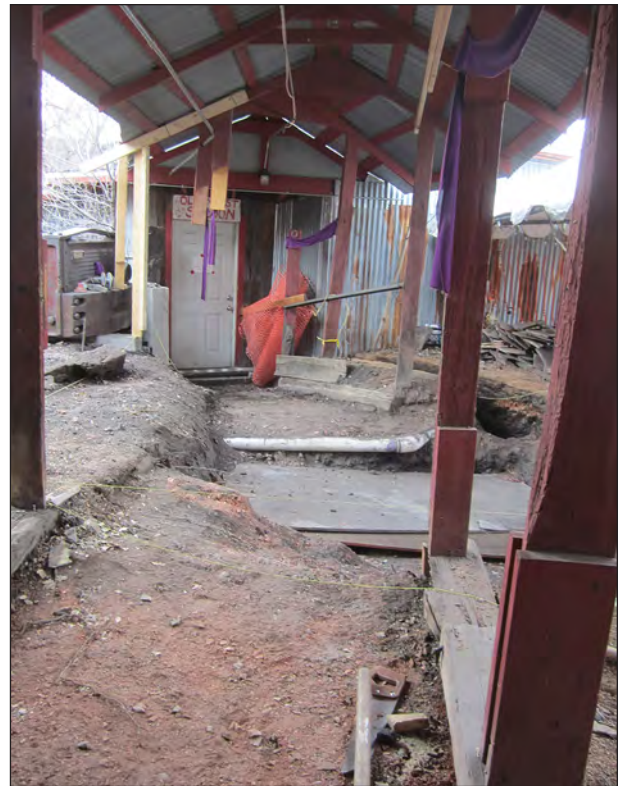
Figure 6.6. Walkway cleared of debris, view west.
