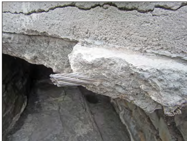
Figure 6.3. Feature 12, cement ceiling of box culvert, with cable reinforcement, view east.
