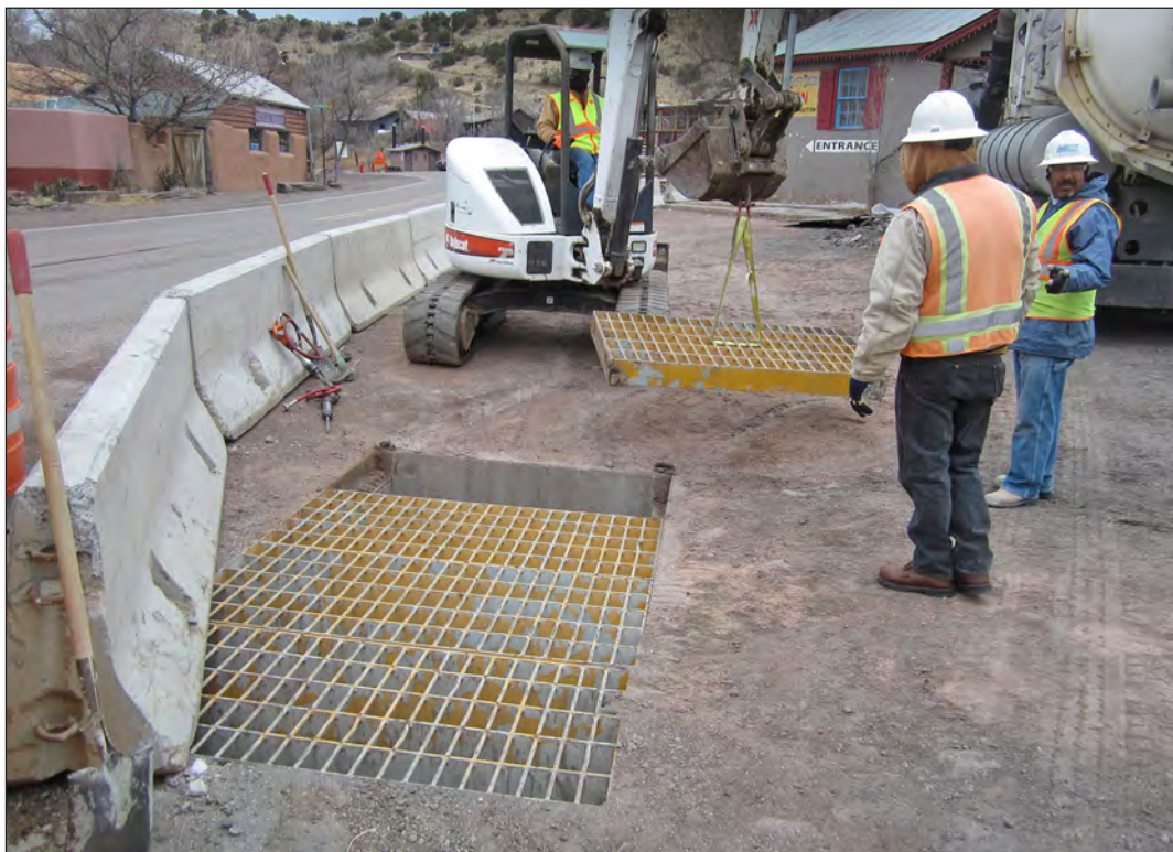
Figure 6.8. Removal of lower drop inlet cover near NM 14, view north.
