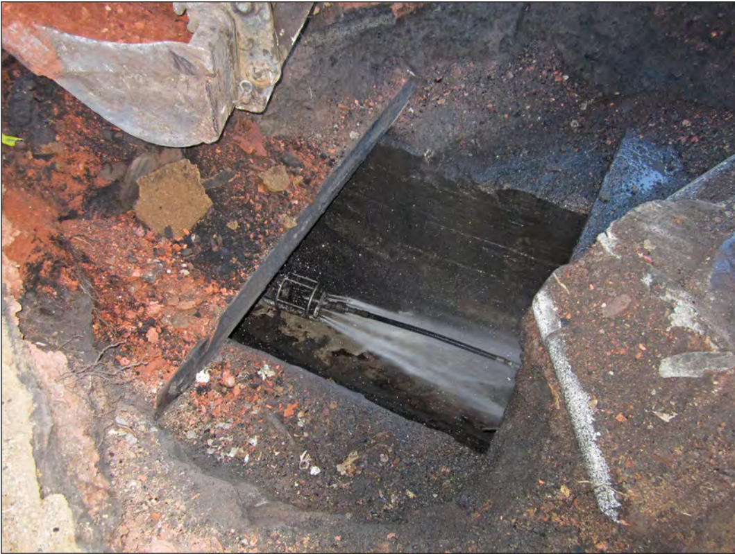
Figure 6.92. AUI crew jet-vacuums box culvert at the theatre walkway, view southeast.
