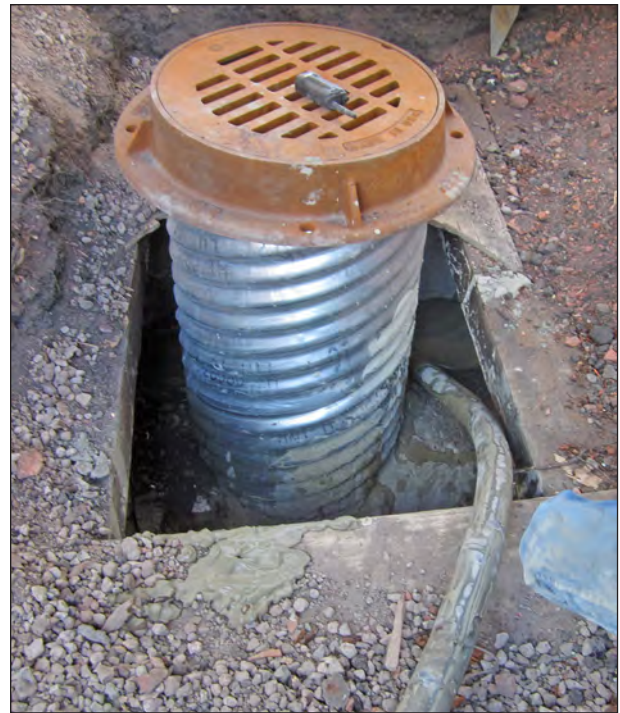
Figure 6.63. Grout is pumped into manhole in the theatre walkway, view north.
