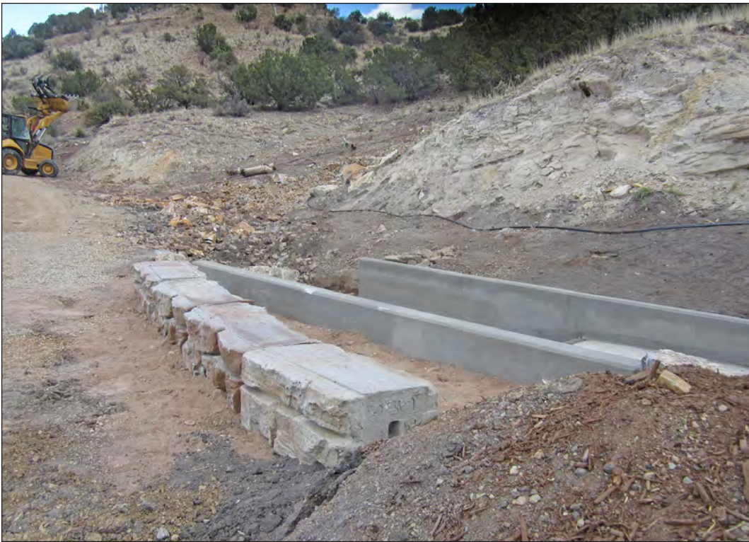
Figure 6.85. Jersey brick wall at upper drop inlet, view northeast.
