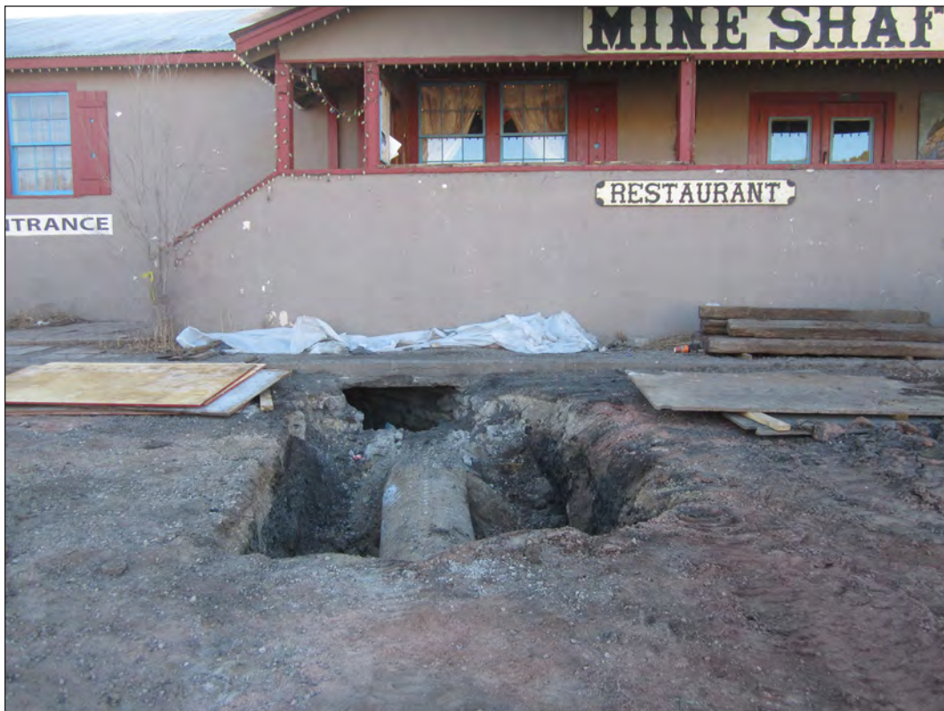
Figure 6.10. Old 60 cm (24 in) culvert at the western end of Feature 12, filled with sediment and gob, view east.
