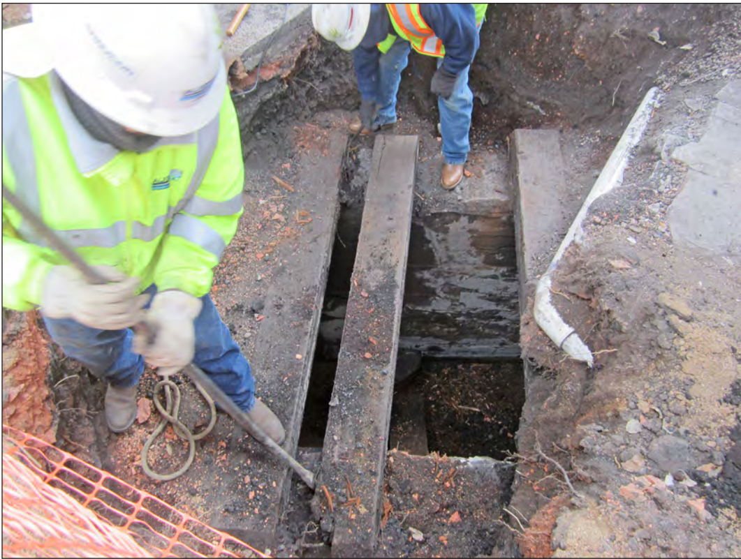
Figure 6.90. AUI crew removes railroad ties from box culvert ceiling, view north.
