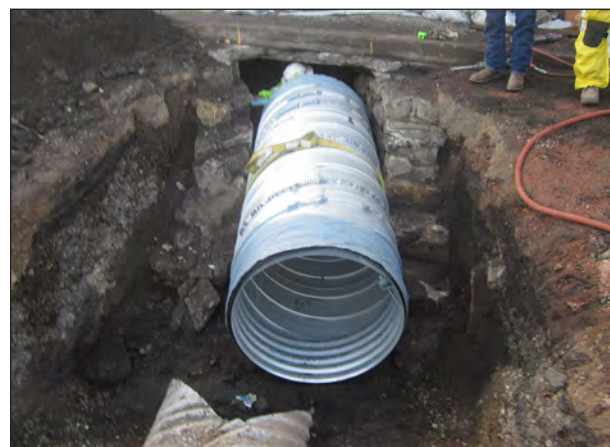
Figure 6.16. Slip lining installed between box inlet cobble walls, view east.
