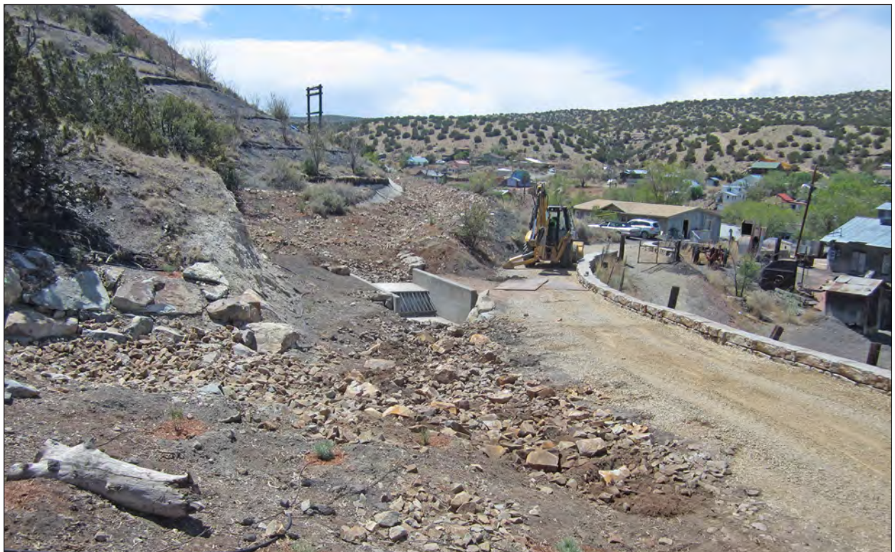
Figure 6.84. Landscaping work completed. Steel road plates have been removed, view south.
