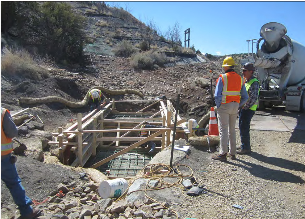
Figure 6.40. John Kretzmann, of AML, observes as cement is poured at the upper inlet of Feature 12, view southeast.
