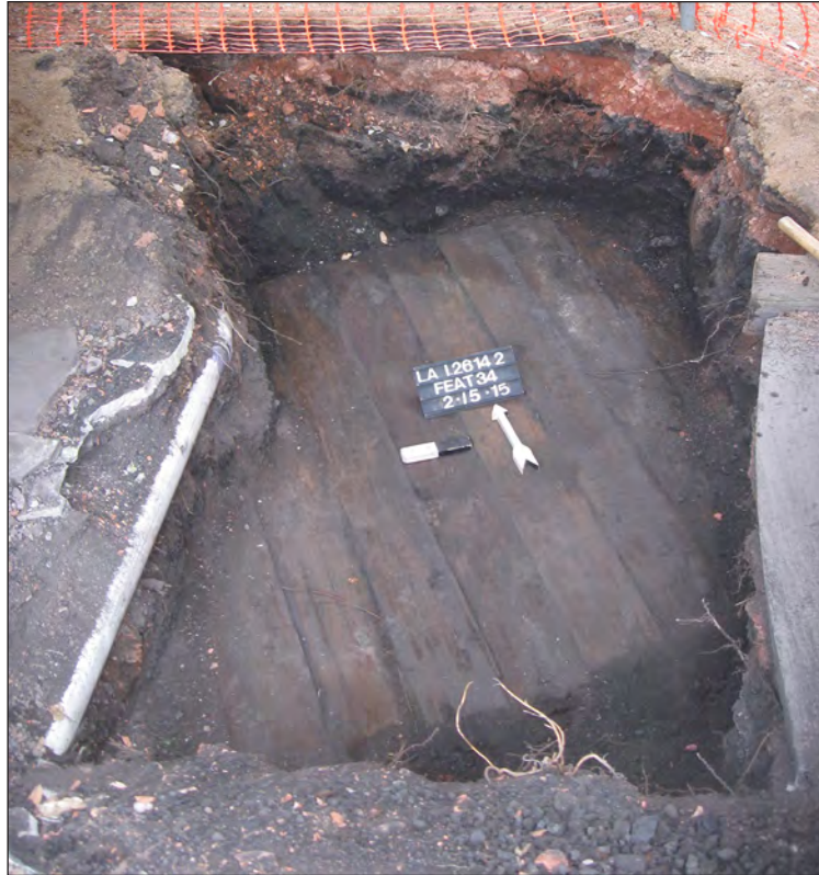
Figure 6.2. Feature 12, the railroad tie ceiling, on historic concrete box culvert. Feature 34 railroad ties in north face, view north.
