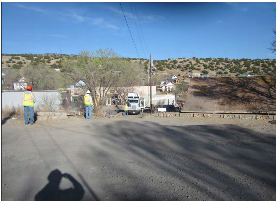
Figure 6.62. Con Deck powder truck arrives on site, view west.
