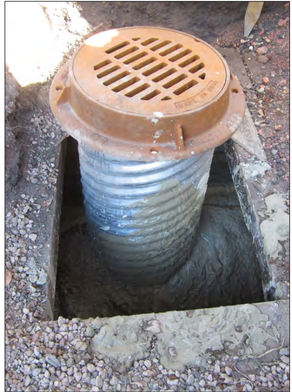
Figure 6.57. Grout-covered slip liner, view north.
