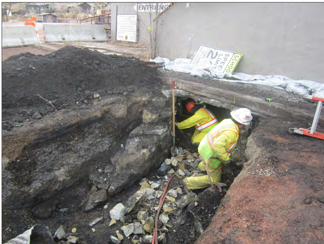
Figure 6.18. Demolition of cobblestone walls, view northeast.
