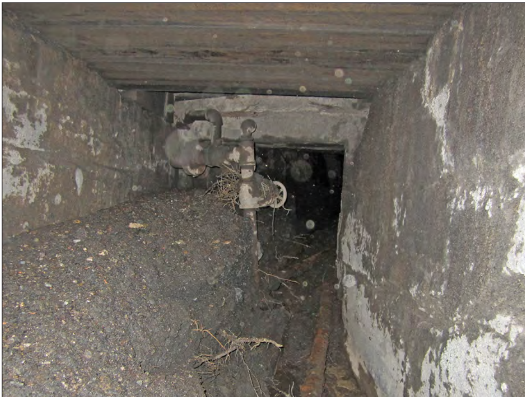
Figure 6.5. Box inlet interior with gob, sediment, and valves, view east.
