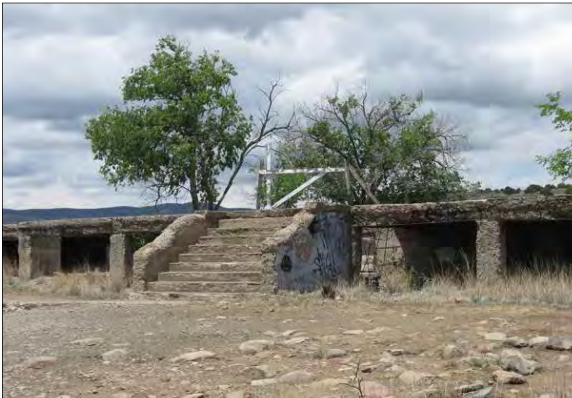
Figure 3.3. The foundation of the 1885 hospital, as seen today.
