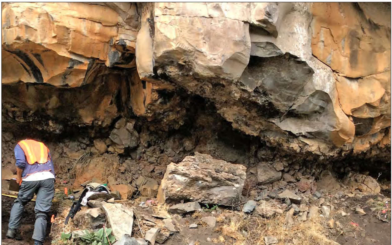
Figure 8.18. South Shelter, detail of light-colored rock showing possible recent impacts and spalling.
