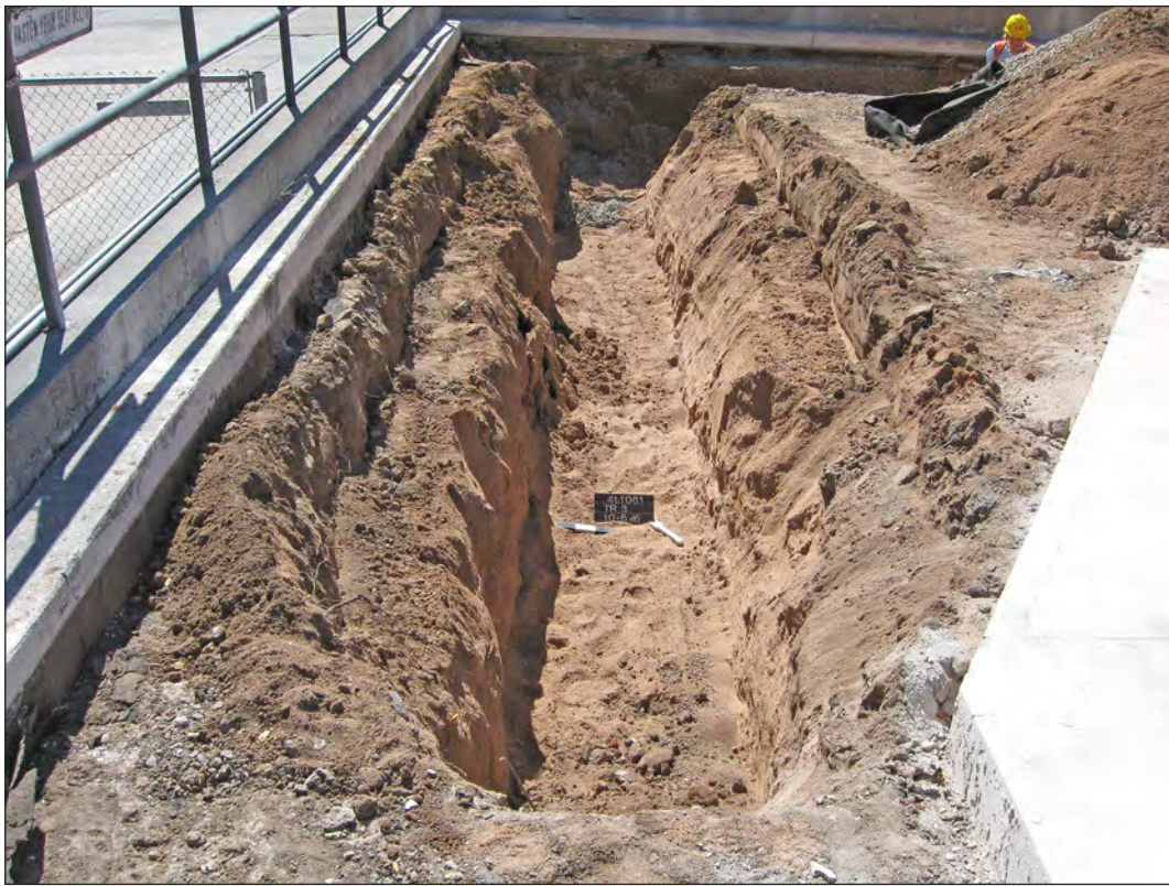
Figure 5.14. Backhoe Trench 3, overview, view south.
