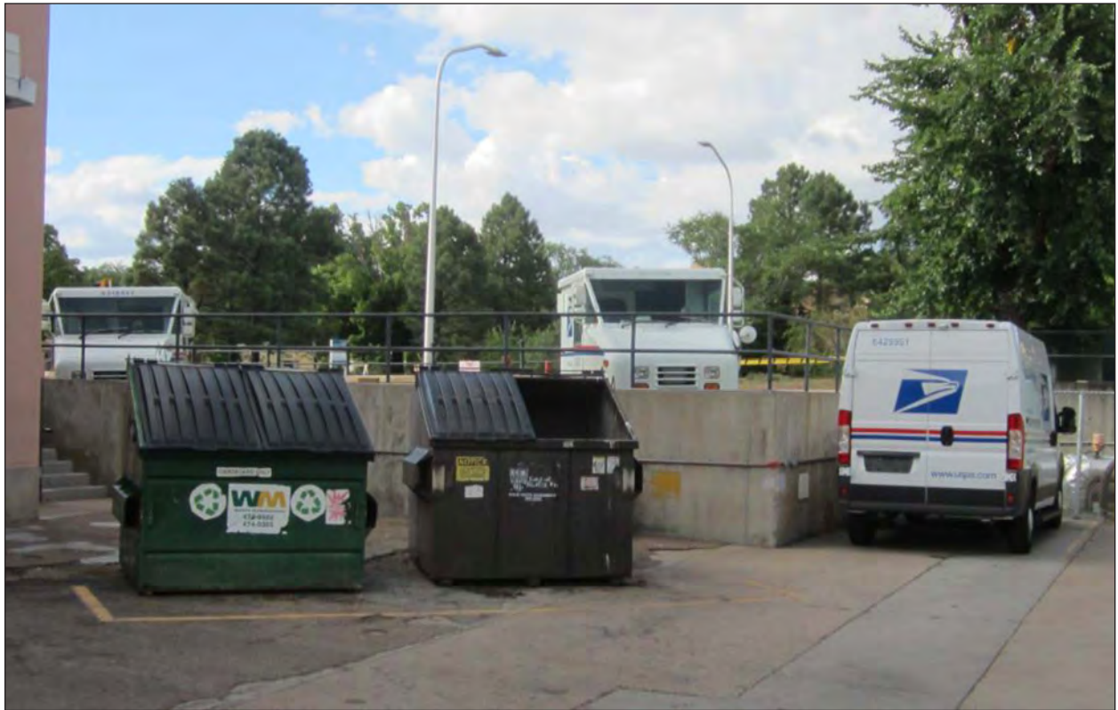
Figure 1.5. Loading dock at the existing post office, view northwest.
