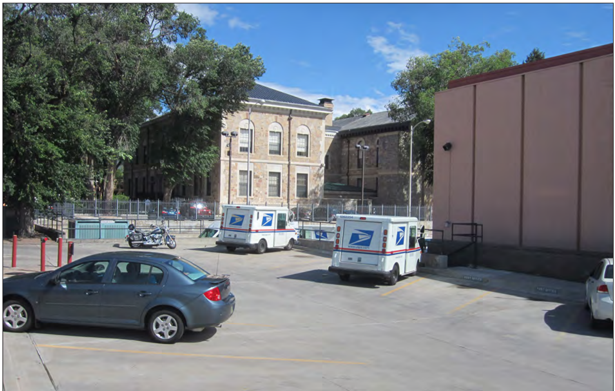
Figure 1.6. Federal Building, pre-excavation, view southwest.
