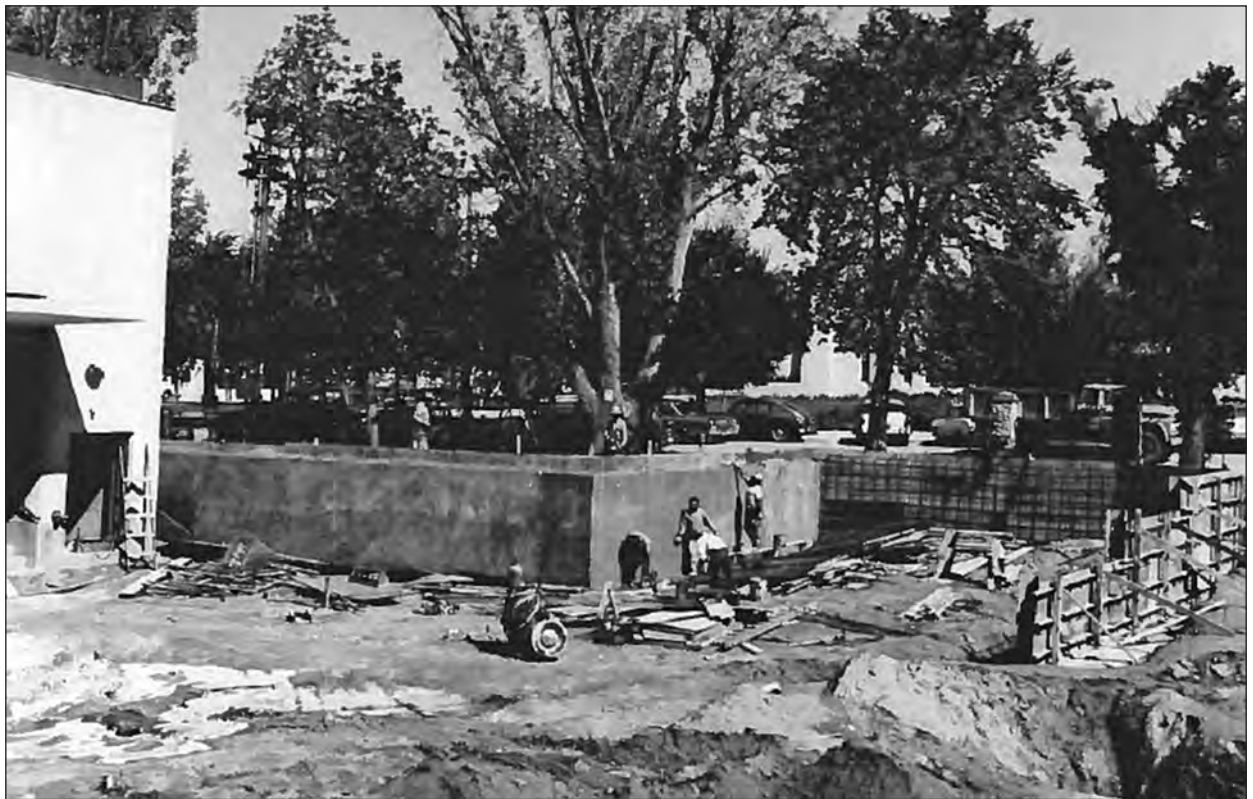
Figure 1.4. Federal Building construction project, 1962.
