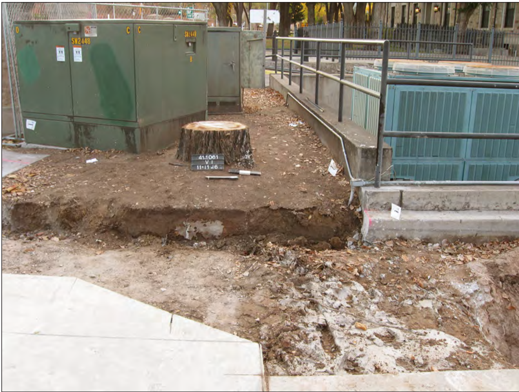
Figure 5.15. Backhoe Trench 3, north end, pre-excitation, view east.
