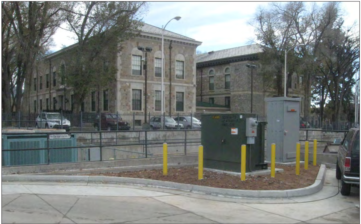
Figure 1.9. Newly installed vaults, view southeast.
