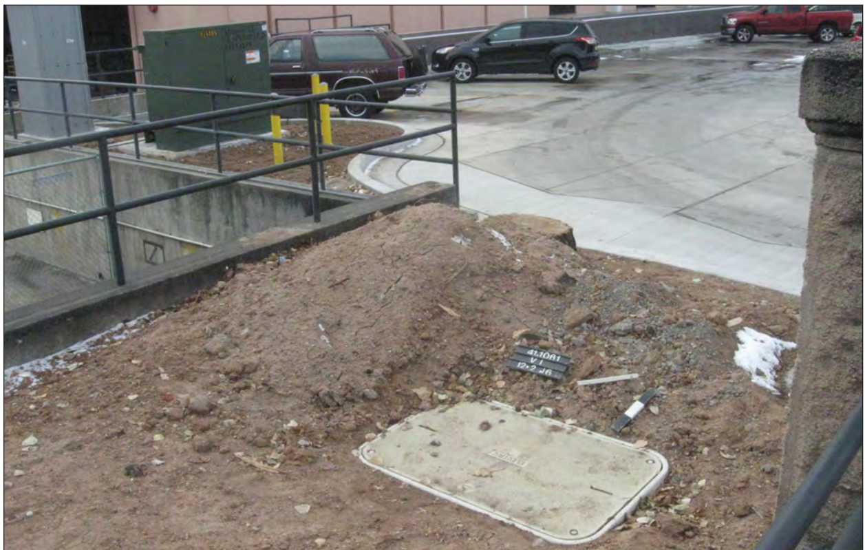
Figure 1.10. Vault replacement cover on north side of project area, view southwest.
