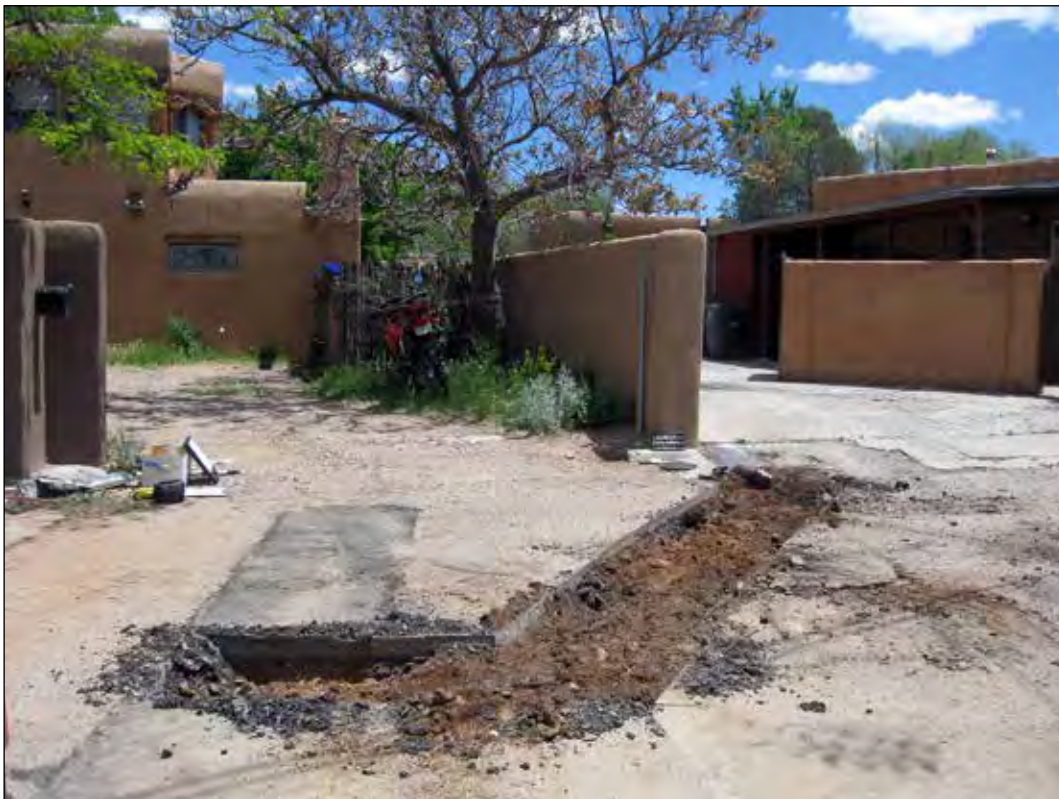
Figure 9.45. 249 Rael Road street trench, pre-excavation, view east.
