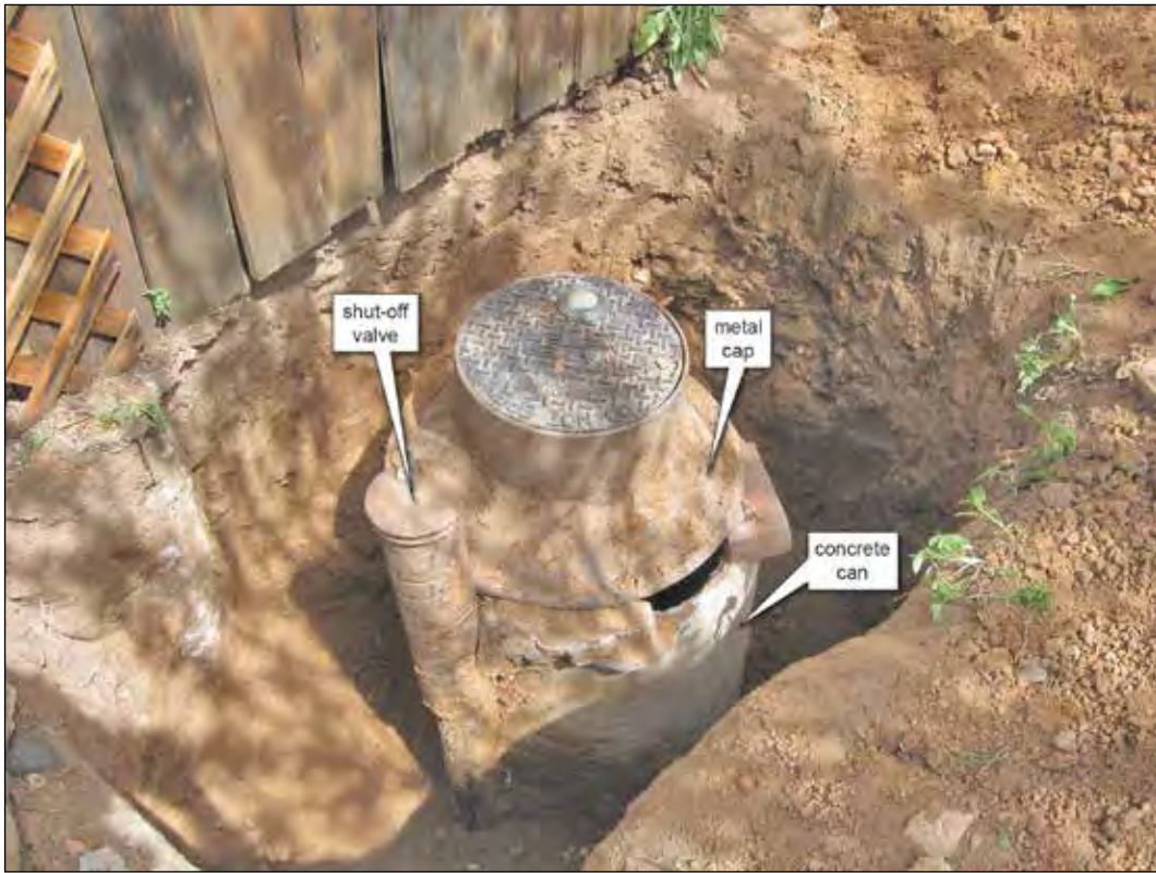
Figure 9.30. Old meter can at 631 Gomez Road, view northeast.
