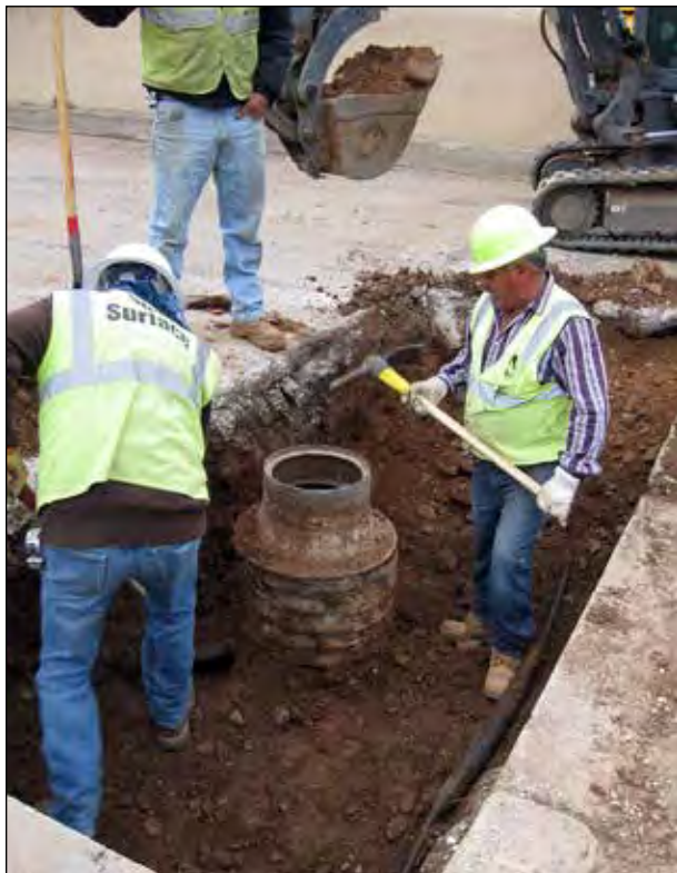
Figure 9.41. Old meter can at 625 Gomez road, view southwest.
