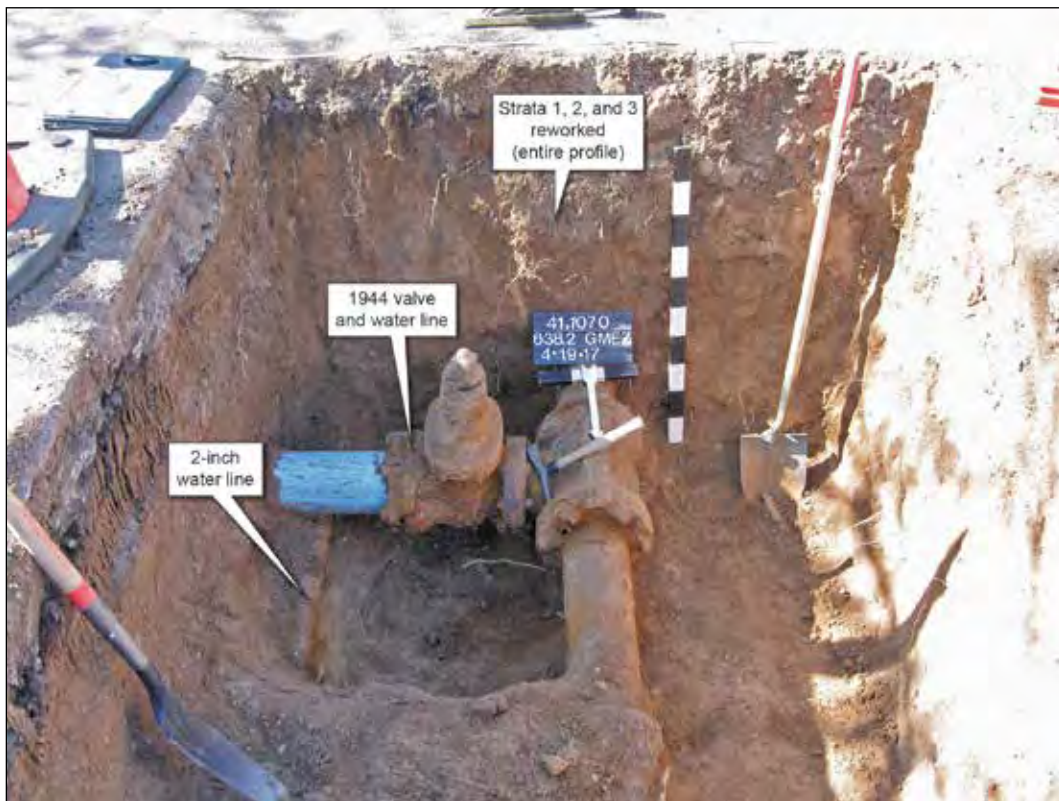
Figure 9.22. 638.2 Gomez Road valve replacement trench, view south.
