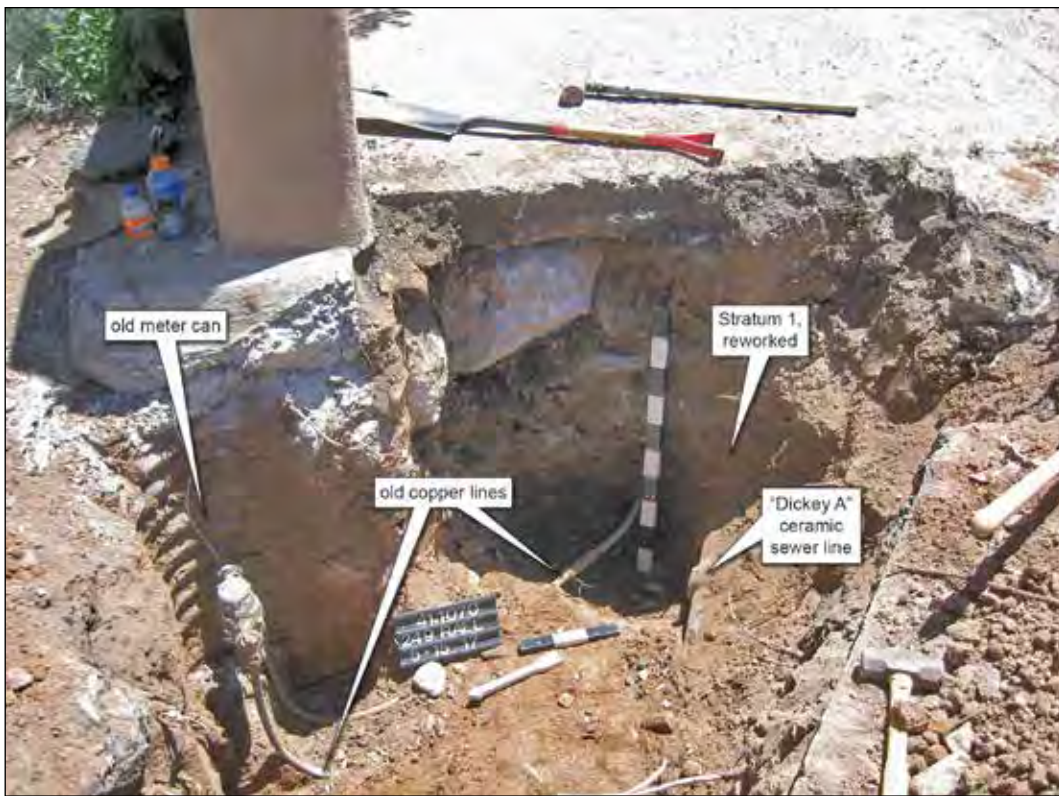
Figure 9.44. 249 Rael Road, view southeast.
