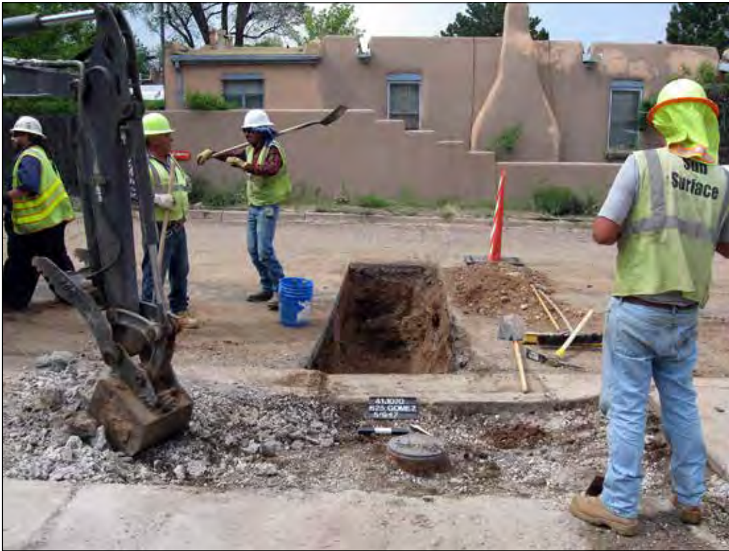
Figure 9.39. 625a–b Gomez Road, excavation in progress, view south.
