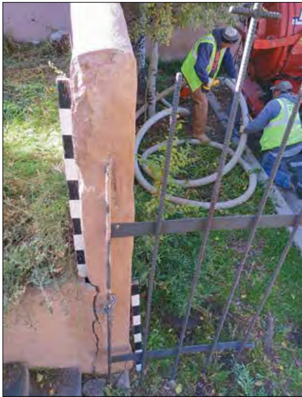
Figure 7.15. Retaining wall bisecting Hole 2, view south.
