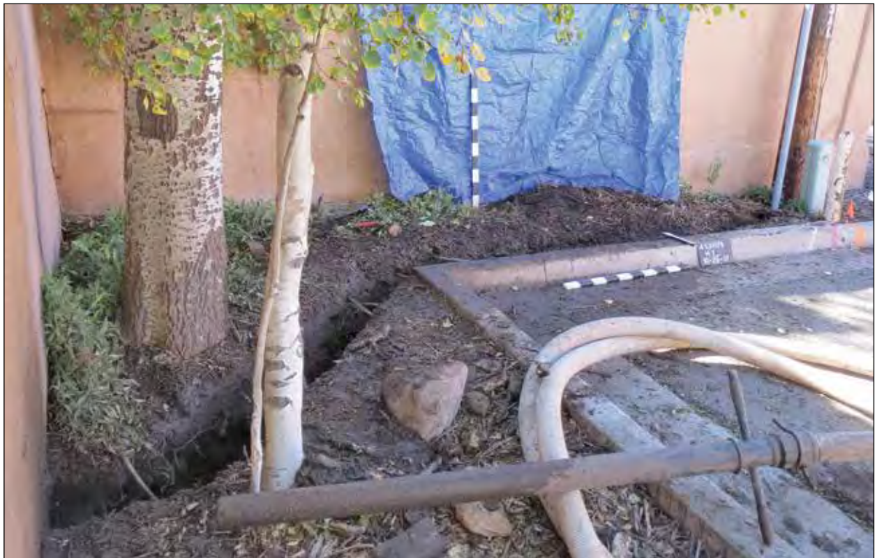
Figure 7.17. Hole 2, post-excavation, view south.
