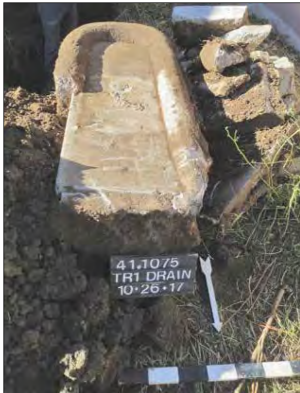
Figure 7.14. Concrete cañale drain slab at 107 Cienega St.
