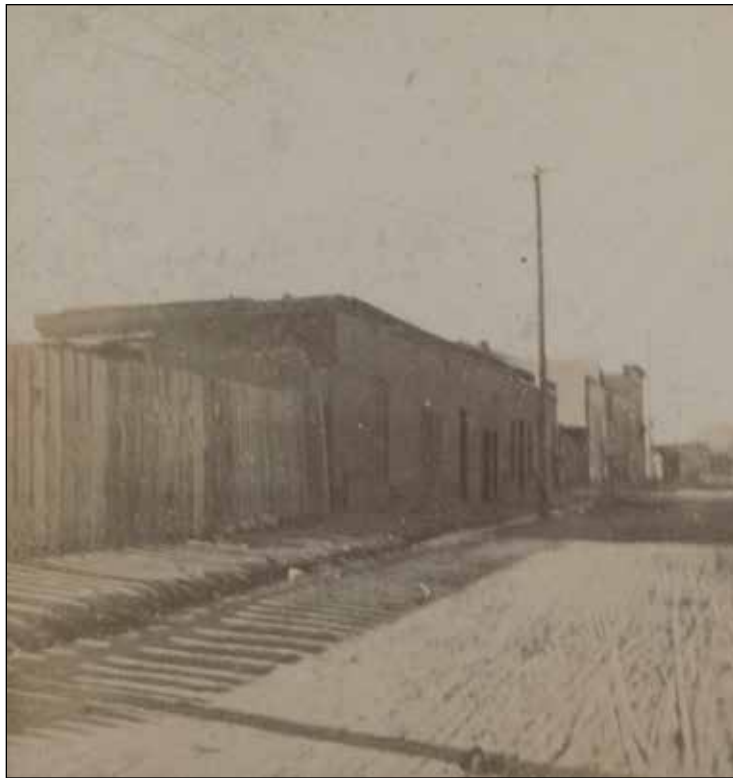
Figure 7.10. Water Street jail, circa 1895. Courtesy Palace of the Governors Photo Archives, Neg. No. 163219.
