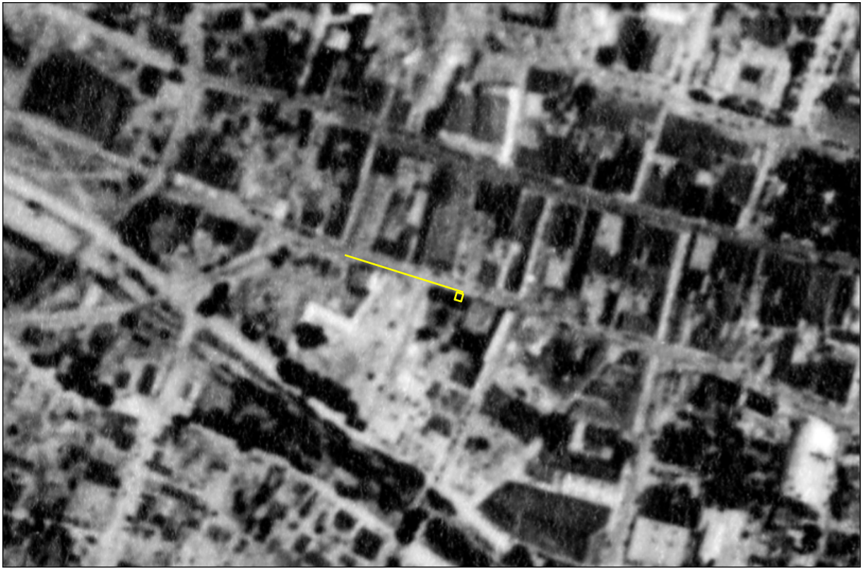
Figure 4.17. SCS aerial photograph (1936) with conduit route and vault overlay (in yellow).
