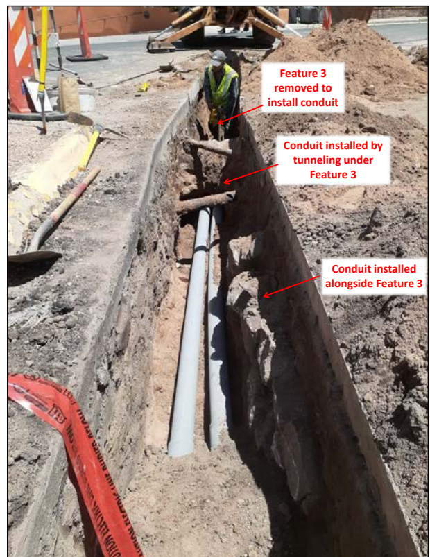
Figure 9.19. Feature 3, post-conduit installation 1890.
