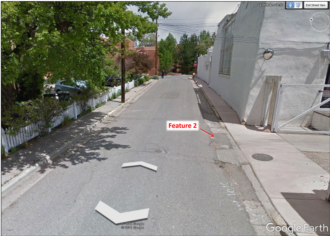
Figure 9.11. Location of Feature 2 in a patched section of the gutter on McKenzie Street, view east.
