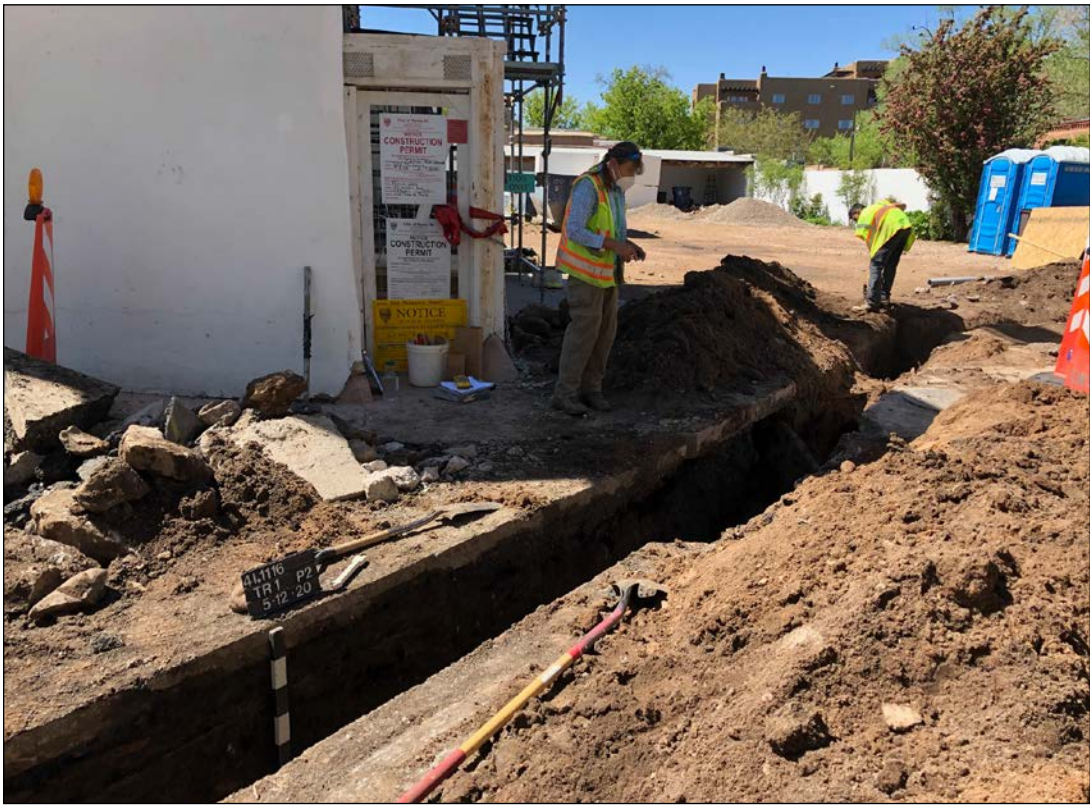
Figure 8.13. Trench 1, Profile 2 location shot, view south.
