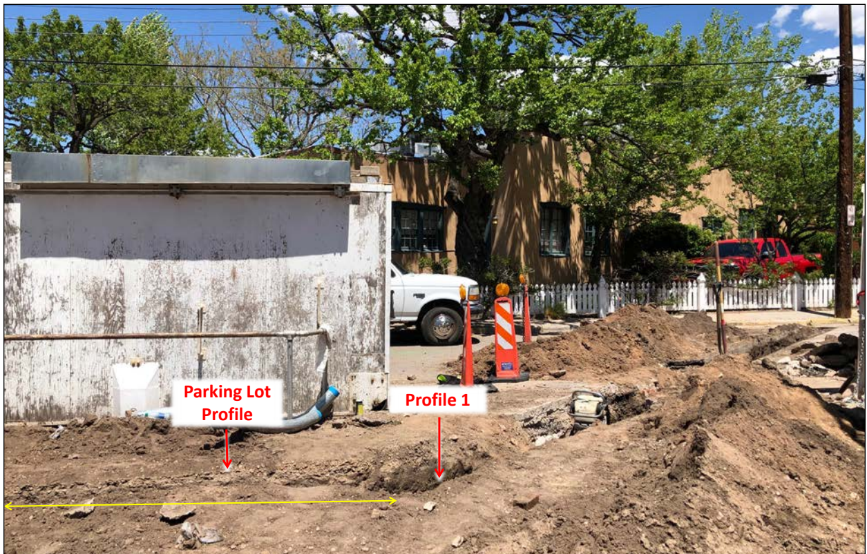
Figure 8.9. Trench 1, Profile 1 location shot, view north.
