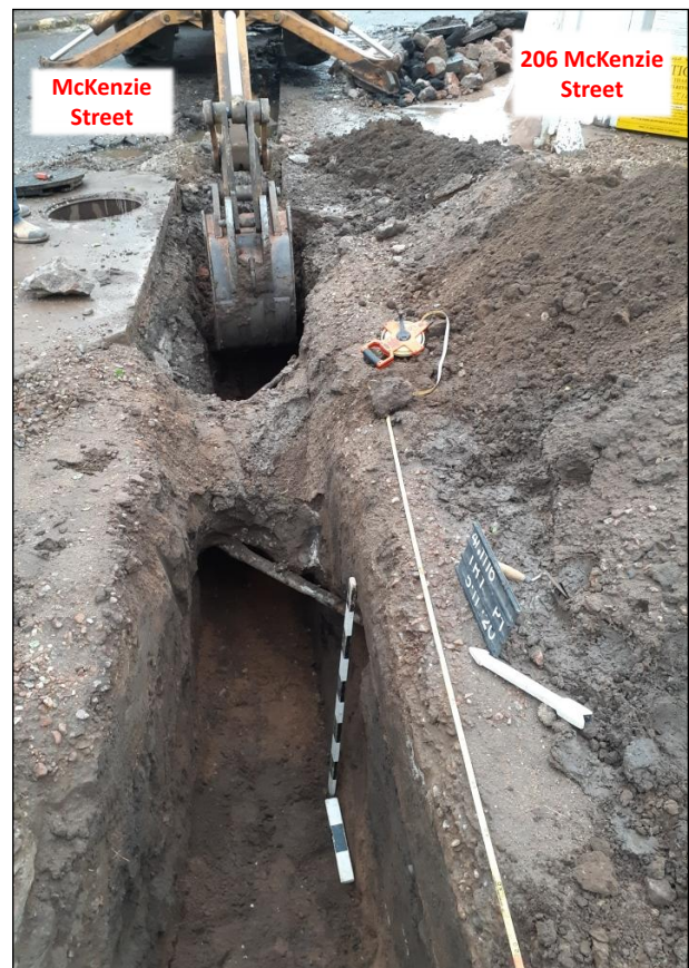
Figure 8.10. Trench 1, Profile 1 location with abandoned utility line, view east.
