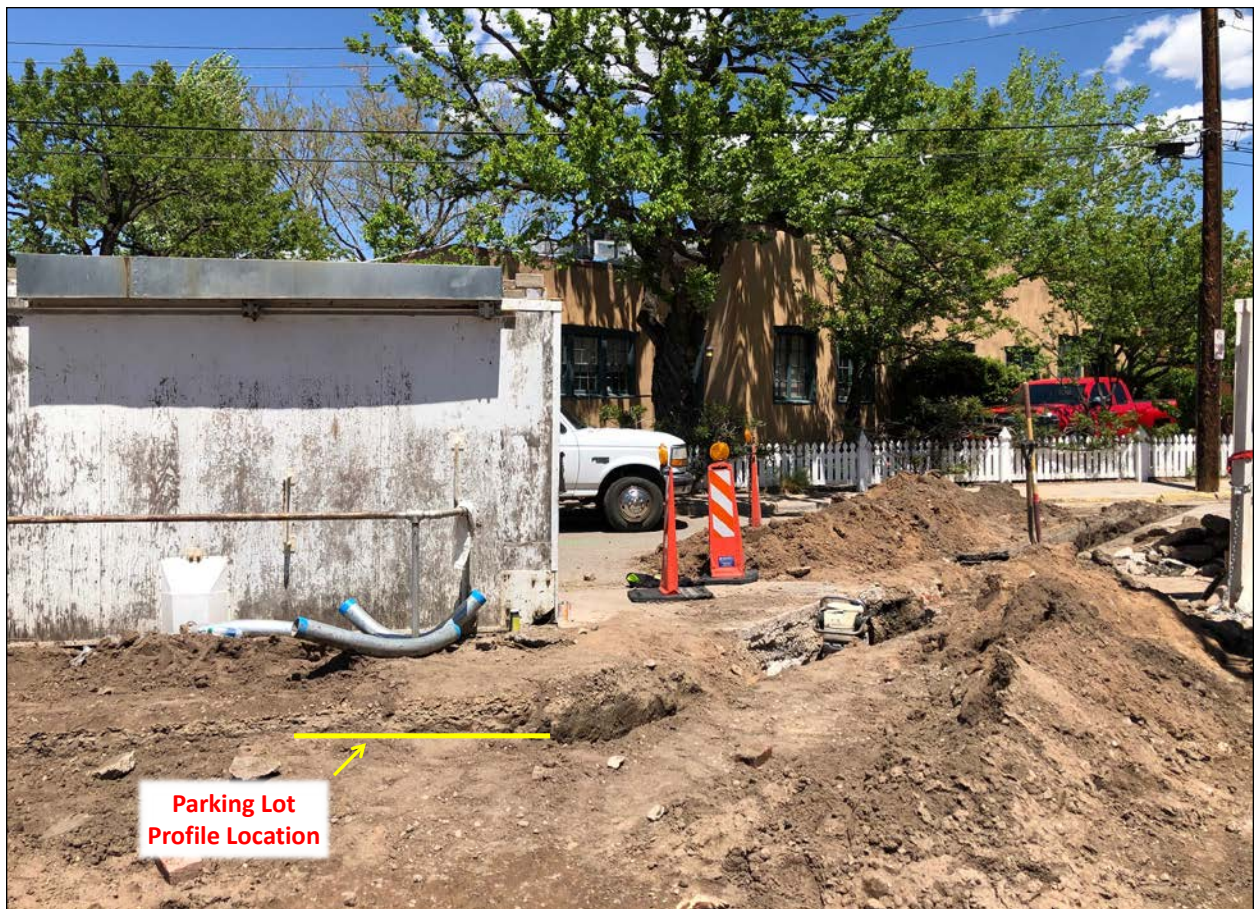
Figure 8.7. Trench 1, parking lot profile location, view north.
