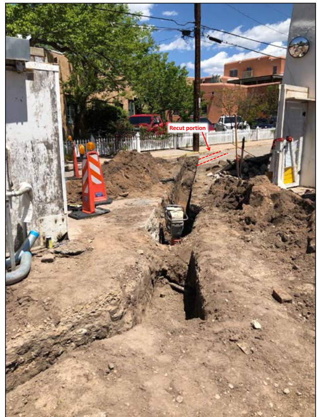
Figure 8.2. Trench 1, west end overview, view northeast.
