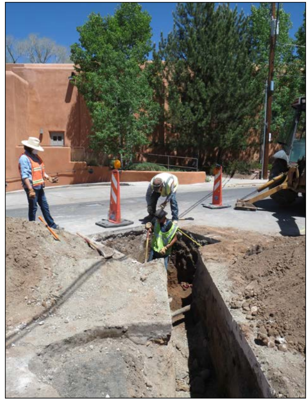
Figure 8.21. Vault location shot, view east.
