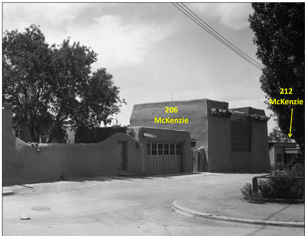
Figure 9.7. 206 McKenzie, view southwest, ca. 1936, prior to the construction of the pen tile structure south of the studio; 212 McKenzie appears on the far right, courtesy Palace of the Governors Photo Archives (NMHM/DCA), 069249.
