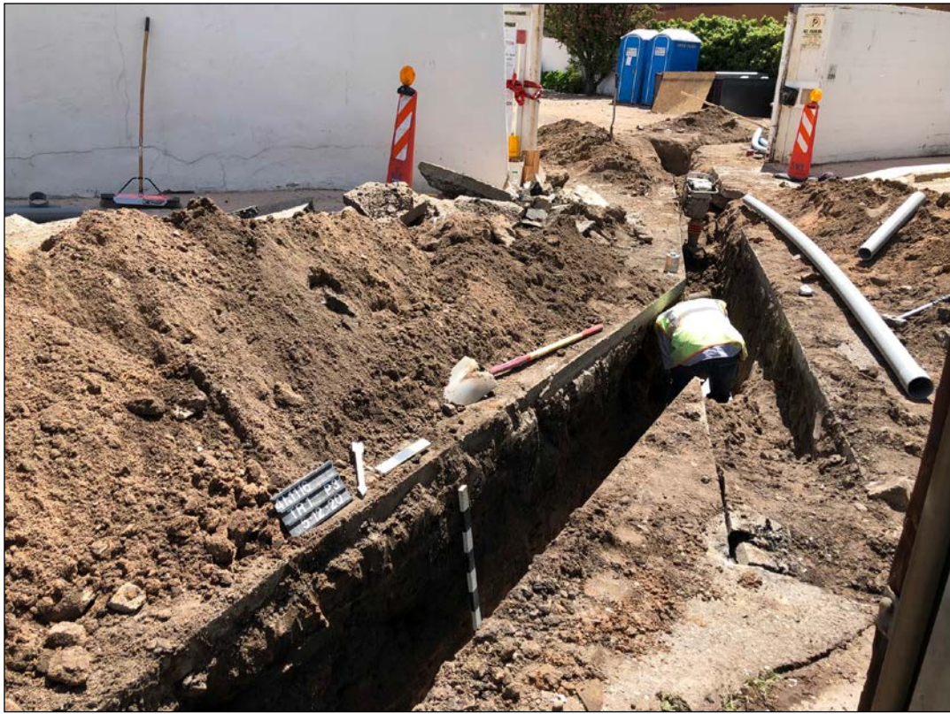
Figure 8.3. Trench 1, central area overview, view south.
