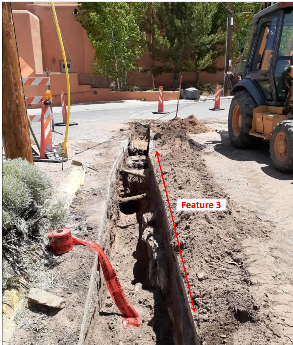
Figure 9.13. Feature 3 overview from west end, view east toward Griffin Street.
