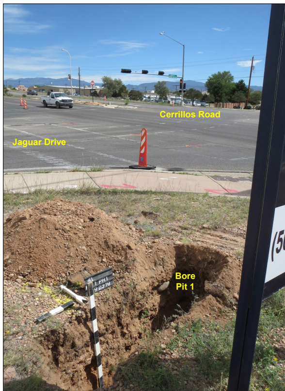
Figure 8.1. Bore Pit 1 location shot.
