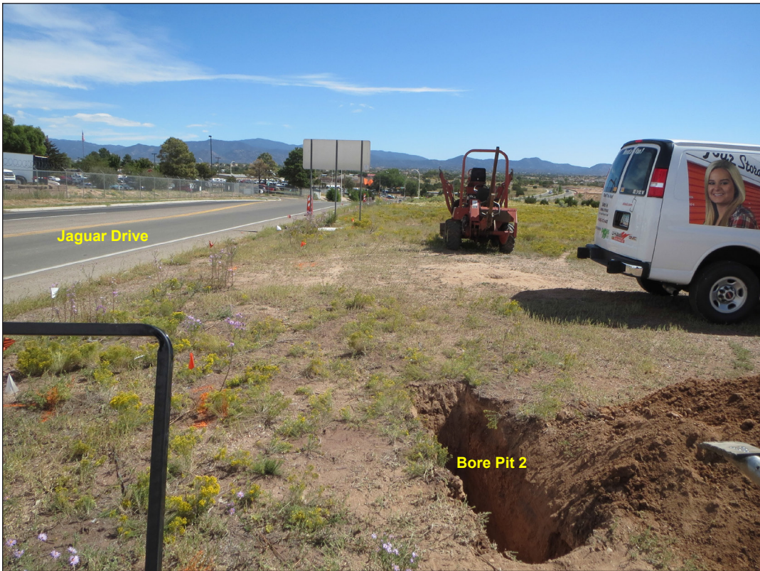
Figure 8.3. Bore Pit 2 location shot.
