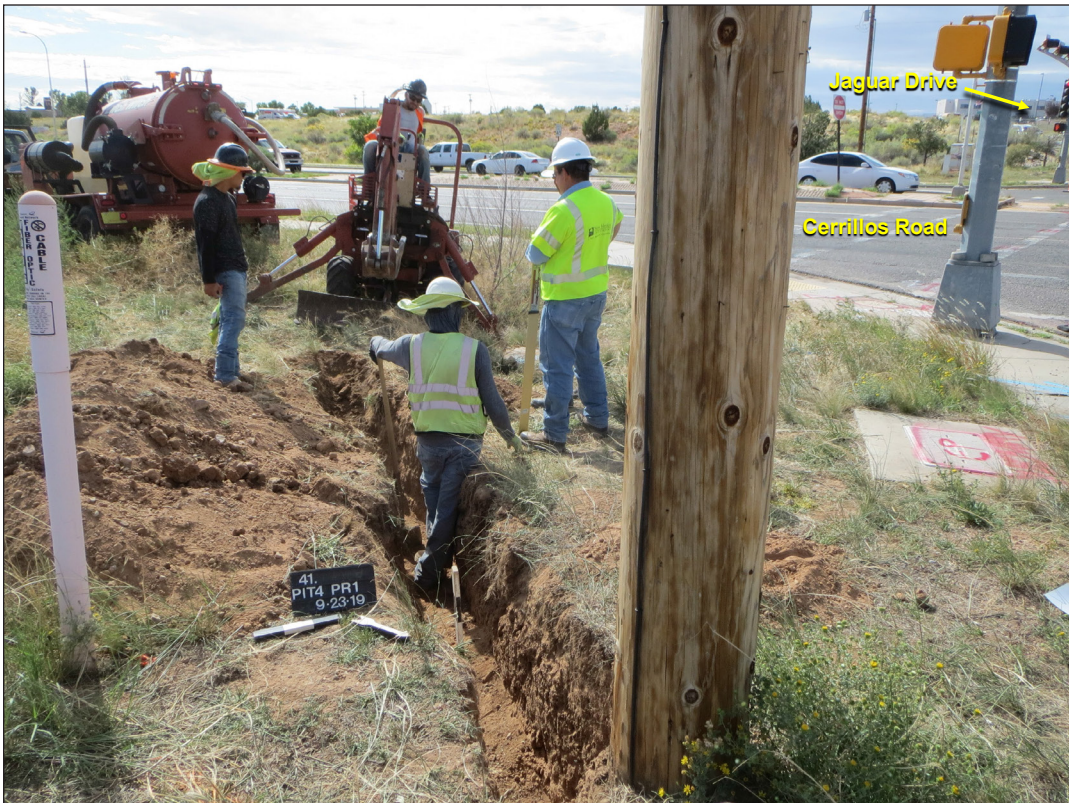
Figure 8.7. Bore Pit 4 location shot.
