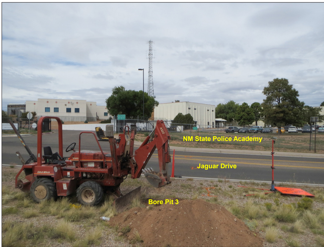
Figure 8.5. Bore Pit 3 location shot.
